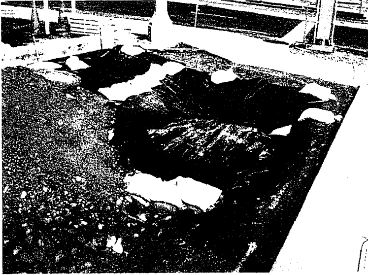
27. Inlet protection has improved at this location.
