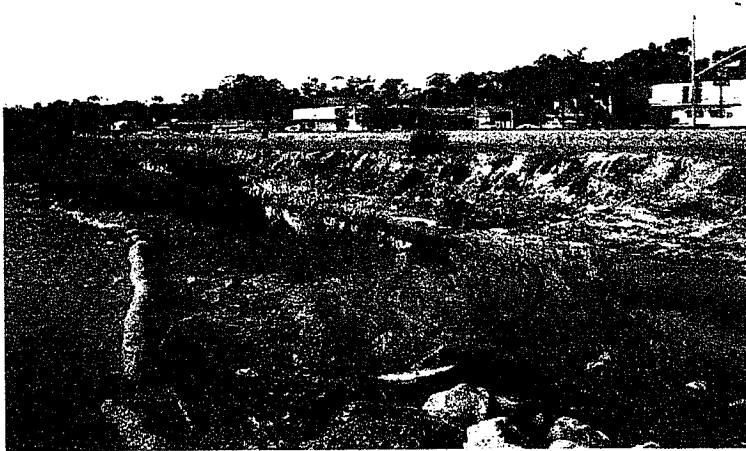
25. Fiber rolls still not trenched in. Previously, water has formed rills below untrenched fiber rolls.
