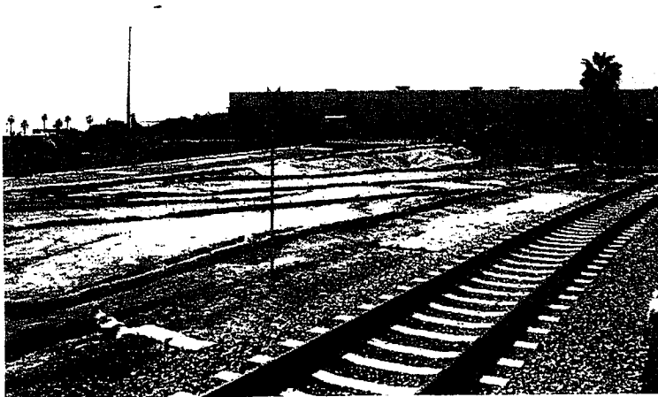
26. Improvements in this area include use of plastic sheeting, more fiber rolls and additional gravel bags.
