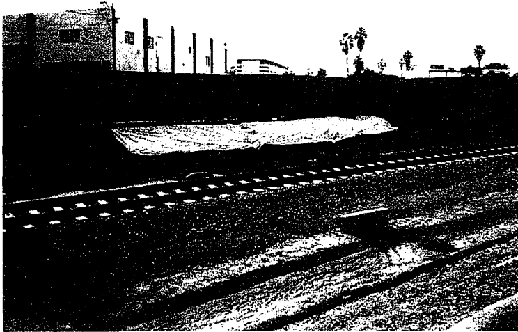
33. Slope is only partially covered with plastic.
