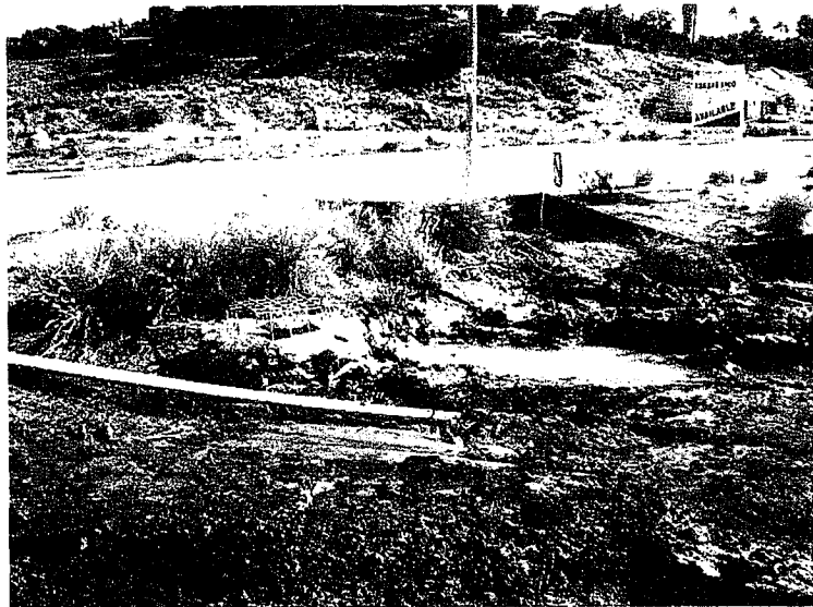
19. Storm drain inlet east of the inlet shown in Photo 16 appears to be adequately protected.
