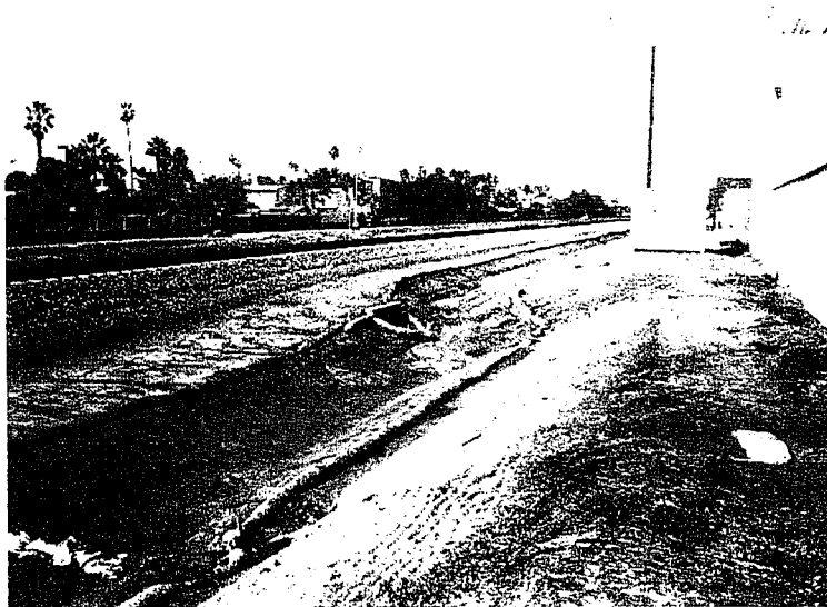
34. Partial stabilization on one side of the channel.
