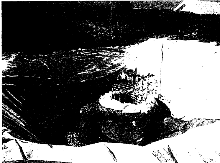
16. Area of the northwest storm drain inlet has been dug out to create a sediment detention basin.
