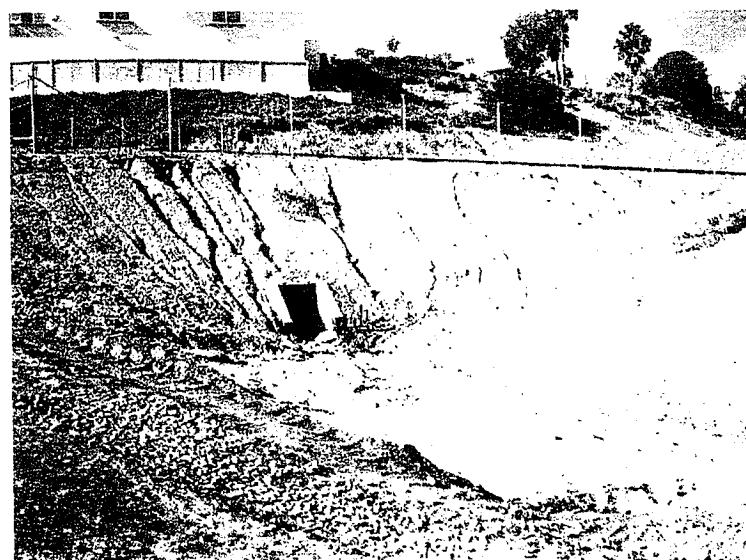
20. Outfall on south side of property leads to a channel that lacks erosion controls.
