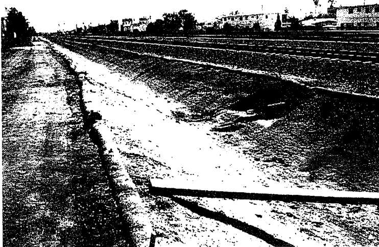
37. Only one side o this channel is stabilized. Channel leads to inlet shown in Photo 39.
