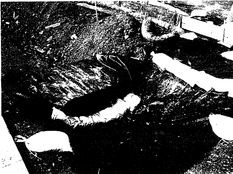
28. Another inlet with improved protection.
