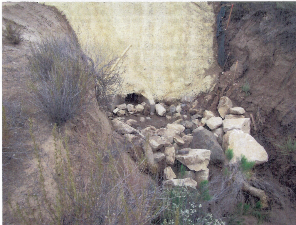
Photo 3: Storm water inlet structure installed at the base of the fill in Drainage 1.
