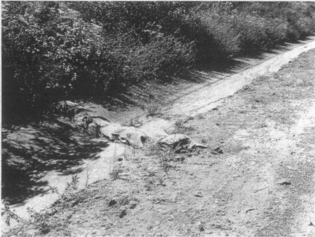
Photo 4 – Drainage channel on 2 nd Bench road from top deck.
