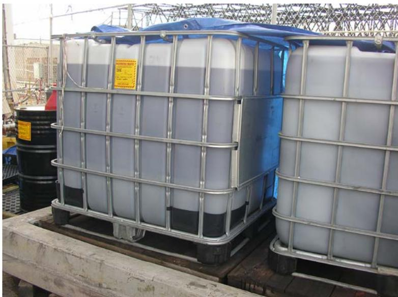
Photo 8. Cubes of oily bilge water have secondary containment. There was some water in the secondary containment.
