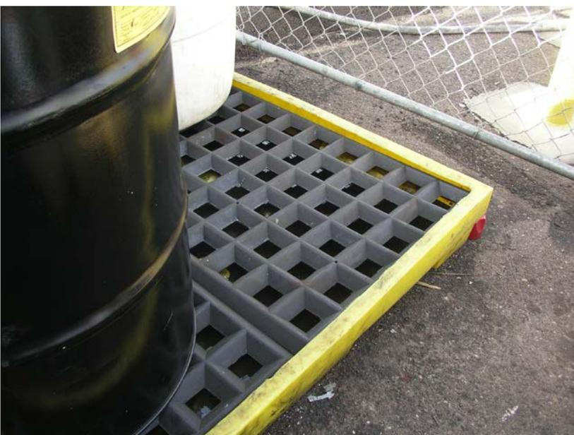
Photo 12. Water in secondary containment for drums in photo 11.
