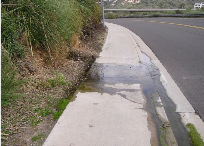
Figure 1. Perennial seepage from over-irrigation on mesa top. Flow enter the MS4 and discharge into Los Peñasquitos Lagoon, a 303(d) listed waterbody.
