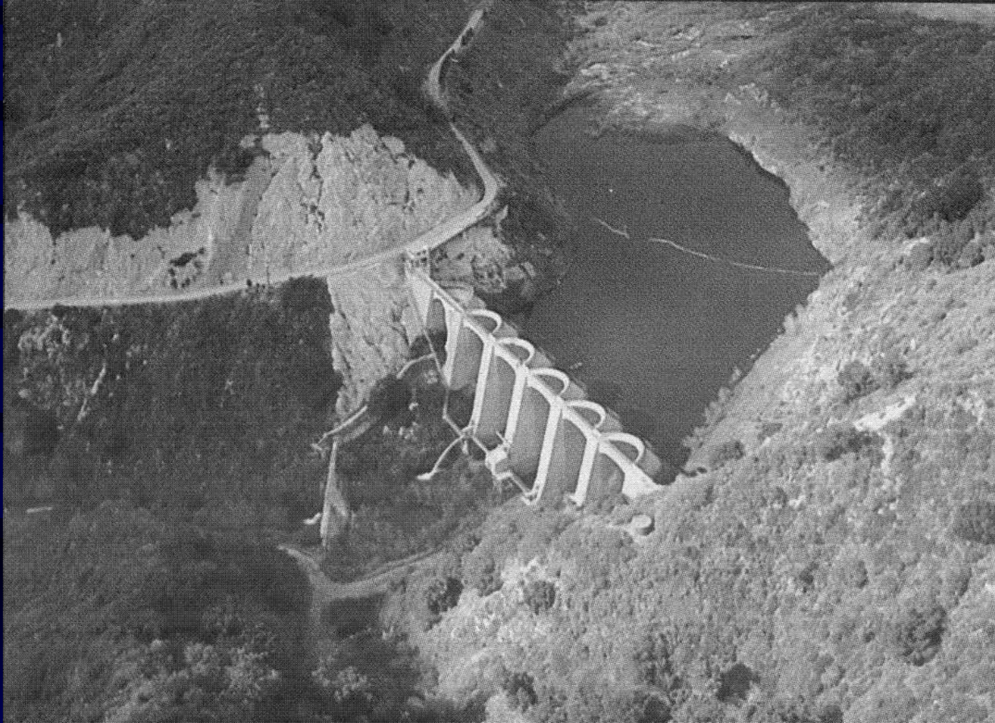
Big Dalton Dam and Reservoir
