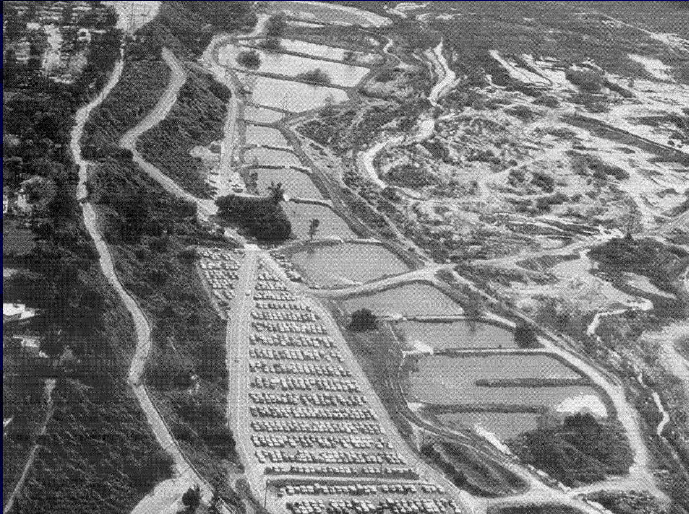
Arroyo Seco Spreading Grounds in Pasadena
