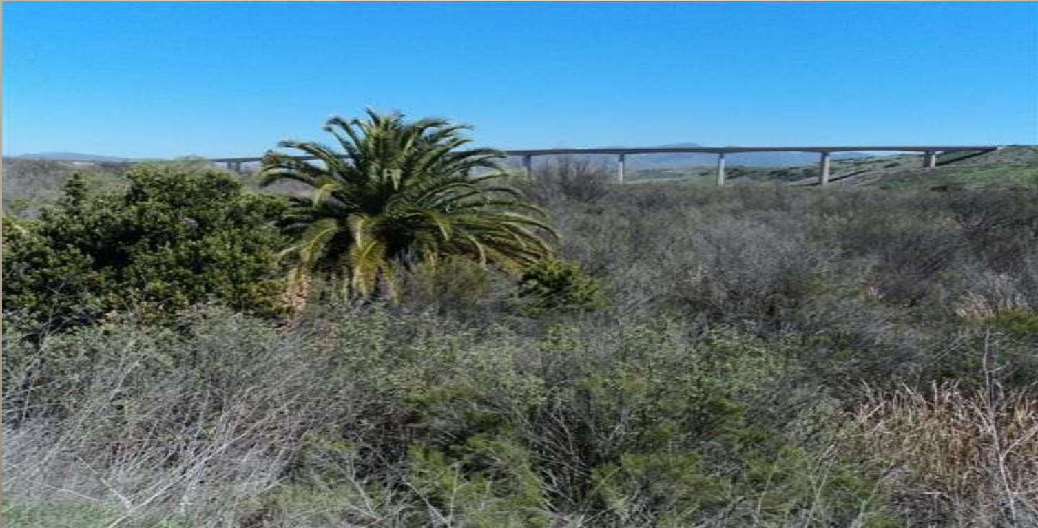
Otay River, Looking East (SR 125 bridge in background)
