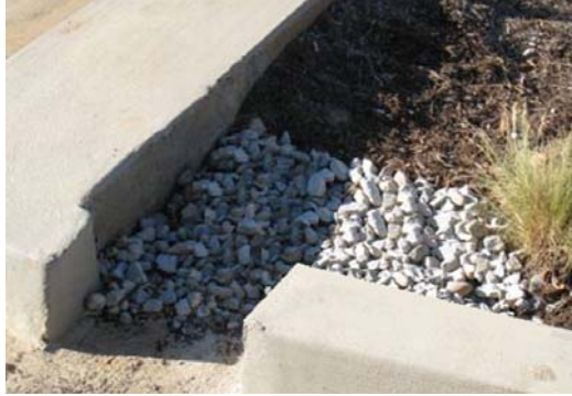
Figure 2: Curb Cut located in a Bioretention Facility
