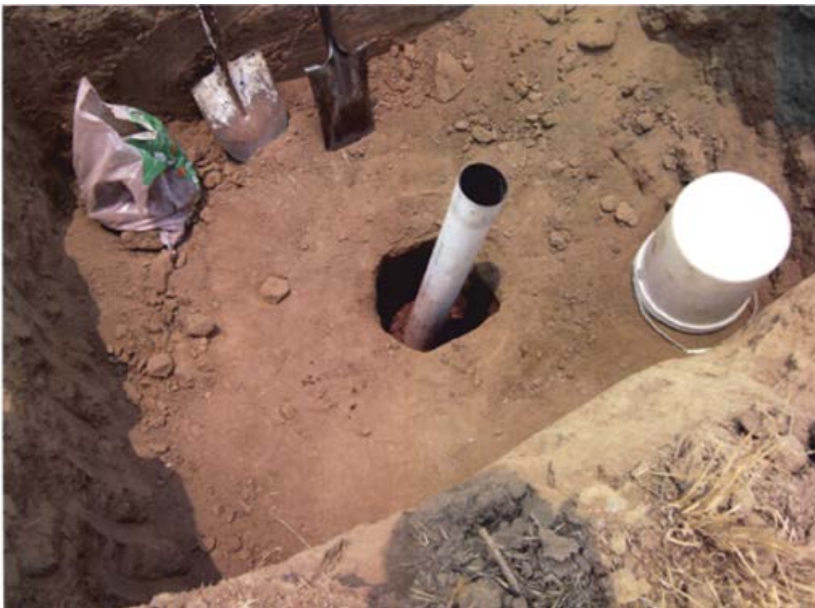
Photo 6 – Percolation Test Pit. Use of perforated PVC pipe is a variation.
