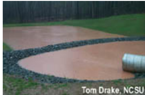
Figure 2: Forebay filled with storm water
