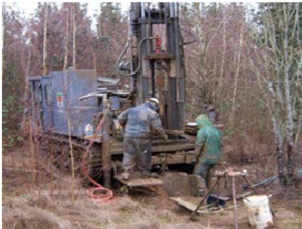
Photo 8- Auger Boring Rig
