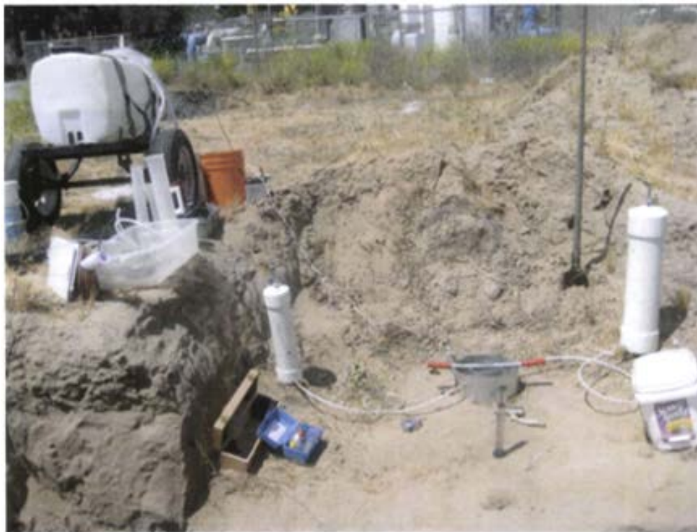
Photo 5 – Double Ring Infiltrometer Set-up for Test at Basin Surface Elevation (Photo courtesy of Turf-Tec International)
