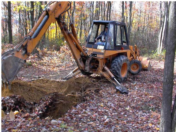
Photo 9 – Test Pit Excavation
