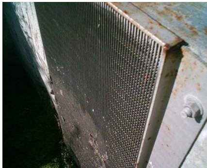
Trash rack with screen
