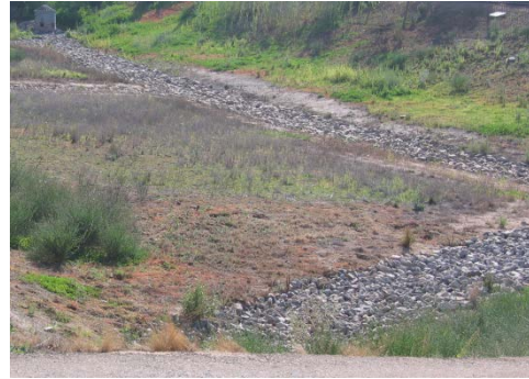
Figure 3: Gravel filled low-flow trench
