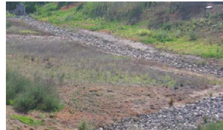
Gravel filled low-flow trench
