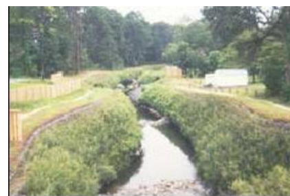
Figure 7.33 Established VRSS Structure (Sotir and Fischenich, 2003)
