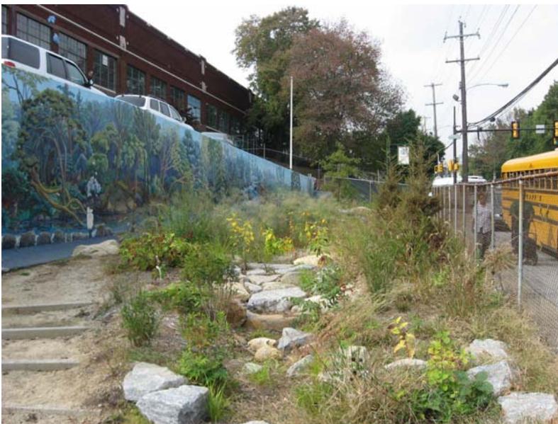
Philadelphia's new impervious-based fee encourages retrofits of large impervious sites, such as the Wissahickon Charter School (above), which now intercepts all parking lot runoff with rain gardens.
