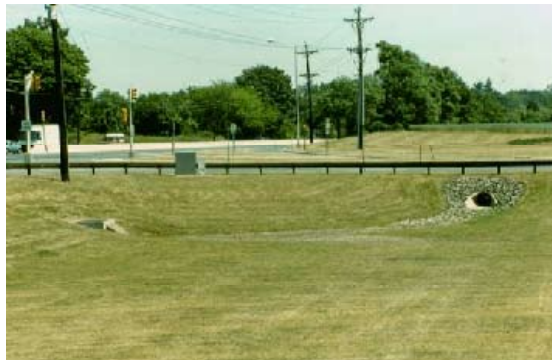
GOOD: Adequate bottom slope in dry detention basin creates intended dry bottom that can be regularly mowed and cleaned.
