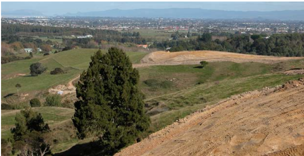
Minimal disturbance for earthmoving
