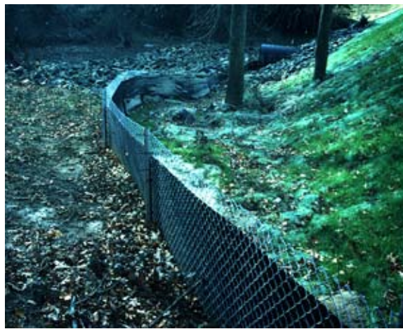
Super silt fence
