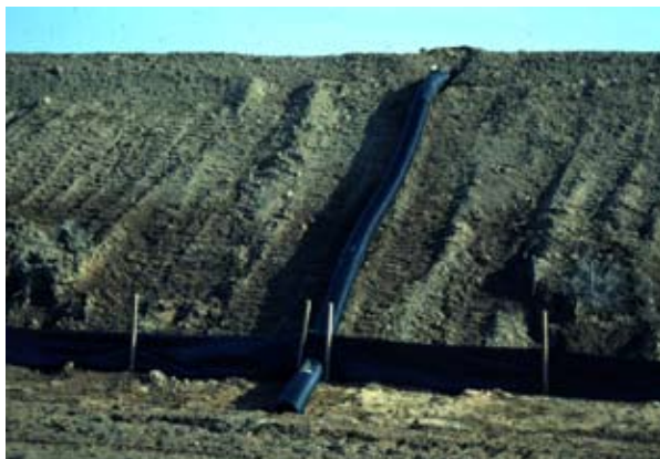
Examples of pipe and flume downdrains
