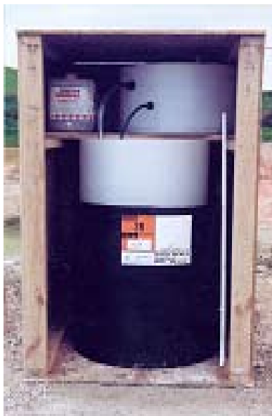
Example of an on-site chemical flocculation system
