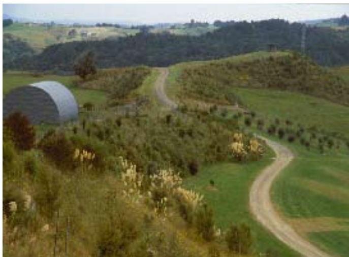
Revegetation of steep slopes and footprinting house locations in a development to minimize surface runoff
