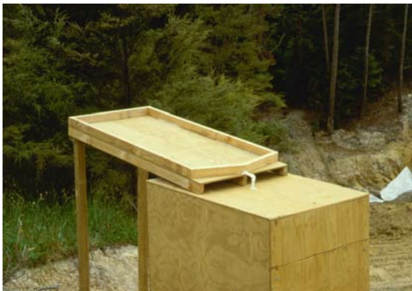
Roof area of flocculation unit
