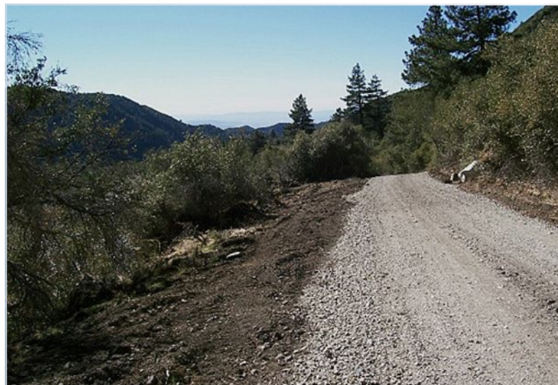
Figure 1. Low-volume road that has been newly graveled and out-sloped, San Bernardino County. Photo: Richard Harris.
