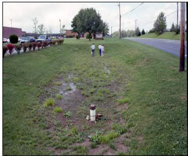
Figure 1: Surface Sand Filter
