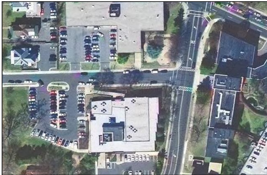
Figure 9: Retrofitting of non-residential rooftops is more complex.
