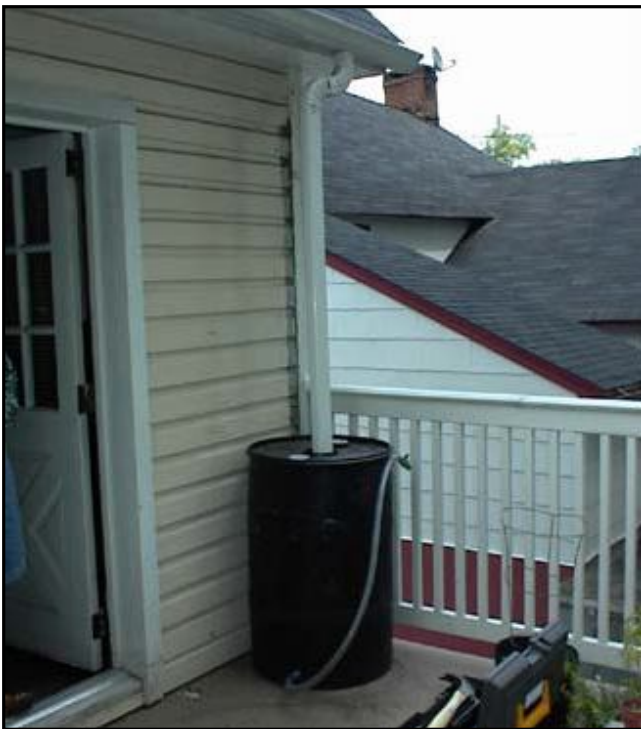
Figure 2: Rain barrel installed on a balcony due to space constraints on a small lot.
