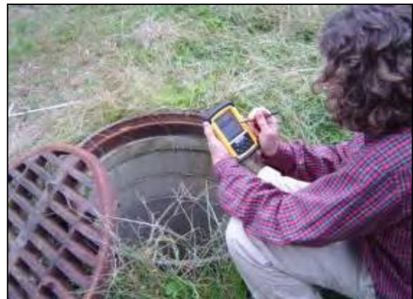
Figure 6: The invert elevation of the storm drain pipe underneath the lot is a critical design factors.
