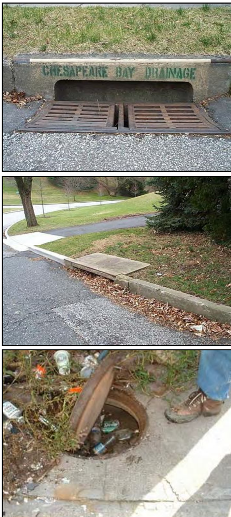
Figure 7: Crews check storm drains, grate inlets or manholes to determine depth of enclosed storm drainage.
