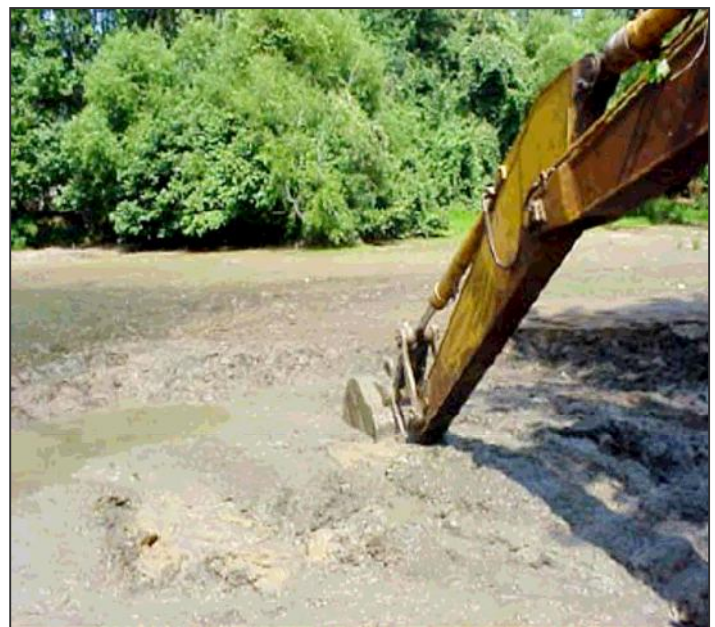
Figure 11: Dewatering is needed to excavate bottom sediments.
