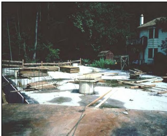
Figure 3: Large underground sand filter under construction to treat runoff near a drinking water intake.
