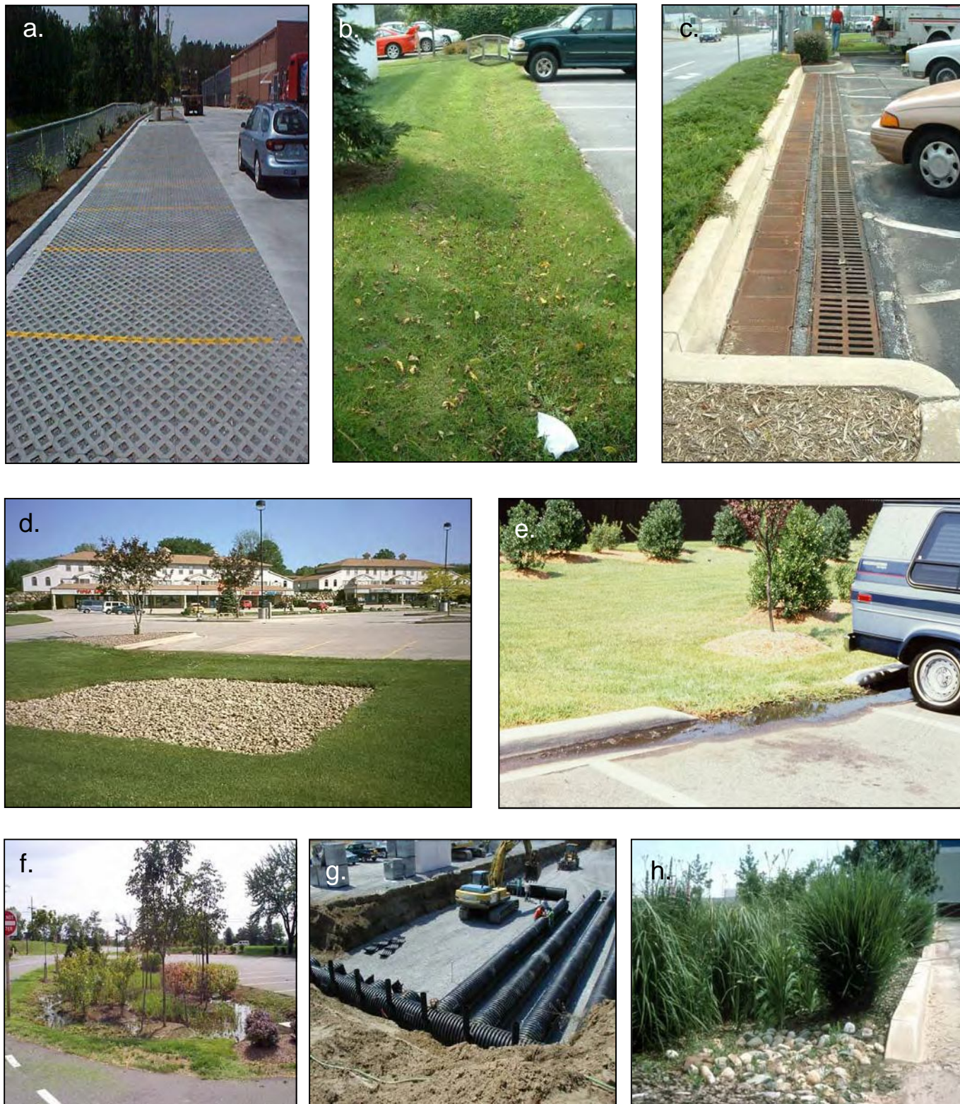
Figure 2: Examples of retrofits employed at small parking lots: permeable pavers (a); dry swale (b); perimeter sand filter (c); grass filter//infiltration trench (d); filter strip (e); internal bioretention (f); underground infiltration (g) and island bioretention (h).
