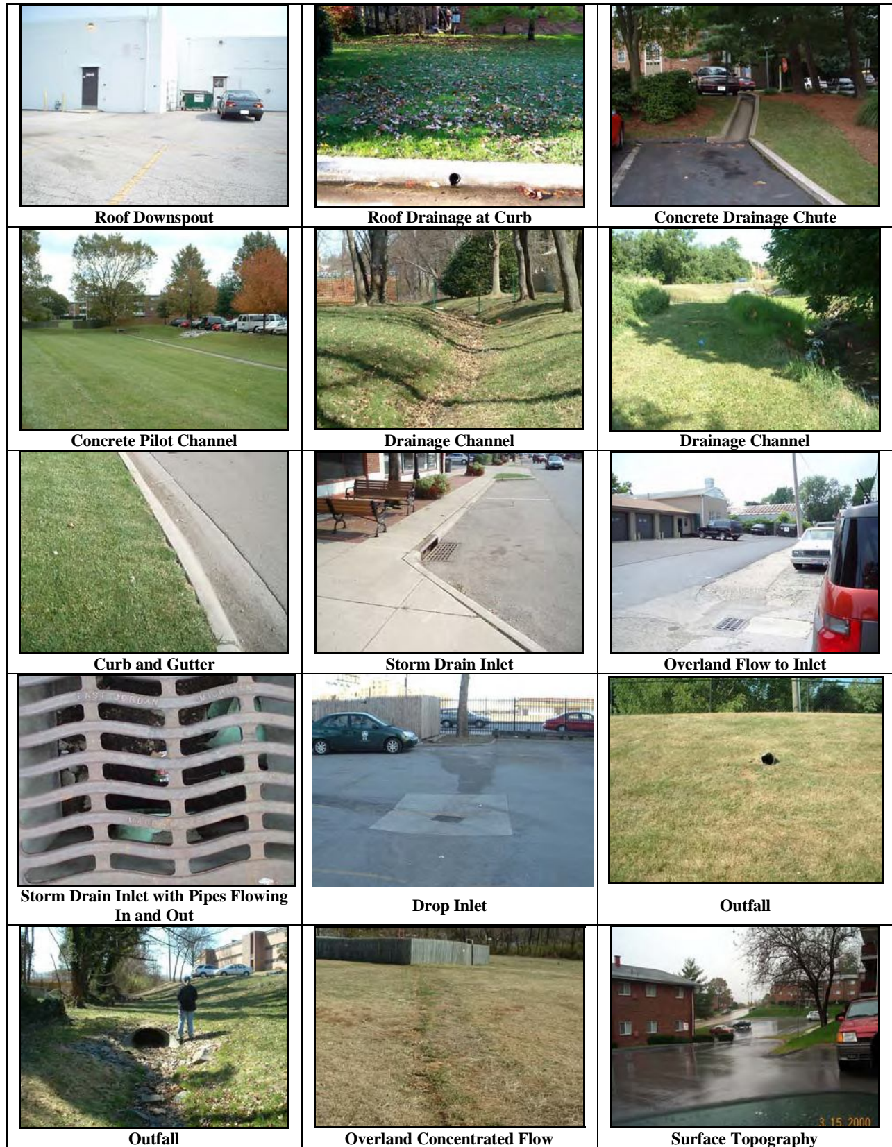
Figure 4.5: Examples of Stormwater Infrastructure Indicators
