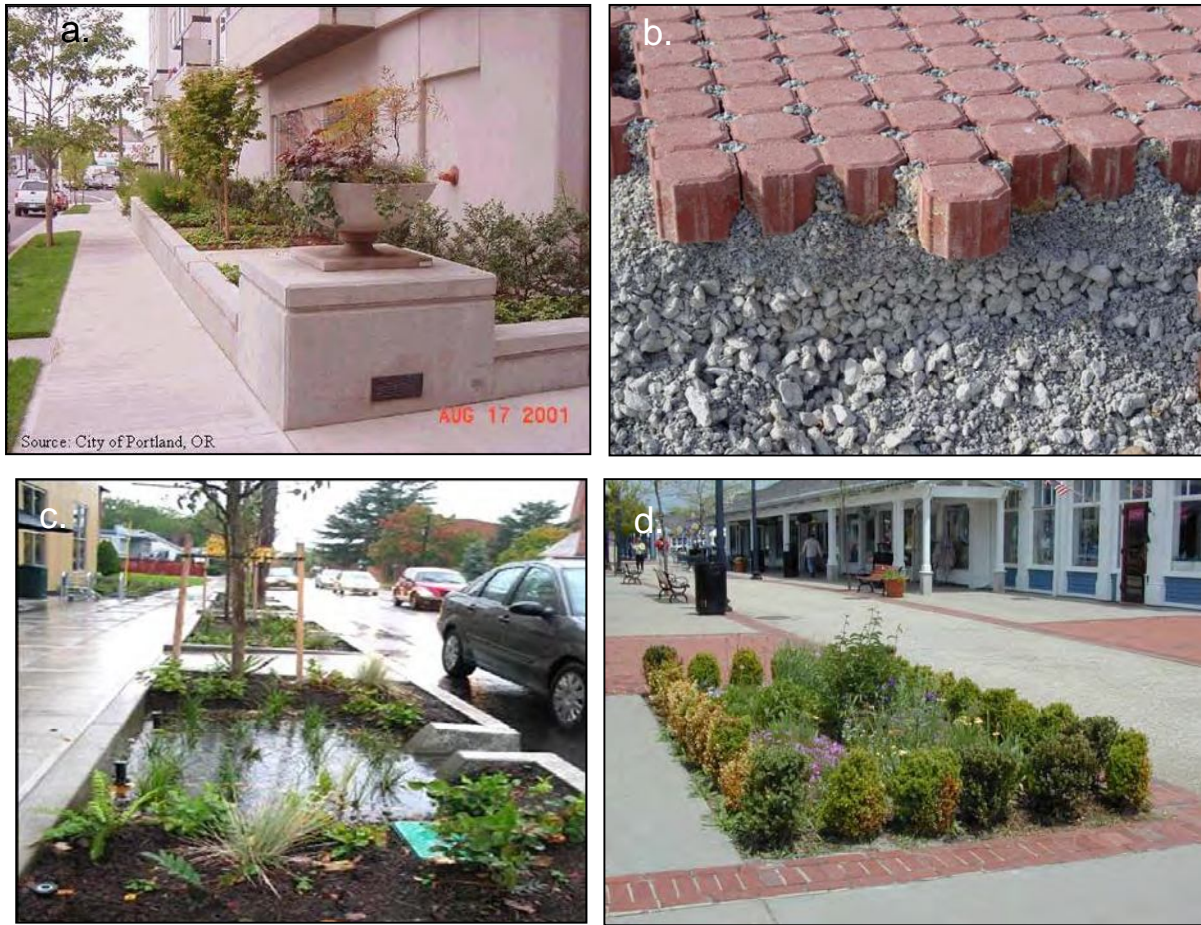
Figure 2: Landscape architects can creatively use stormwater as a resource in foundation planters (a); permeable pavers (b); bioretention (c); and stormwater tree pits (d).
