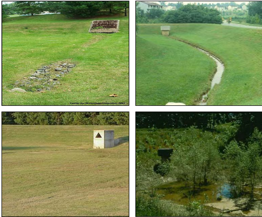
Figure 2: Older stormwater detention ponds are an attractive retrofit target
