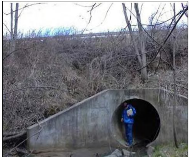
Figure 5: Field crews measure culvert dimensions and examine upstream and downstream conditions.
