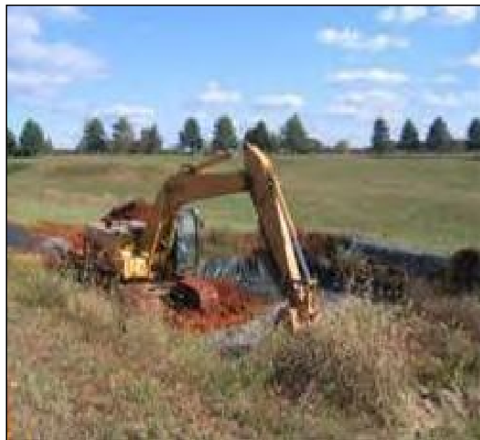
Figure 11: Specialized equipment is needed to work within tight project boundaries.
