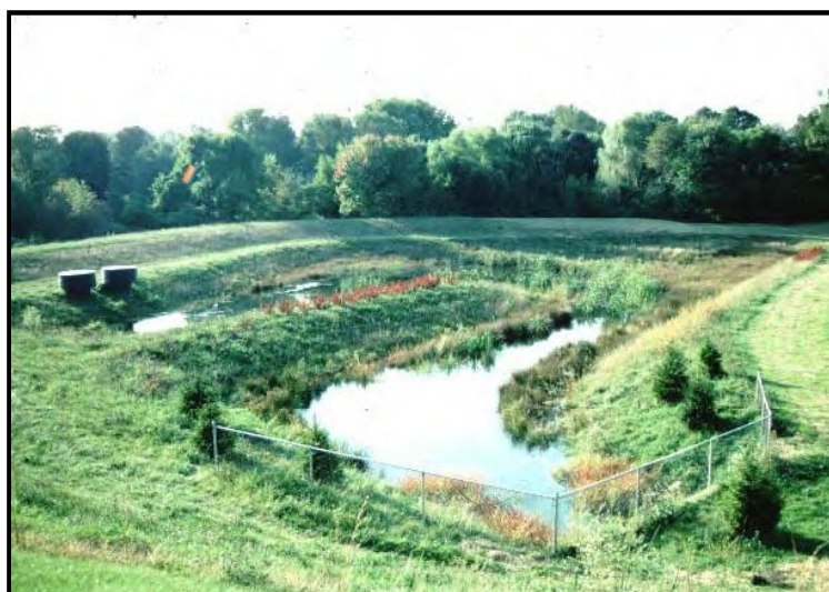
Figure 1: This shallow wetland was designed with extended detention. (Rolling Stone retrofit, Montgomery County, MD)
