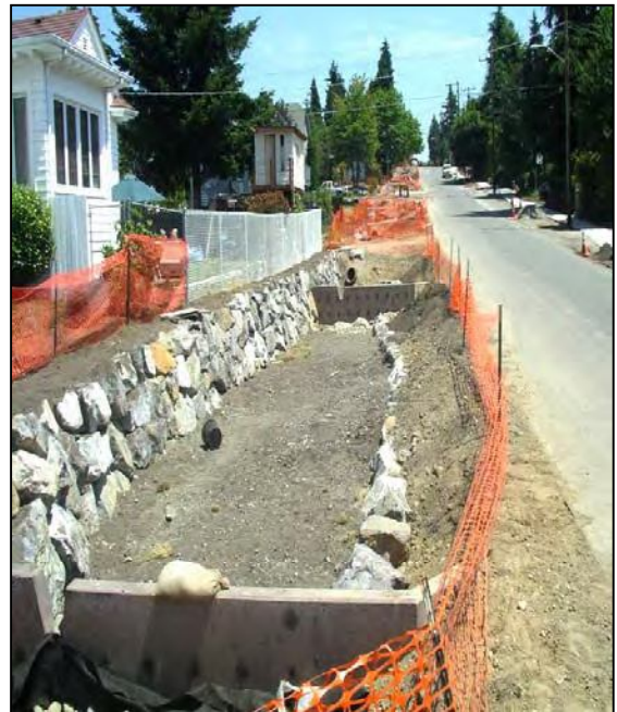
Figure 10: Construction sequencing is critical to maintain driveway access and minimize disruption to homeowners.
