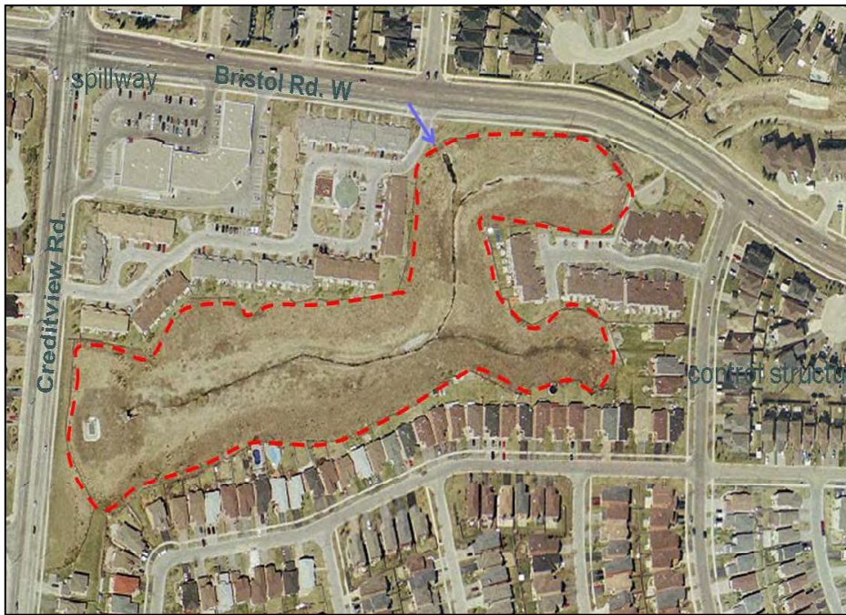
Figure 4: Dry ponds are easy to pick up on fine resolution aerial photos
