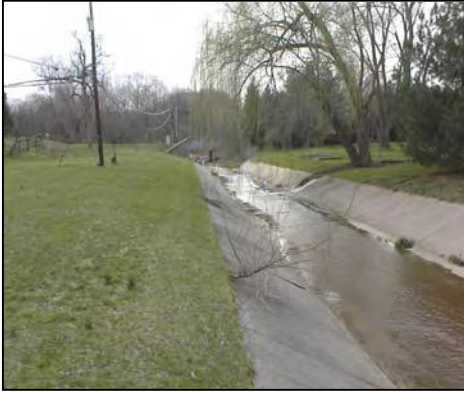
Figure 3: De-channelization and other stream repair practices are preferred when the conveyance system has perennial flow.
