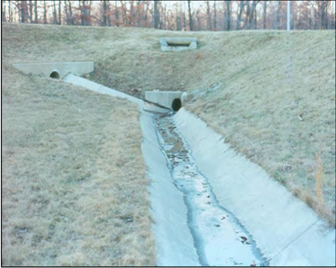
Figure 5: Multiple outlets are a clue that storage trading is a possibility
