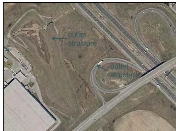
Figure 4: Highway retrofits really stand out in aerial photos, although highway drainage does not.
