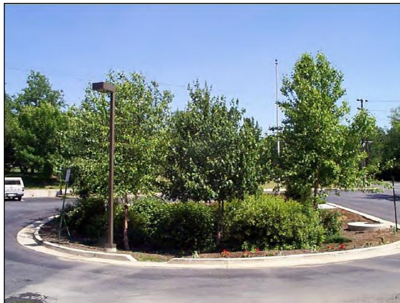
Figure 1: Bioretention created in a parking lot turn-around
