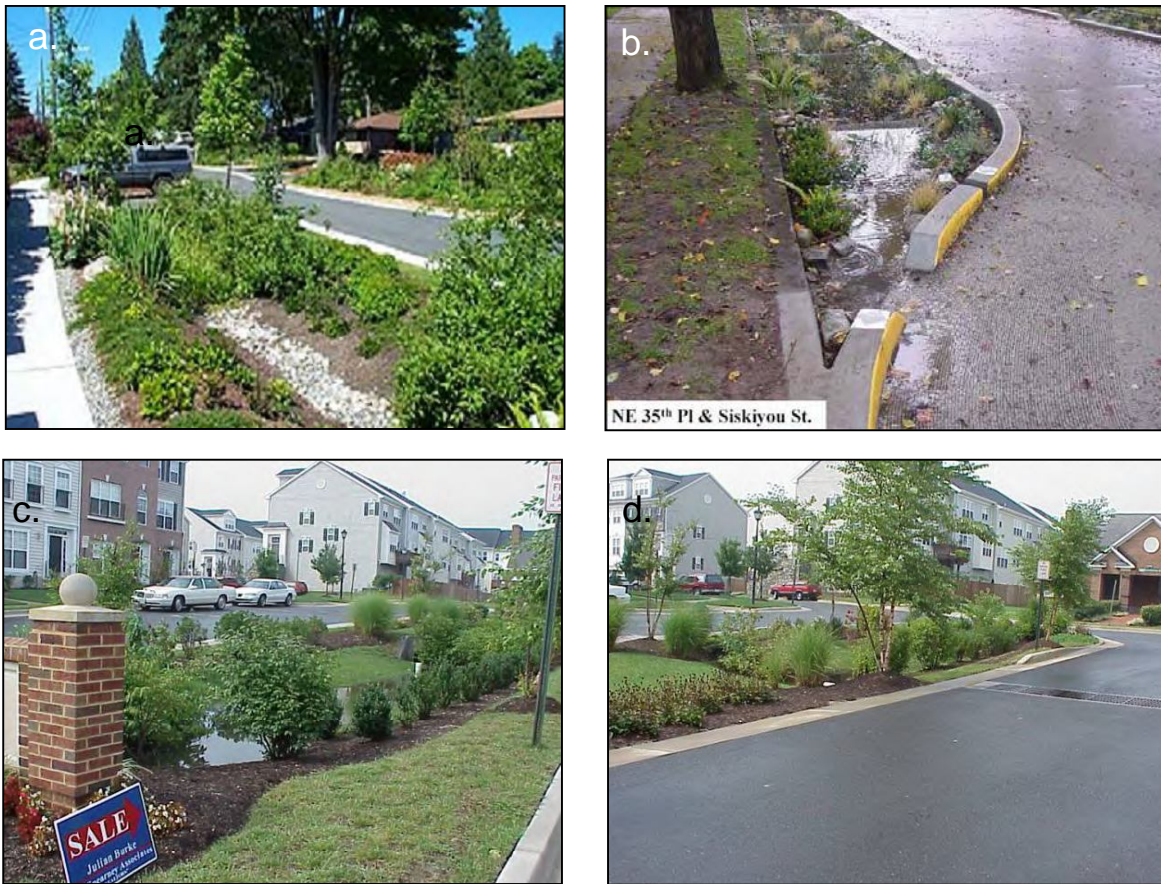
Figure 4: More street retrofit ideas: SEA streets swale (a); close-up of Portland street bioretention (b) and bioretention in street medians (c/d).
