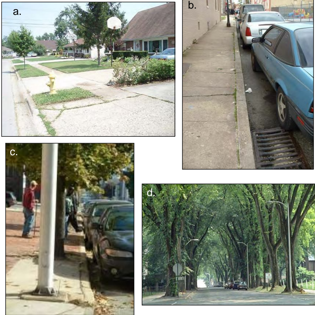
Figure 6: Conditions that make street retrofits difficult include: small lots and multiple driveways (a), on-street parking demand (b), underground and overhead utilities (c), and mature street trees (d).
