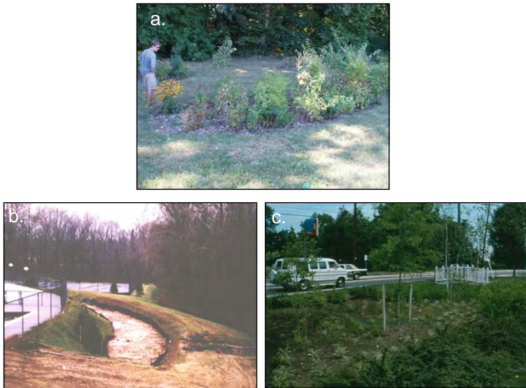
Figure 1: Examples of little retrofits serving small impervious areas: a rain garden treating runoff from a trail (a); surface sand filter treating tennis court (b); and bioretention treating a small courtyard (c).
