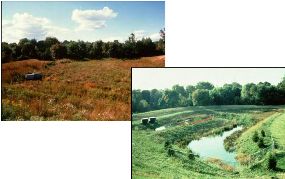
Figure 9: The Rolling Stone retrofit: before and after
