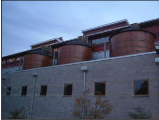
Figure 1a: Wooden Cisterns at the Chesapeake Bay Foundation Headquarters
