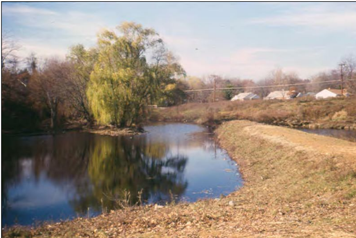
Figure 12: This under-sized forebay filled up with sediment within five years of retrofit construction.
