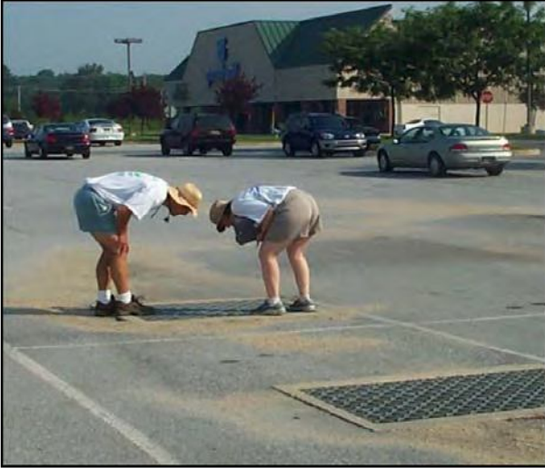
Figure 5: The crew should check out the internal plumbing of the lot to see where runoff goes.
