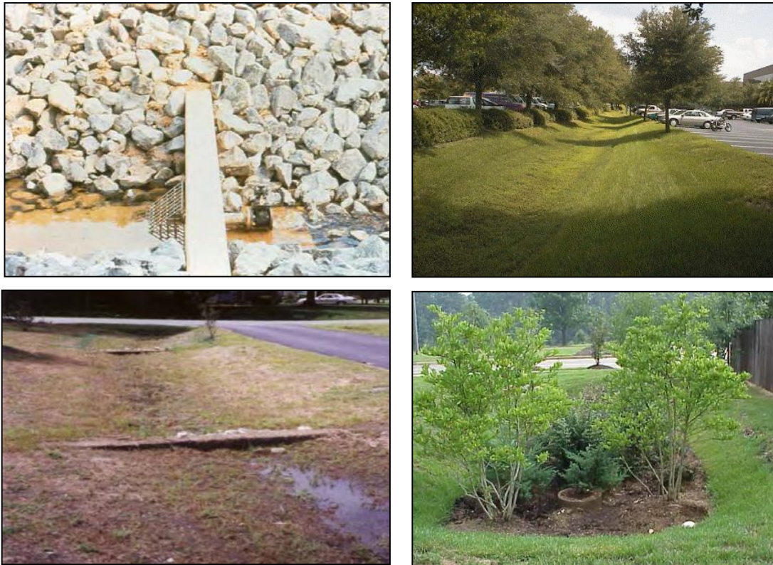
Figure 10: Four examples of conveyance retrofits.
