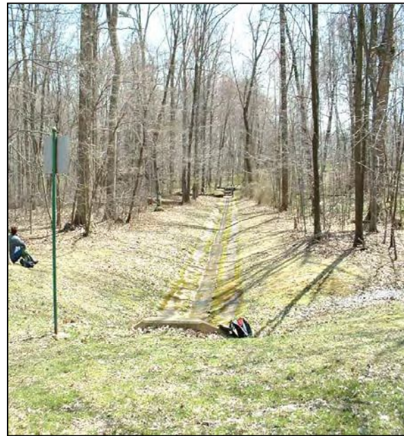
Figure 4: Example of a “cutoff” outfall discharging well away from the stream
