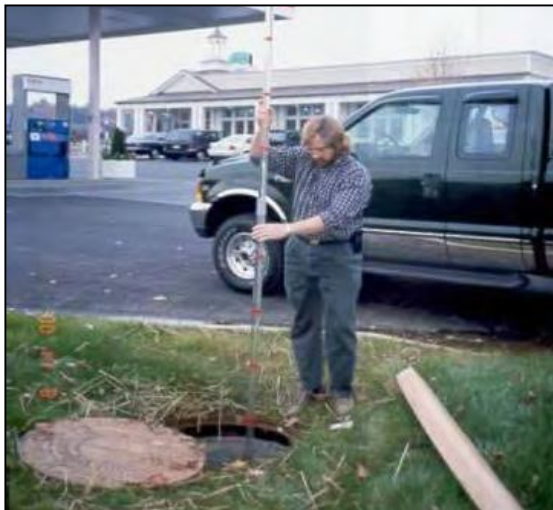
Figure 5: Out of sight means out of mind – make sure inspectors can access underground retrofits.
