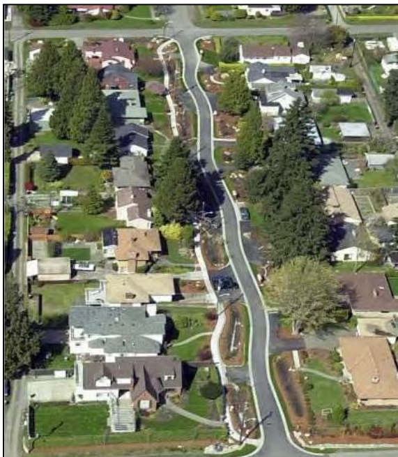
Figure 9: Aerial shot of Seattle SEA Streets retrofit.
