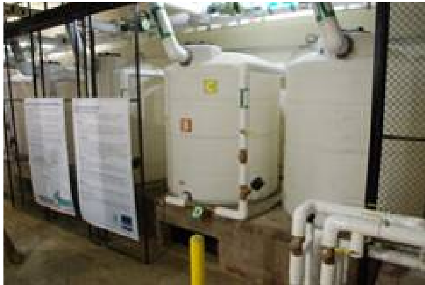
Figure 65. Six (6) 1,000 gallon cisterns at U.S EPA headquarters provide water for irrigation Source: U.S. EPA
