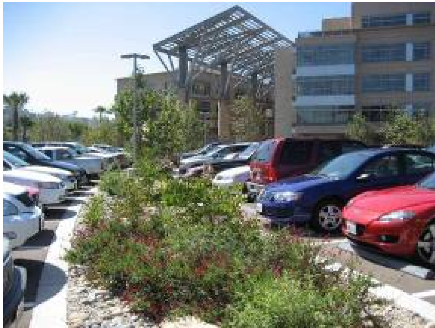
Figure 17. Bioretention Cell in Parking Lot, Caltrans District 11 Headquarters, San Diego, CA.
