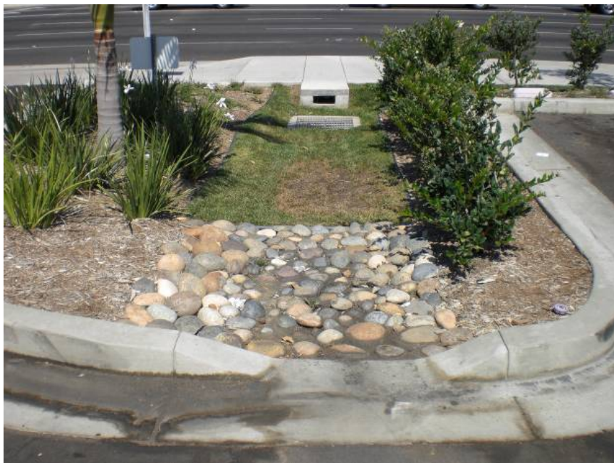
Figure 27. Inlet Structure, Downey, CA. Source: Bill DePoto
