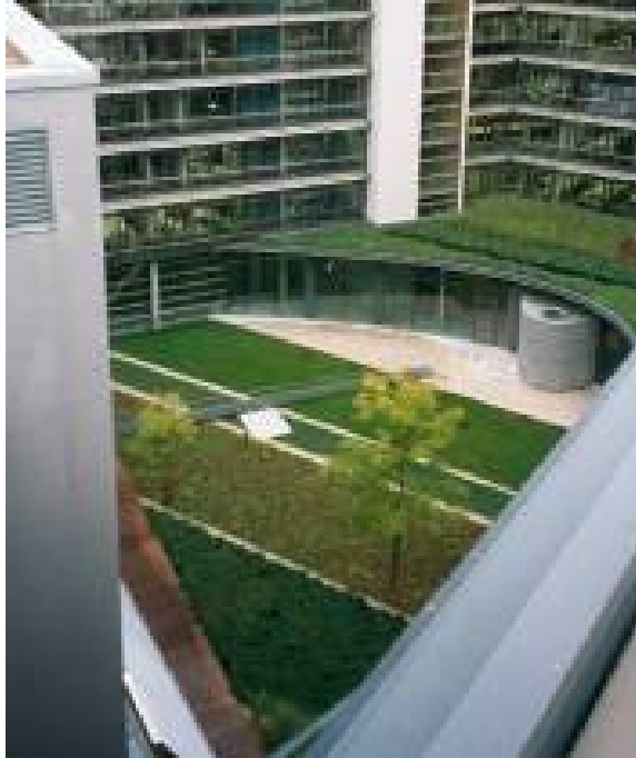
Figure 64. Large cistern for vegetated roof plaza maintenance. Source: Cahill Associates
