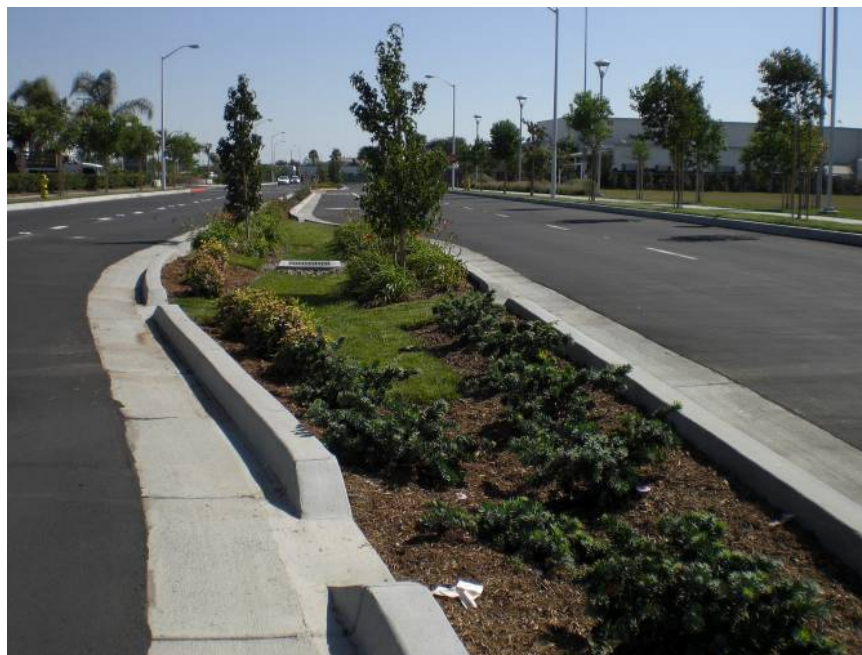
Figure 24. Bioretention cell for street/yard drainage, Downey, CA. Source: Bill DePoto
