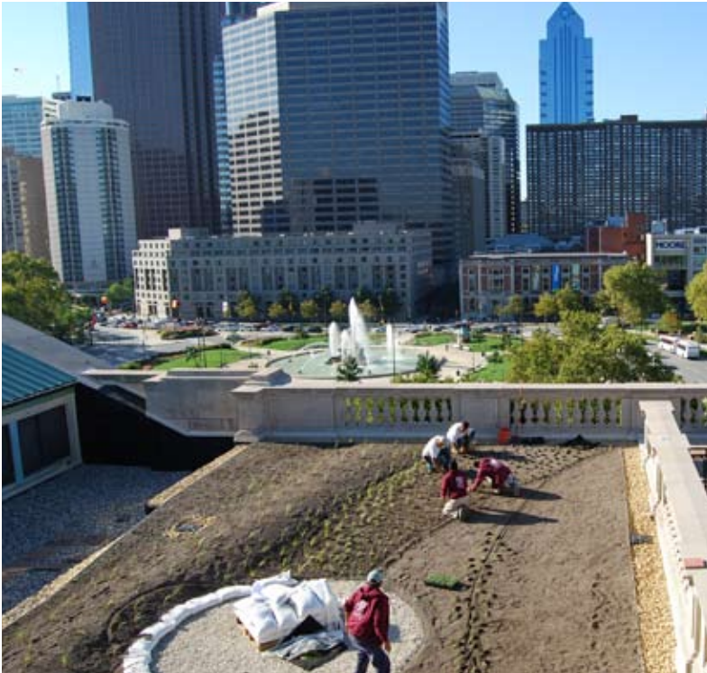
Left: Green roof being planted on the Free Library of Philadelphia in the Schuylkill Watershed.
