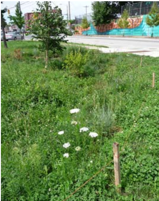
Above: Street runoff is captured at this rain garden at 47th St. and Gray's Ferry Ave. in the Combined Sewer Area within the Schuylkill River Watershed.
