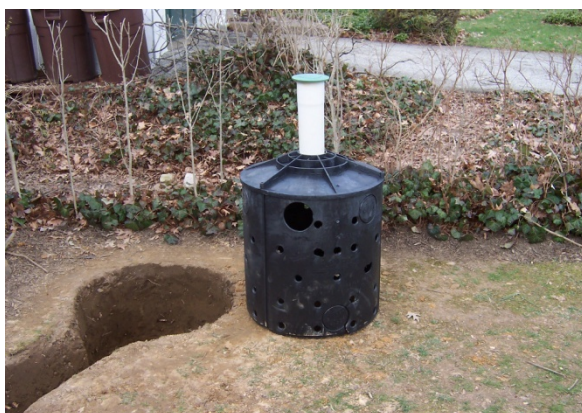
Drywell installation
