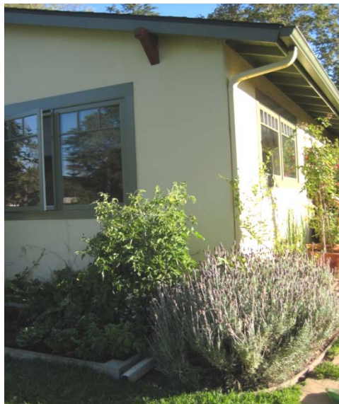
Diverted Roof Runoff City of Santa Barbara
