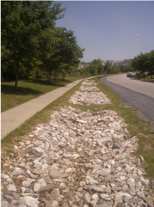
Rural Highway Infiltration Trench
