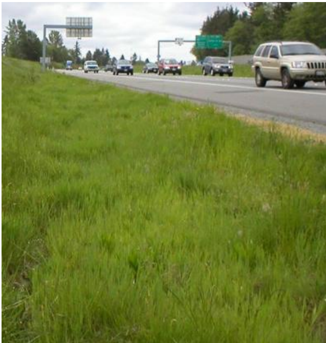
Vegetated filter strip captures runoff from freeway
