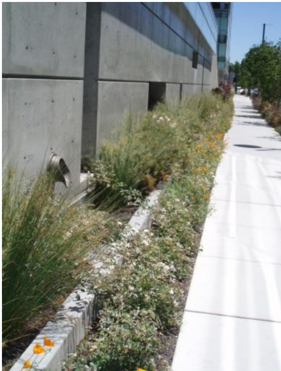
Planter boxes extending along a building wall
