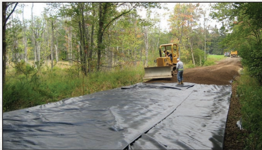
Figure 2.23—Geotextile fabric provides support for permeable fill.
