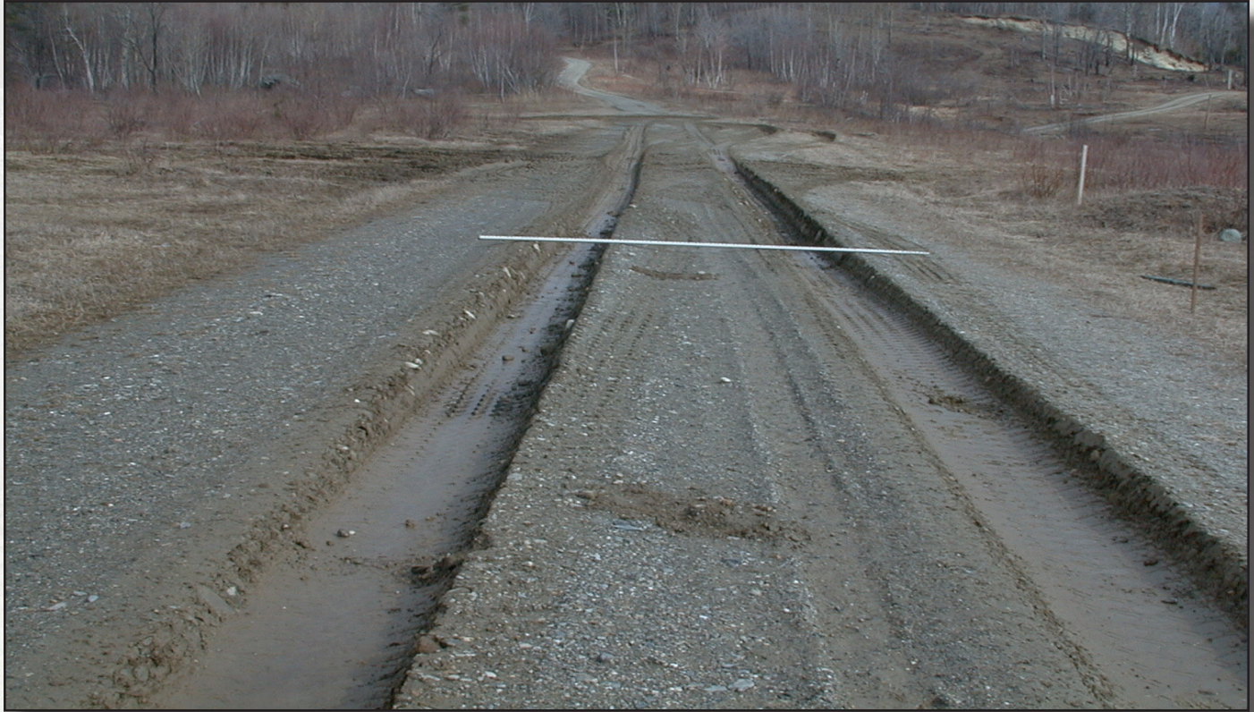
Figure 8.1—Proper gradation of aggregate can prevent the raveling and pumping in this picture.
