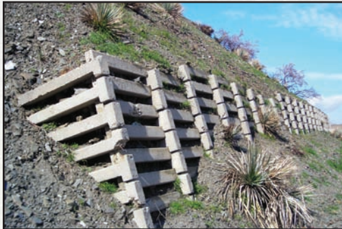
Figure 7.6—Crib wall stabilizes this steep cutslope ensuring appropriate road width and drainage function.
