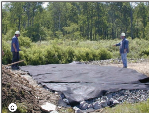
Figures 2.16a through 2.16d—French mattress construction sequence.
