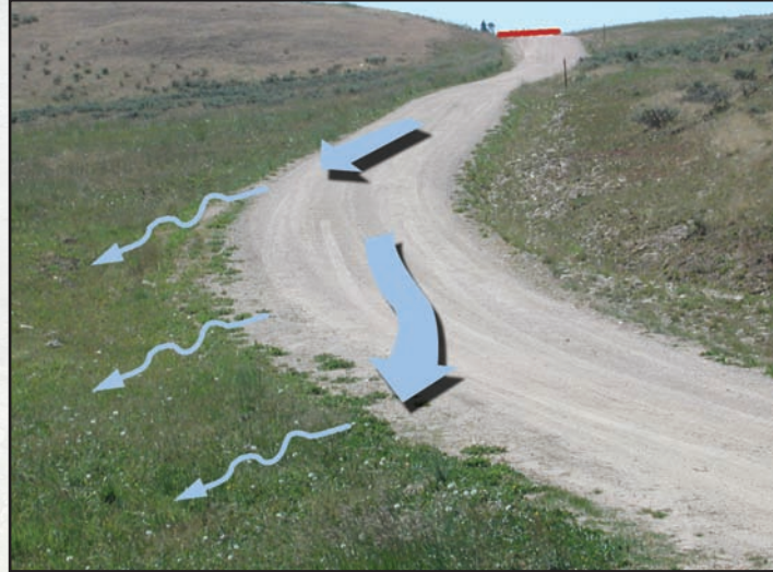
Figure 3.4a—Outsloped road disperses flow.
