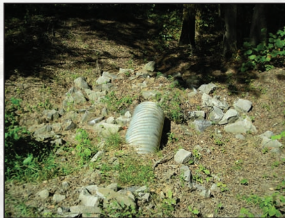
Figure 5.3—Culvert outlet is well armoured.
