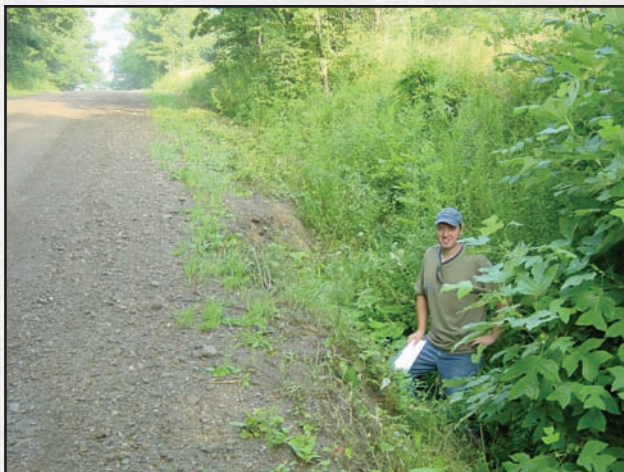
Figure 4.2—This photograph is taken only 300 feet from the top of the hill, yet the road ditch is over 5 feet deep. Further investigation of the site revealed a large amount of water emptying out of a meadow and into the road ditch. This water should be either diverted before it reaches the road or handled as quickly as possible and not allowed to flow down the road ditch.
