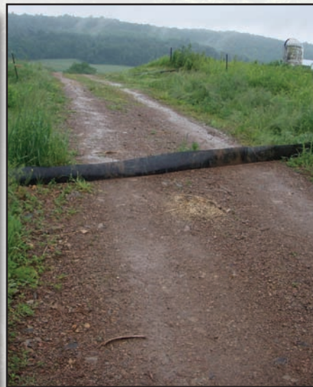
Figure 3.13—Conveyor-belt diversion on a farm lane (road).
