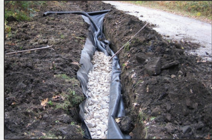
Figure 2.7—Free draining stone.
