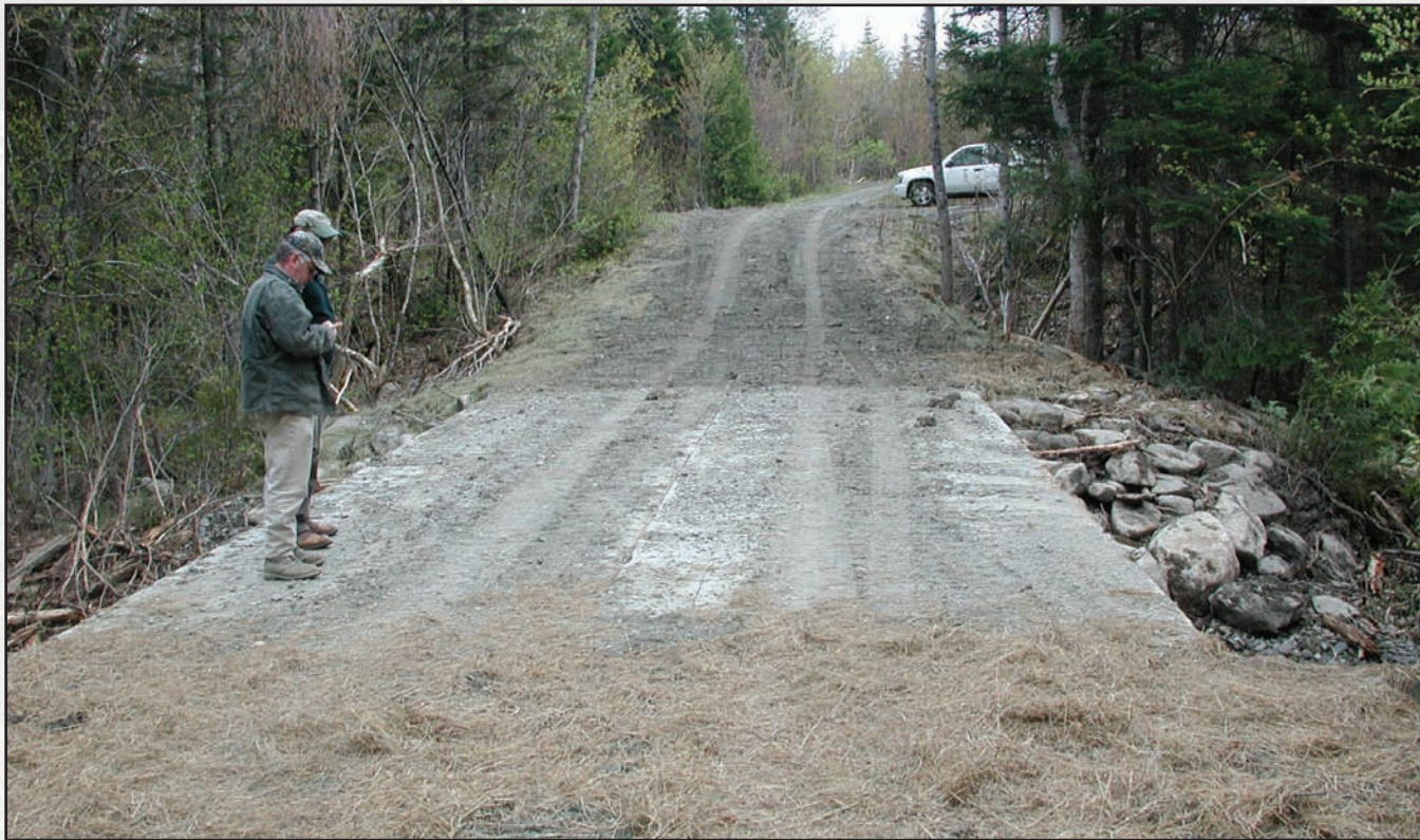
Figure 9.1—Road Assessment and monitoring.
