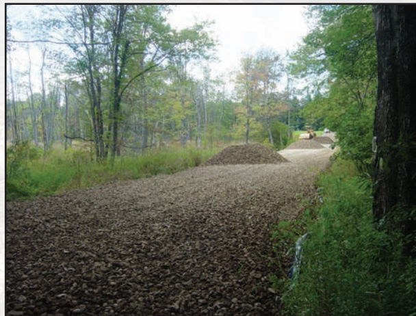
Figure 2.15b—Large mattress allows wetland flow.
