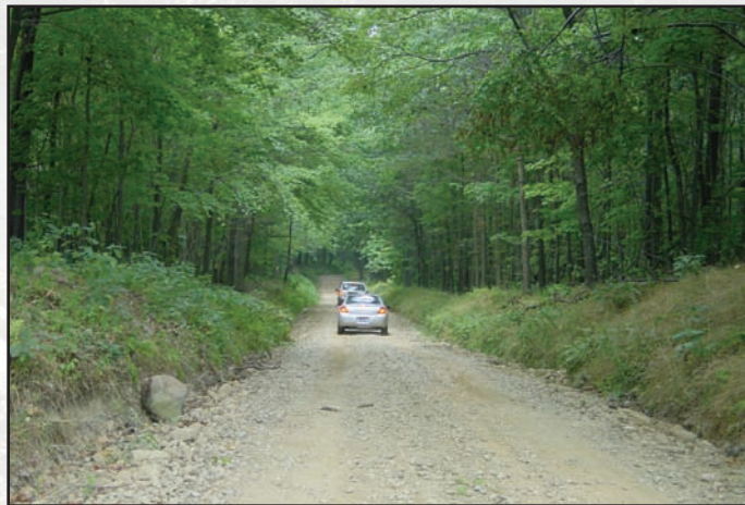
Figure 4.7—Example of an entrenched roadway.
