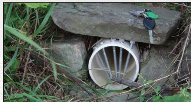
Figure 2.10—This homemade guard will prevent animals from entering the underdrain outlet.
