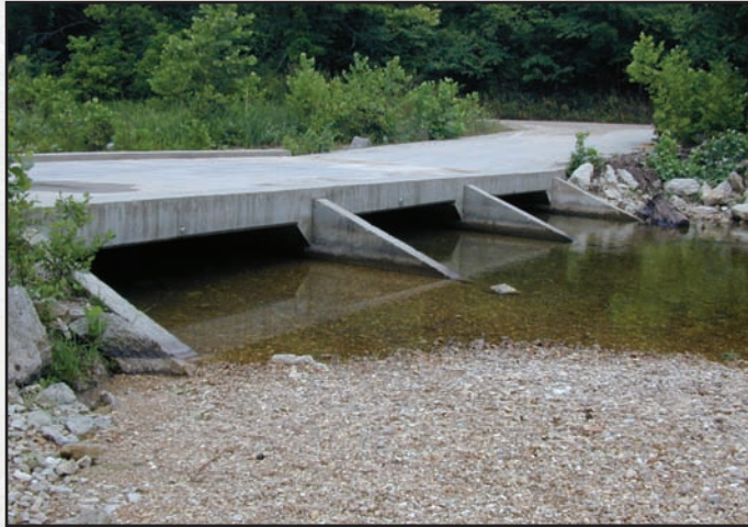
Figure 6.7—Vented ford or low-water bridge.
