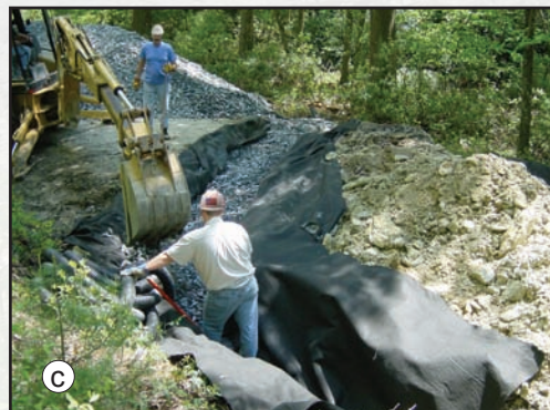
Figures 2.8a through 2.8d—French drain construction sequence.
