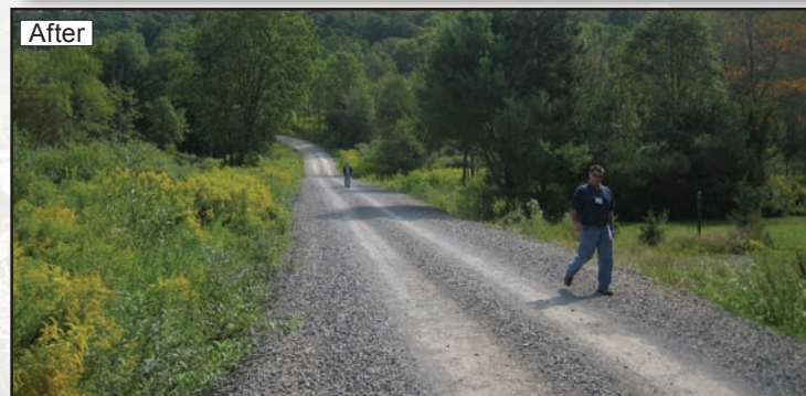
Figure 2.17 and 2.18—This roadway cuts across a flood plain wetland. A 300-foot-long French mattress was used to provide relief for wetland flows while providing a stable road base and preventing beavers from damming the nearby stream pipe.
