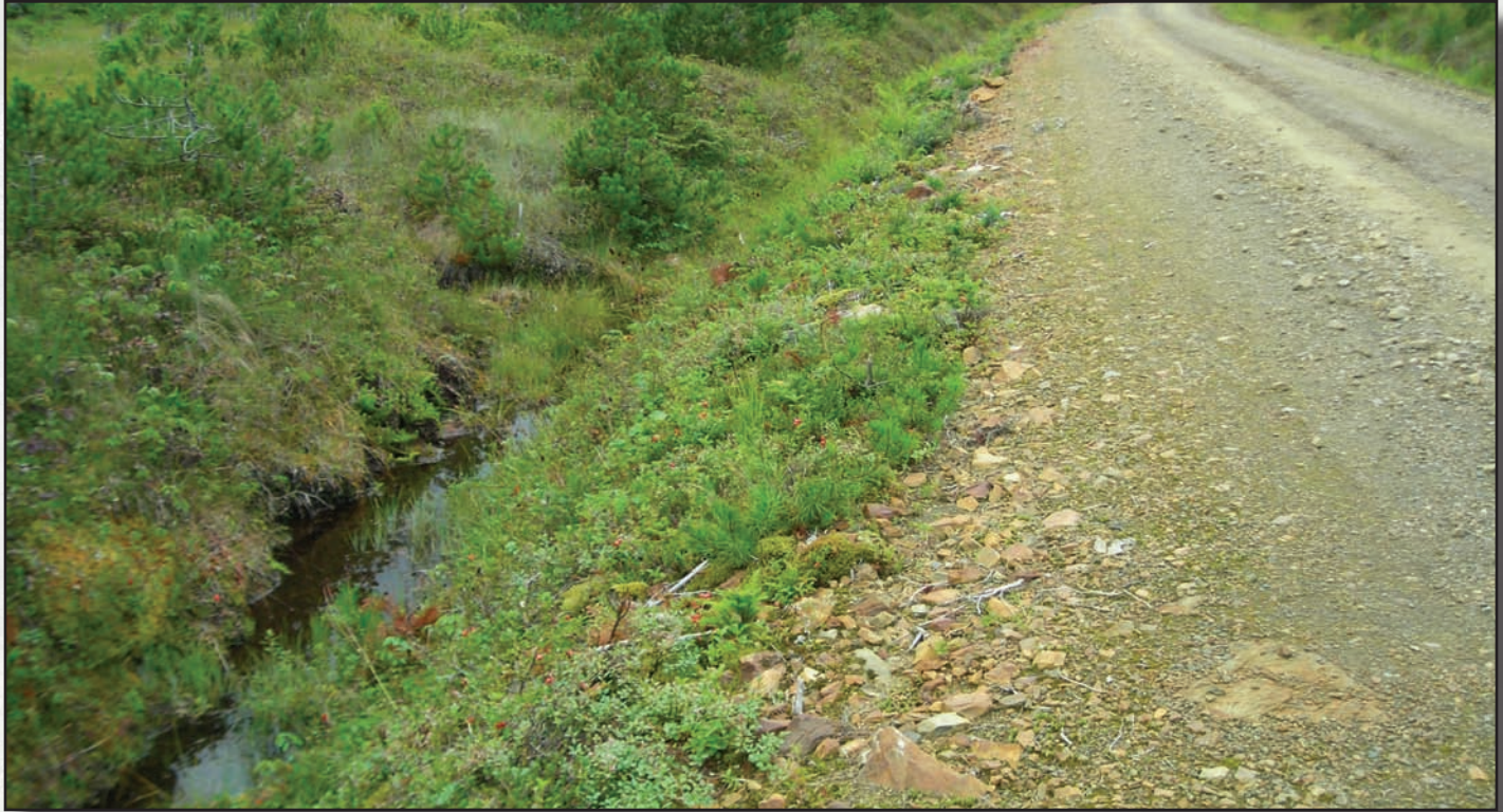
Figure 2.1—Permeable fill provides for subsurface flows.
