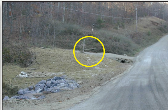
Figure 7.14—The broad-based-dip on this driveway provides a good transition and keeps water off the public road.
