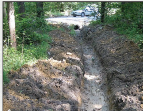
Figure 5.5—Traditional deep pipe. It has a long outlet trench requiring continual maintenance.
