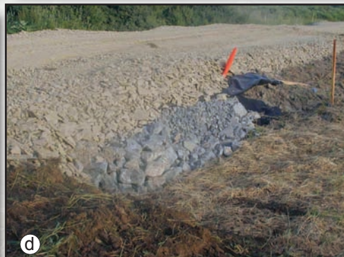
Figures 2.16a through 2.16d—French mattress construction sequence.
