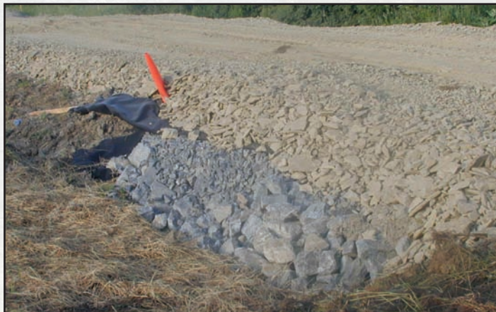
Figure 2.11—Side view of a large French mattress.
