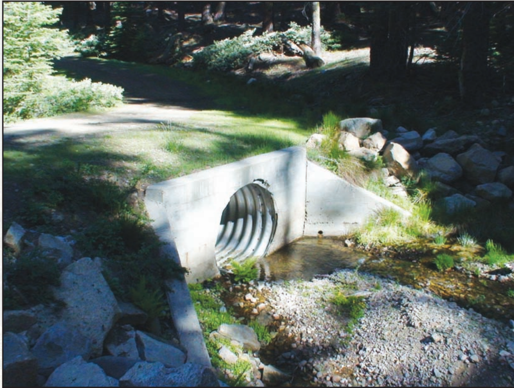
Figure 5.14—Headwall with wingwalls.
