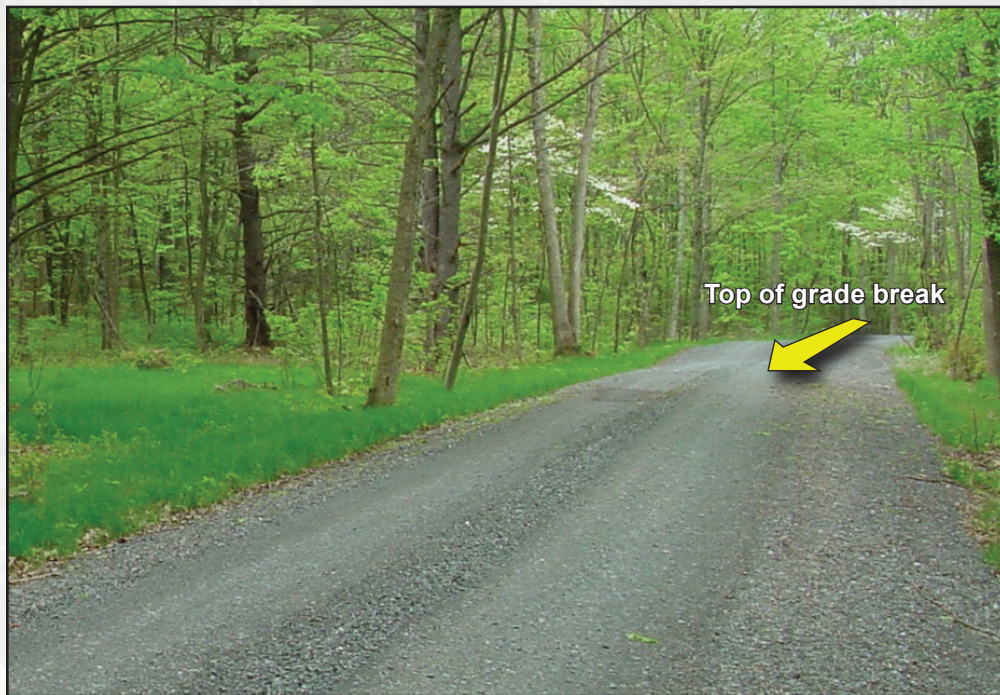
Figure 3.8—A grade break, such as the one pictured in the distance, should be big enough to shed water, but gentle enough to allow traffic passage.
