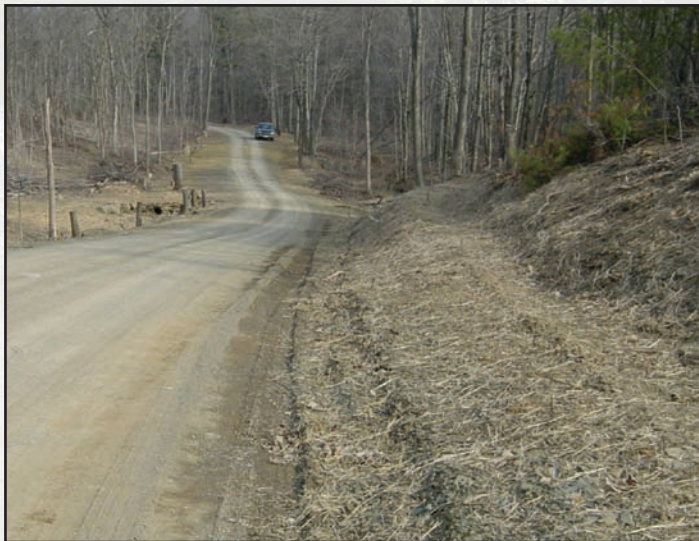
Figure 7.10—The slightly insloped bench in this image takes water around the hill and away from the road.
