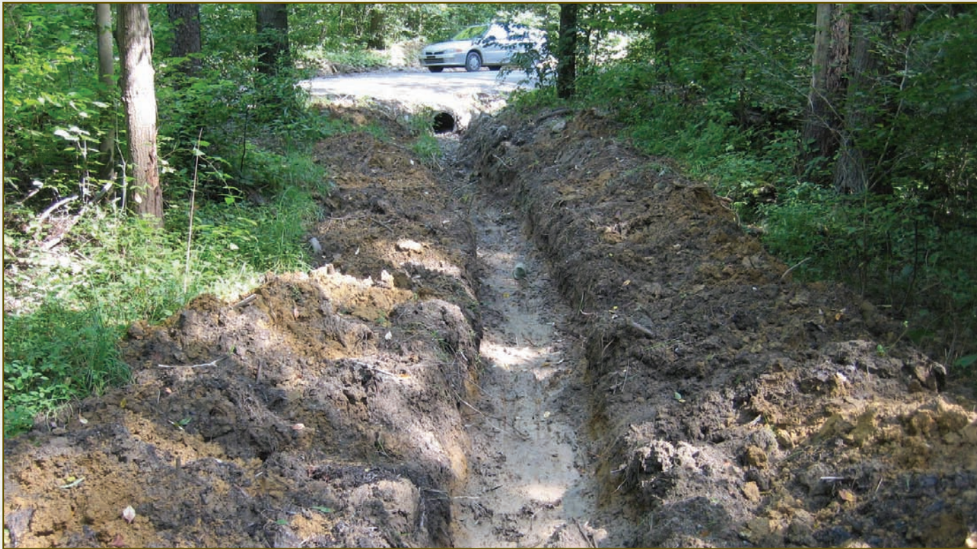
Figure 5.1—Culvert placed below the natural elevation requires frequent maintenance and long ditch outlets.
