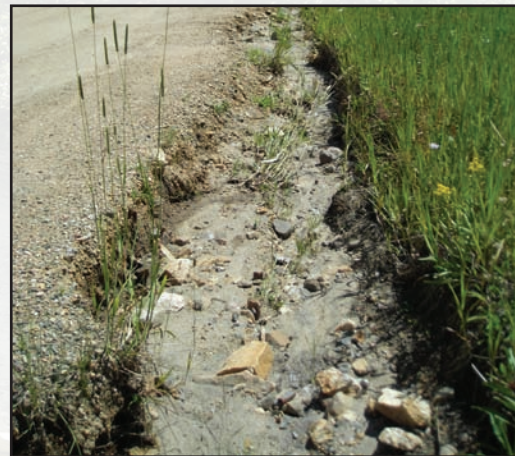
Figure 4.19—Unstable ditch. This ditch presents a safety, maintenance, and environmental concern. It is too deep, too wide, unvegetated, and can route sediment to the stream.
