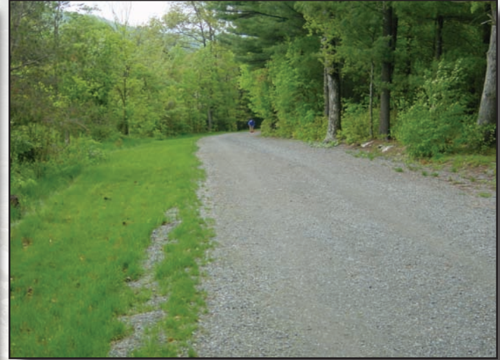
3.4b—Outsloped roads eliminates ditches.
