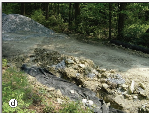
Figures 2.8a through 2.8d—French drain construction sequence.
