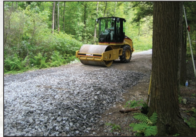
Figure 2.25—Roller compacts each of lift aggregate.
