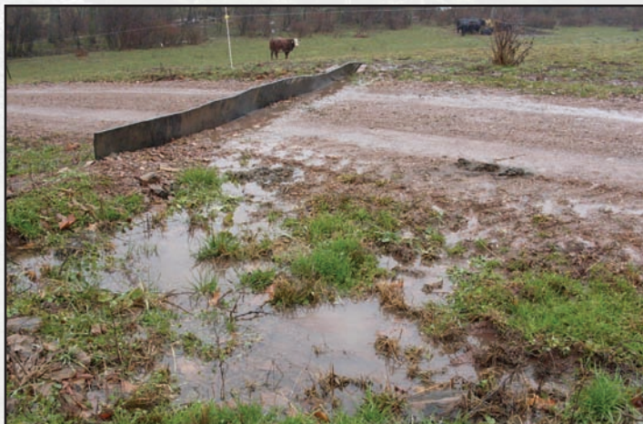
Figure 7.13—This conveyor-belt diversion on a farm access lane prevents drainage from flowing on to the public road at the bottom of the hill.
