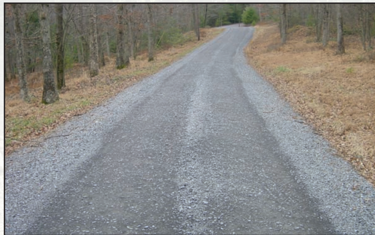
Figure 8.4—Loose aggregate will unravel and form windrows of material along the road center and edge.
