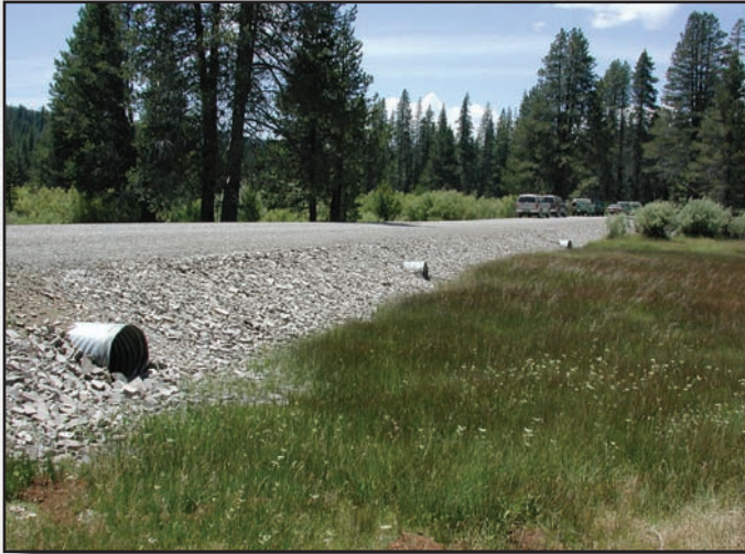
Figure 2.20—Permeable fill with culverts.
