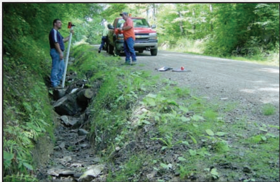
Figure 4.4—This eroded ditch is a symptom. The problem is excessive water volume for this road gradient and soil, and must be managed upslope.
