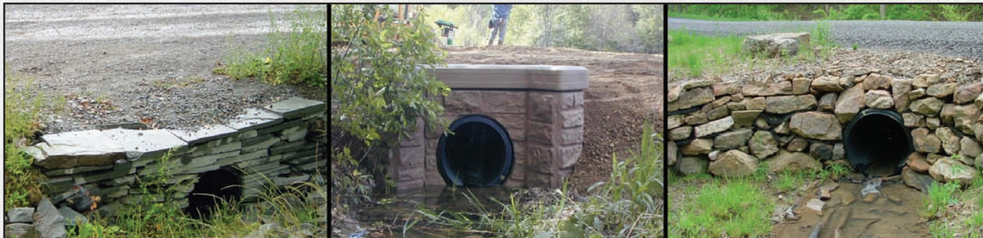
Figure 5.11—Headwalls come in various shapes, sizes, and materials, based on the situation and material available.
