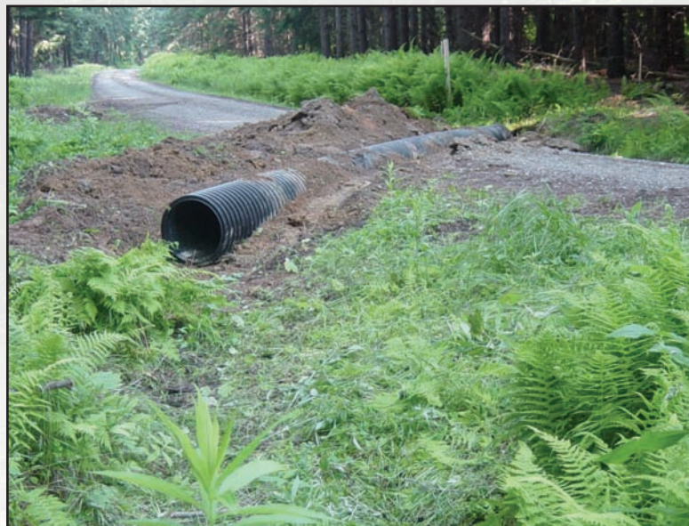
Figure 5.7—A shallow cross pipe being installed: The cross pipe shown is partially installed. Notice that the pipe outlet is at the elevation of the existing ground, no outlet trench or tail ditch is required. The top of the pipe is ABOVE the existing road surface. The required pipe cover is obtained by importing fill. When completed, the fill will create a grade break over the pipe.
