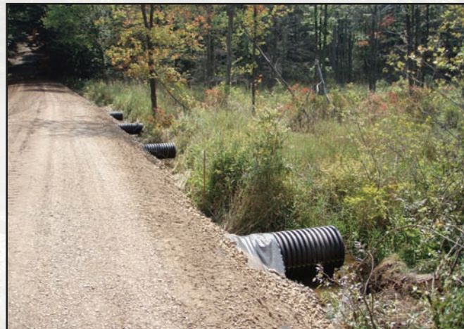
Figure 2.19—Permeable fill with culverts spreads surface flows.
