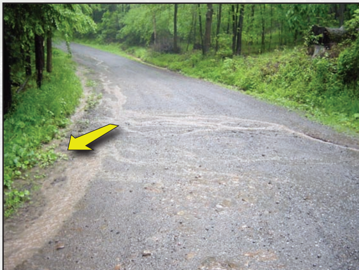
Figure 4.14—Berms can range from several feet high to only a few inches high as pictured here. The small partially vegetated berm on the left is preventing runoff from exiting the road surface. A stable vegetated buffer exists to the left, but the berm is causing an unnecessary ditch to form at the road edge.
