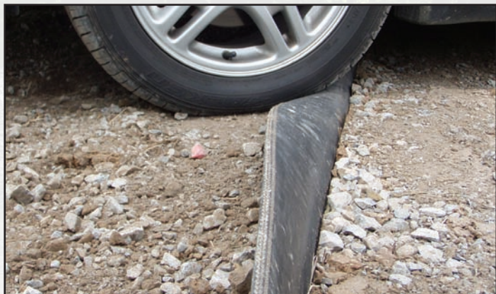
Figure 3.14—On most roads a completed diversion should leave no more than 4 inches of belt exposed.
