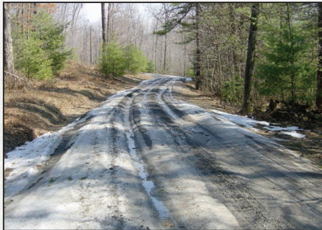
Figure 8.2—Rutting due to excess clay content.
