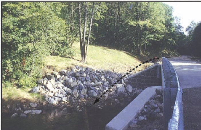
Figure 4.22a—Before: A typical crossing with ditches armored with rock and draining directly into the stream.
