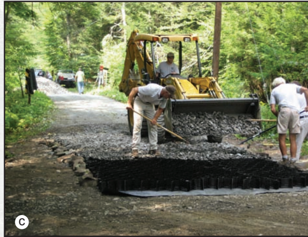
Figures 6.4a through 6.4d—Construction sequence for high-water-bypass.
