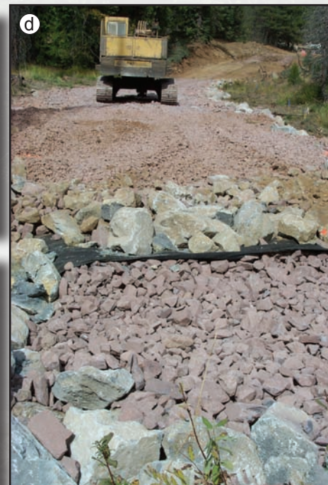
Figures 2.22a through 2.22d—Permeable fill construction sequence.
