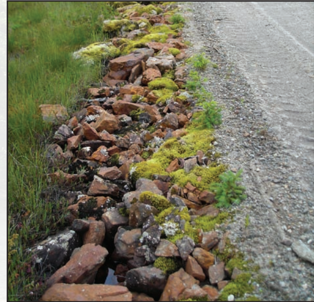
Figure 2.21—Permeable fill without culverts.
