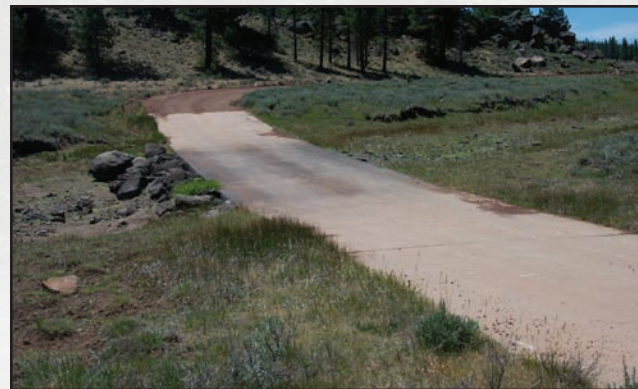
Figure 6.5—Concrete ford crossing.
