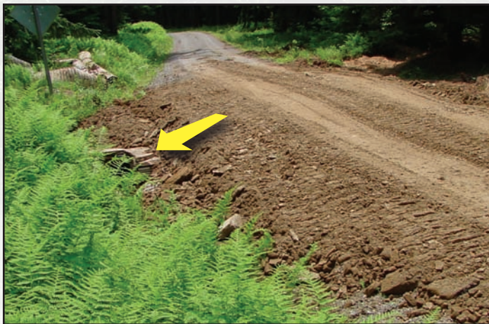
Figure 5.8—The same pipe is shown here covered with fill, before final compaction. Arrow denotes headwall or pipe inlet.
