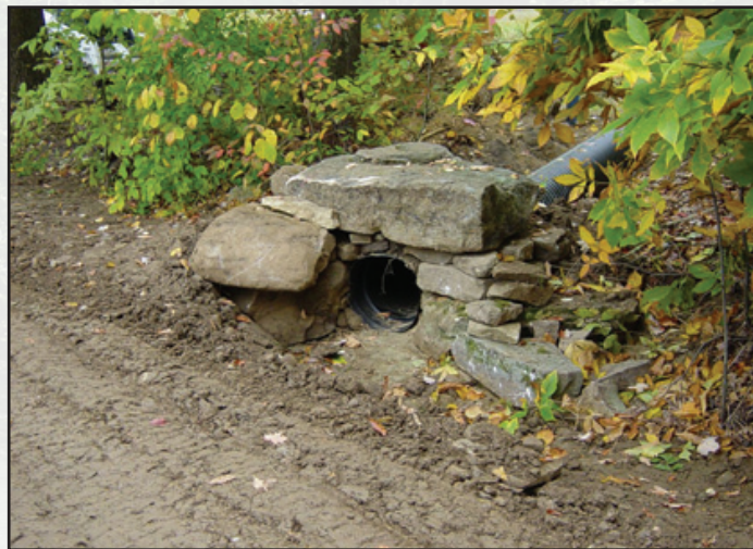
Figure 5.10—The inlet of a through-the-bank pipe shown during installation before the pipe is covered.
