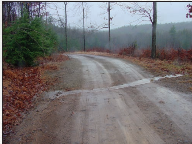
Figure 3.10—The broad-based dip pictured here conveys water from the road surface and upslope ditch into a vegetative filter area on the right.
