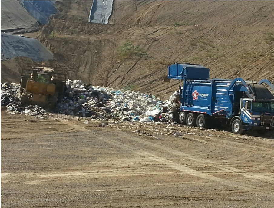
Figure 2: Municipal solid waste being placed in the Stage III-C unit on July 13.
