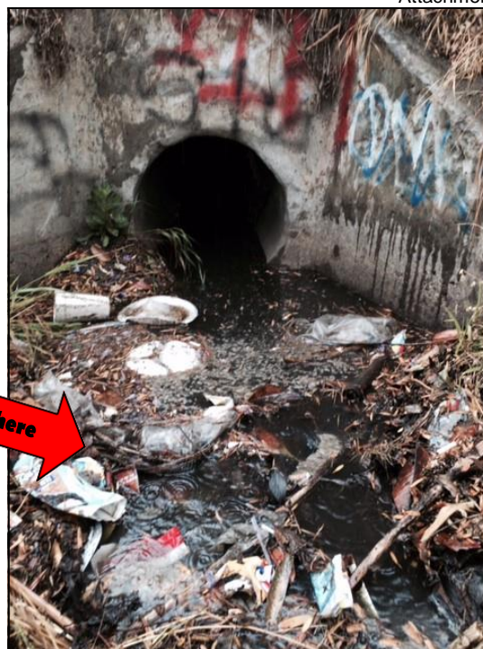
Figure 3. Stormwater runoff containing food and beverage containers in the Tijuana River watershed.
