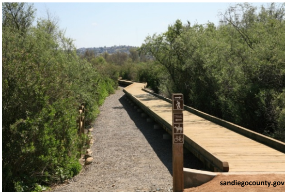
Dairy Mart Boardwalk
