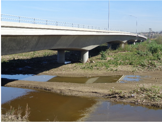
Figure 5 Tijuana River at Dairy Mart Bridge
