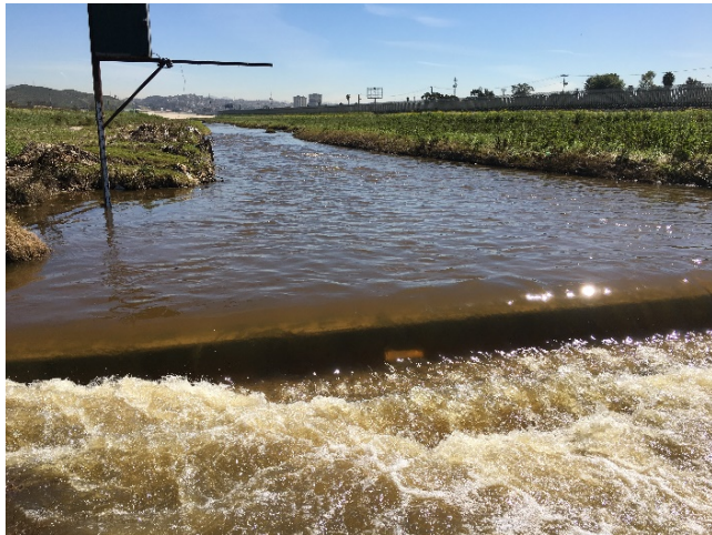
Figure 6 Tijuana River at IBWC gaging station, March 8, 2017
