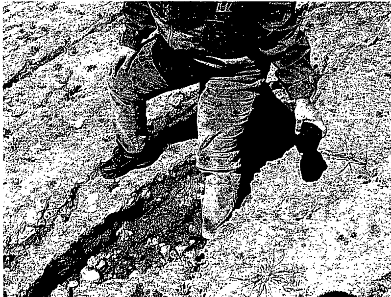
Photo #4, taken around 10:45 a.m. Erosion gully on southern sideslope, approx. one foot deep.
