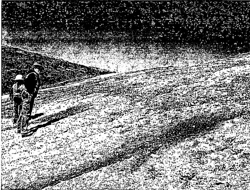
Photo #3, taken around 10:30 a.m. Two areas of stained soil on southern sideslope. Both stained areas seem to originate from the same elevation.
