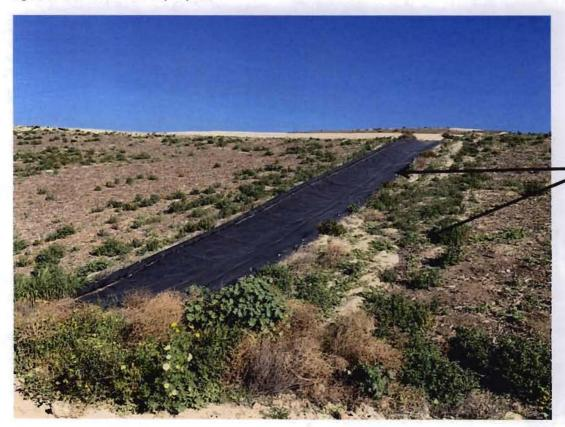
Side slope adequately vegetated. Drainage feature clear of any debris.
