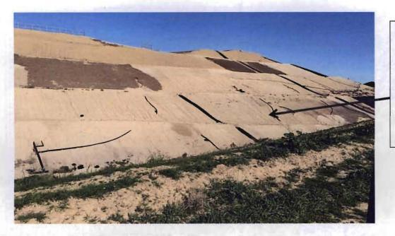
Signs of erosions evident all over the side slope. No vegetation observed on the side slopes. The side slope is not implemented with erosion BMPs.
