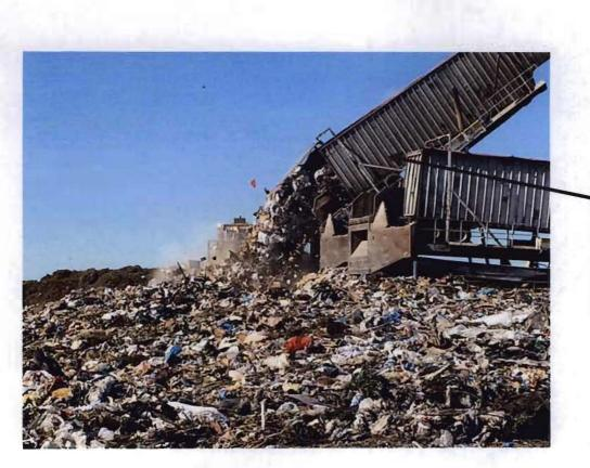
Three tons of municipal solid waste being dumped in active portion of landfill from transfer station.
