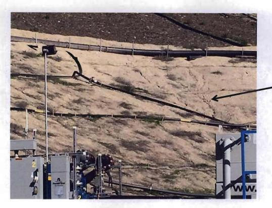
Signs of erosion evident on the side slopes.
