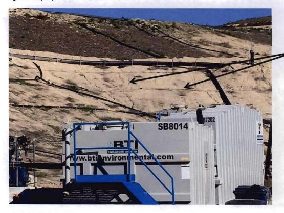
Signs of erosion evident on the side slopes. BMPs are no longer functioning.
