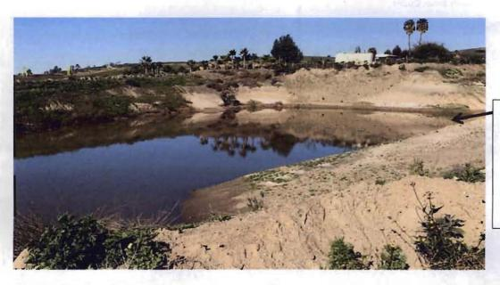
North portion of West Basin was excavated prior to rainy season with intention to keep storm water onsite for reuse for dust control.
