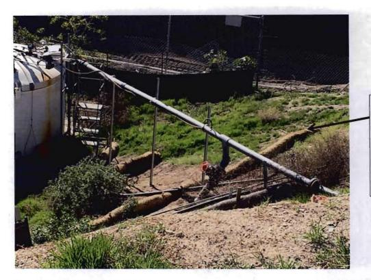
New straw wattles implemented in a lower risk area. While high risk erosion areas have failed or poorly implemented BMPs.
