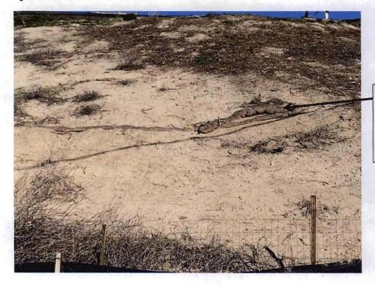
Straw wattles are no longer functioning as intended for erosion control. Straw wattles need to be replaced.
