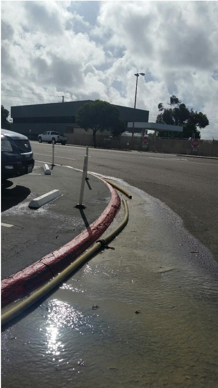
**Photo 6** shows the sediment laden storm water discharged from the site at Pacific Coast Highway onto Anna Avenue.
