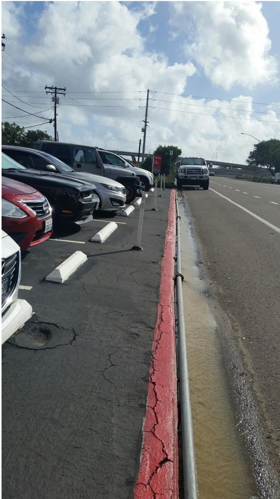
**Photo 7** shows the sediment laden storm water discharged from the site to Pacific Coast Highway.
