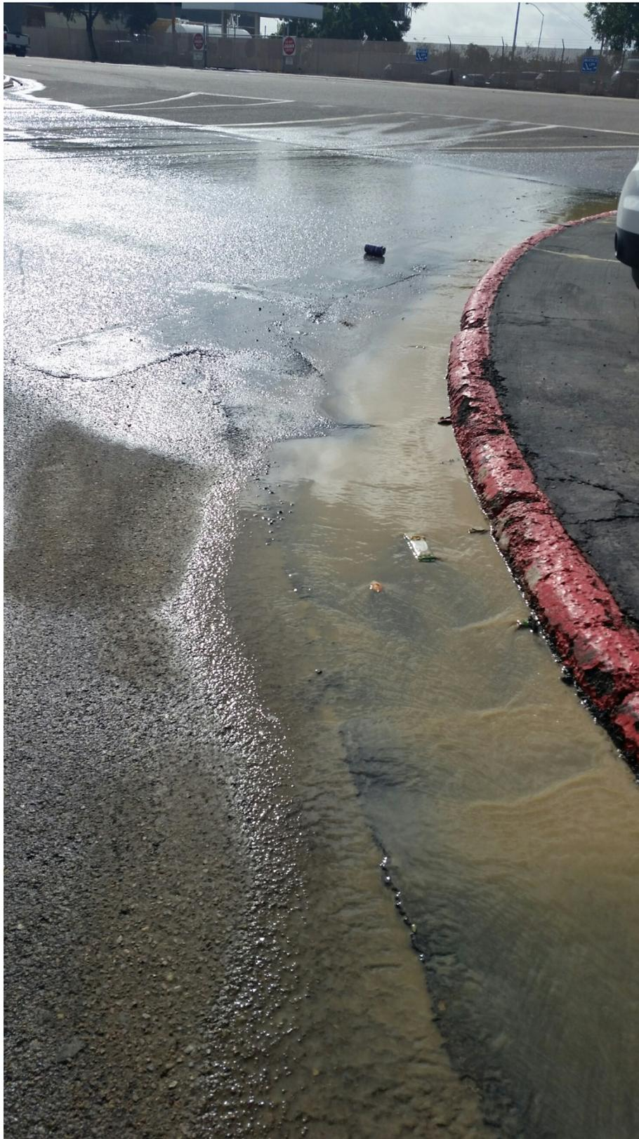
**Photo 5** shows the sediment laden storm water discharged from the site at Anna Avenue and Pacific Coast Highway.
