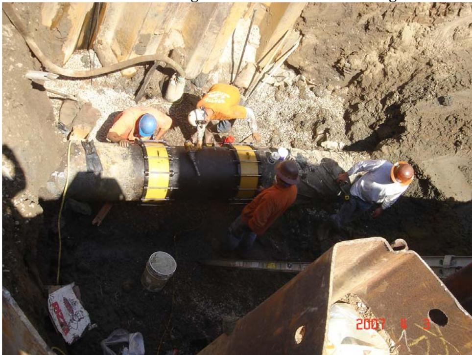
**Figure 7: Replacement Section with Couplings in Excavation**
