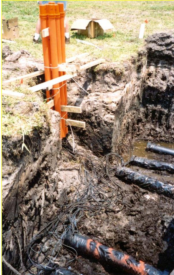
**Figure 1** – Photo of typical test pipe and monitoring station installation. Polyethylene encased pipe are shown.
