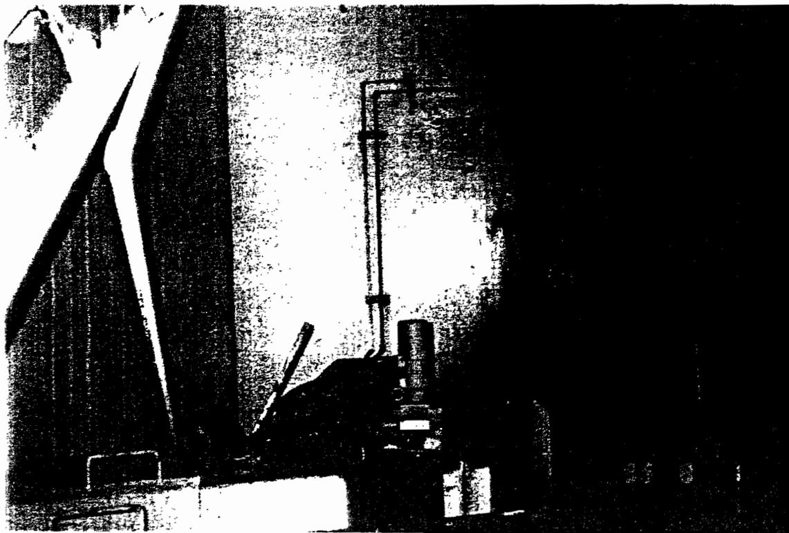
Wetwell - Class I Div. 1 requires corrosion protection
