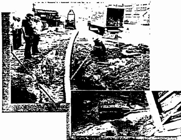
A practical and economical method for rehabilitating sewer, force main and industrial piping. Slip-lining creates a new pipe within an old one through the introduction of a high-density, polyethylene liner. It is an appropriate repair method for extensively cracked or corroded pipe, particularly if the original pipe is located in unstable soil or in an area that makes excavation and replacement impossible or too expensive.
