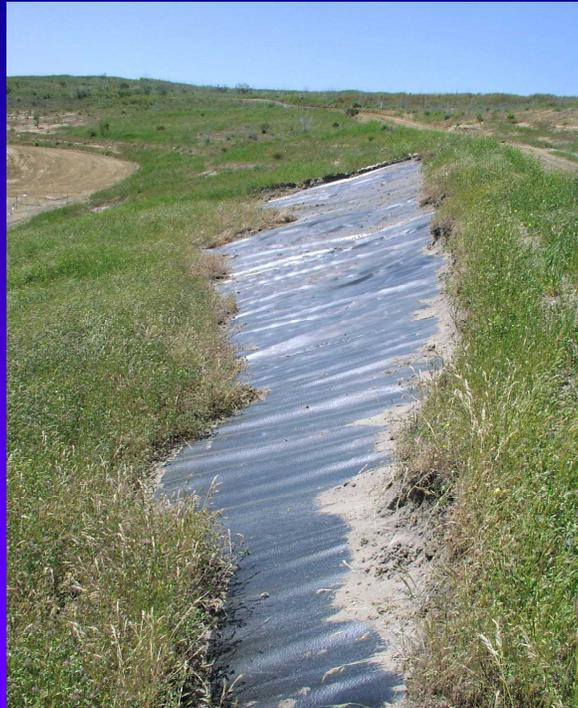
**Figure 4-** Localized failure/slumping of operations layer in the Phase 1 expansion unit during April 2003.<sup>31</sup>
