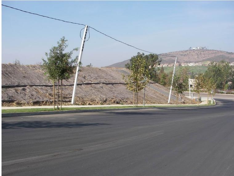
Figure D-3. Use of Netting and Fiber Rolls at San Elijo Hills Construction Site, Northstar Way, Carlsbad Watershed.
