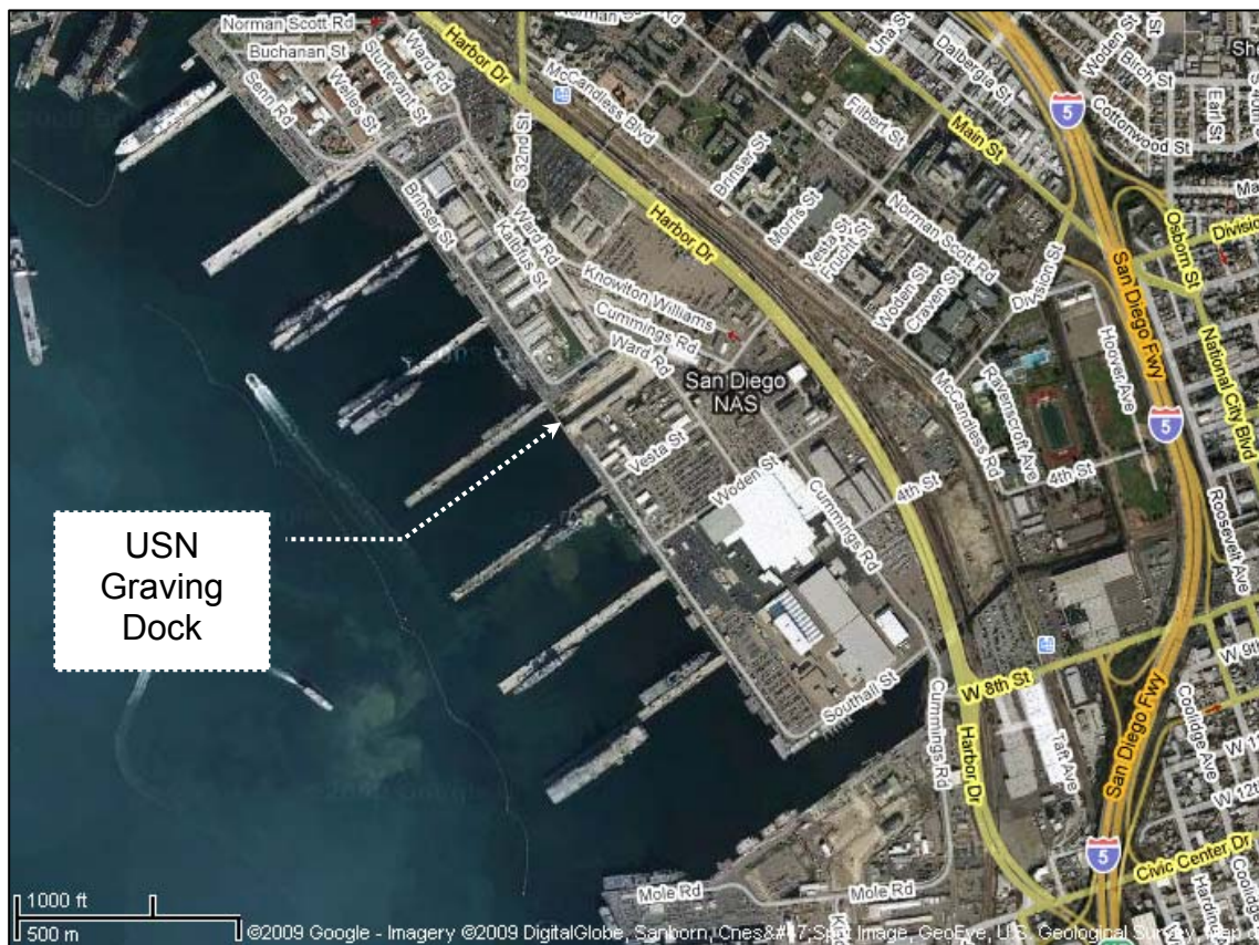
Figure B-8. USN Graving Dock at NBSD
