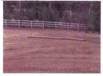
Observation: The straw wattles were not properly keyed into the ground, and they need to be staked in to prevent failure during a rain event. RWQCB staff provided Dr. Moritz's counsel with a CASQA BMP fact sheet after the inspection. With the amount of disturbed soil on site, the implementation of only three straw wattles on site does not seem to provide effective coverage of the entire disturbed area, should soil become mobilized during a rain event.
