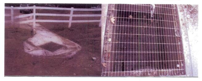
Observation: The inlet that was constructed to convey runoff from Jerome Drive to drainage pipe installed across the property lacked sediment control BMPs to prevent the discharge of sediment into the inlet. Either gravel bags or straw wattles placed around the perimeter could alleviate this problem. The inlet also has standing water in the bottom of the inlet which could pose vector problems.
