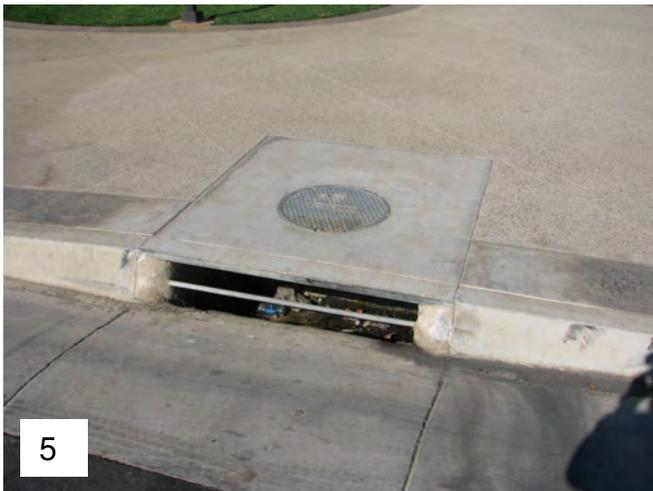
Photos 1 to 5 – Photos of the four inlet drains in the parking lot. None have inlet filters or other treatment devices.
