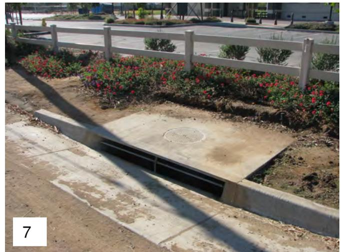
Photos 6 and 7 – Photos show the storm drain inlet along Palomar Street next to the parking lot. This inlet also appeared to not have any inlet filters or other treatment devices.
