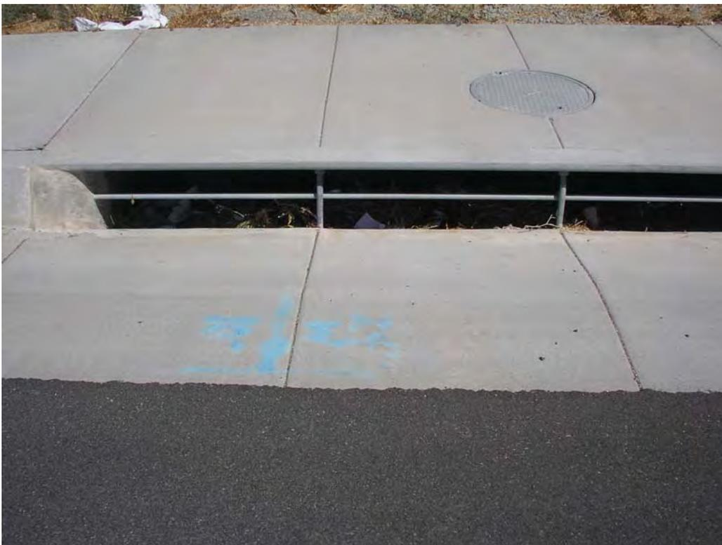
Figure 12. Storm Drain Inlet—no signage
