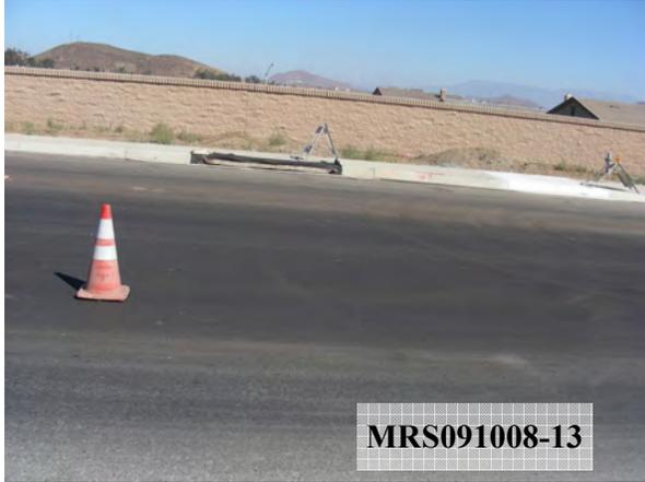
North side of Scott Rd storm drain with silt cloth and straw waddle. Plan to supplement with gravel filled bags to provide added protection
