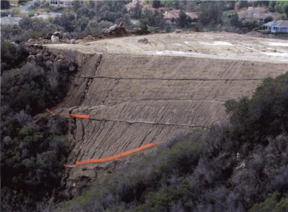
Photo 19: Failed BMPs on slopes; silt fence does not follow contour.
