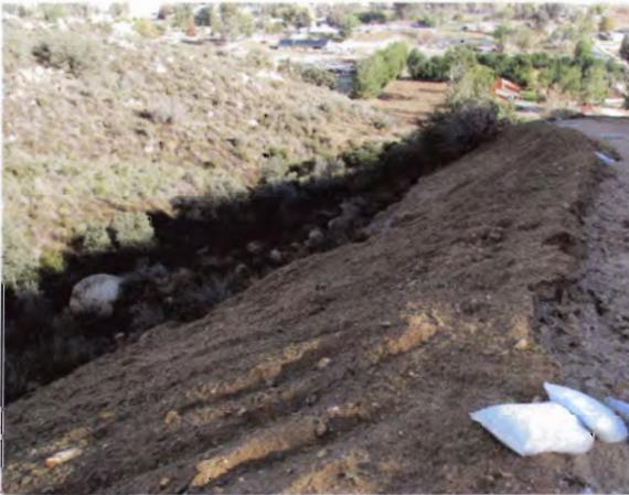
Photo 08: Outside slope not stabilized, discharge of fill (rocks, boulders, and vegetation) in waterway
