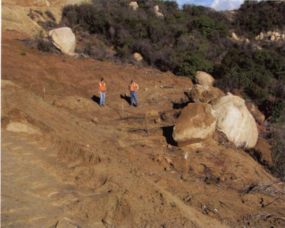
Photo 13: This area lacks erosion and sediment controls as significant quantities of dirt is placed alongside a natural waterway.
