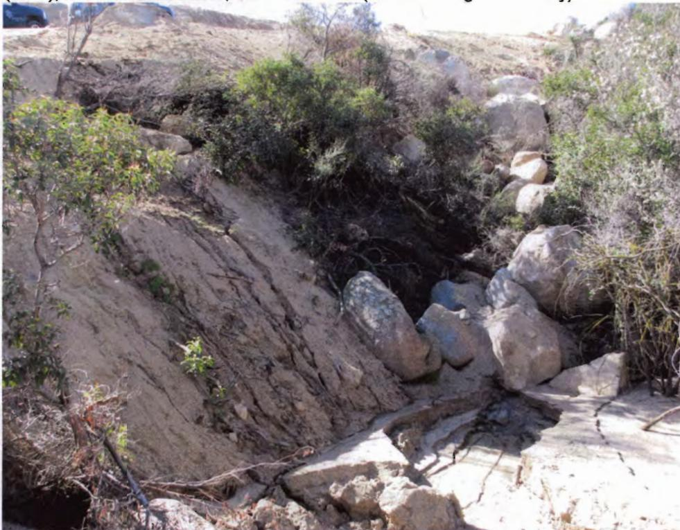
Photo 11: Rocks and boulders were sidescaped into the natural drainage area along the fire road. The caked sediment is evidence of flow blockage.
