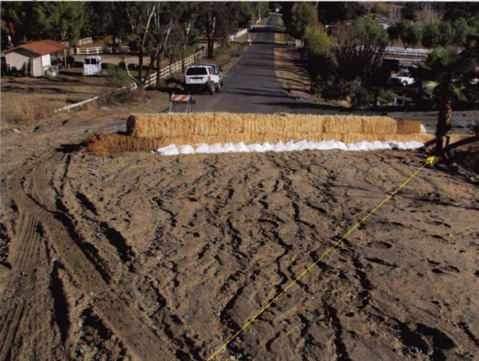
Photo 04: Looking east along Clairemont Street-site entrance/exit lacks tracking control. Insert shows point of sediment discharge under road crossing.
