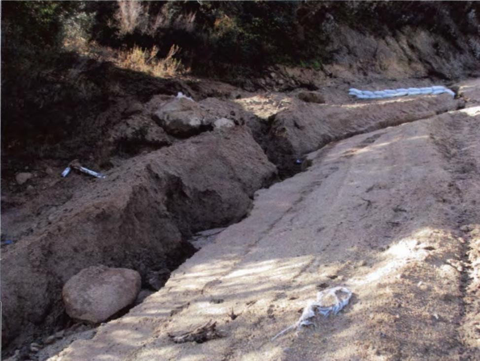
Photo 06: Erosion gullies along the fire road leading to Fairway Hills Estates site.
