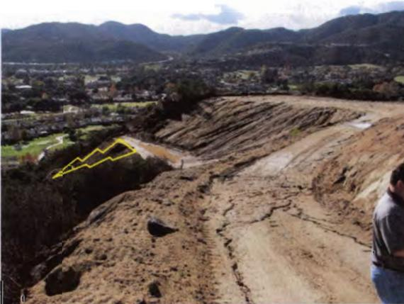
Photo 09: Unstabilized slopes and access road, breached sediment basin allowed sediment discharge (insert) in waterway
