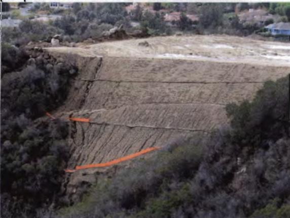
Photo 21: Close-up of erosion rills on slope shown in photo 20
