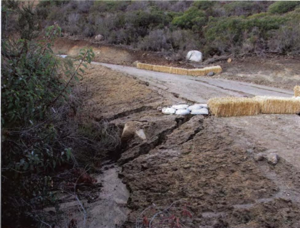
Photo 07: Inappropriate BMPs (hay bales and sand bags) are unable to contain and abate the high, concentrated flows causing rills and gullies.
