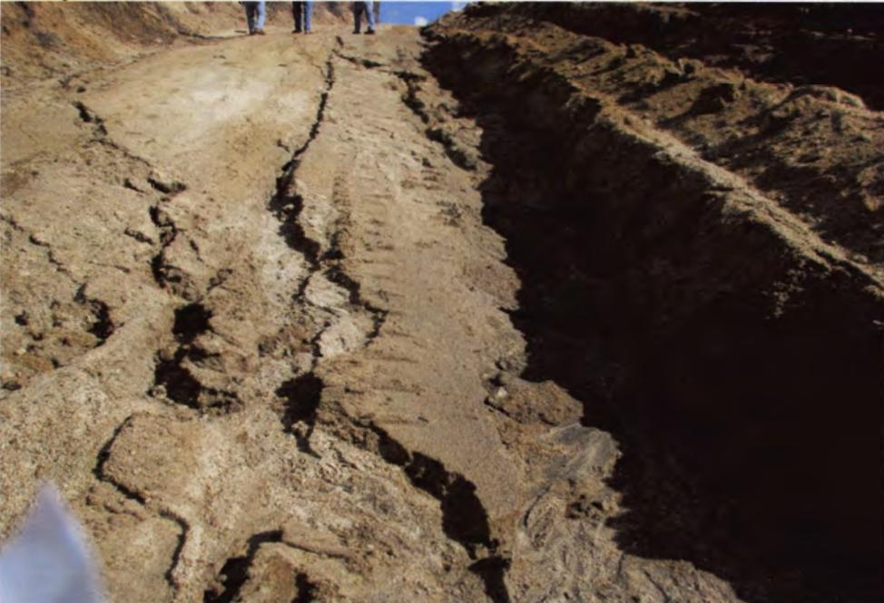
Photo 18: Road leading to basin is heavily eroded. The slopes along the roads are not stabilized to prevent erosion.
