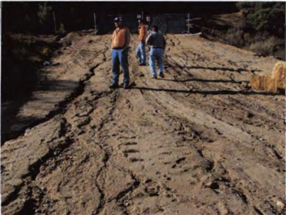
Photo 02: Shows fire-road with significant erosion at site entrance
