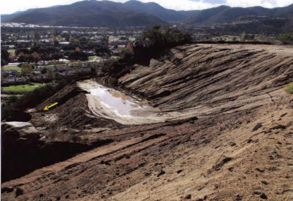
Photo 12: Failed sediment basin is unable to capture sediment-laden runoff from surrounding building pad.
