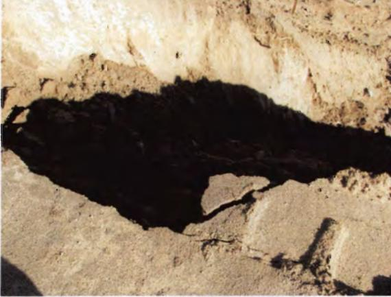
Photo 10: Failed slope along access road
