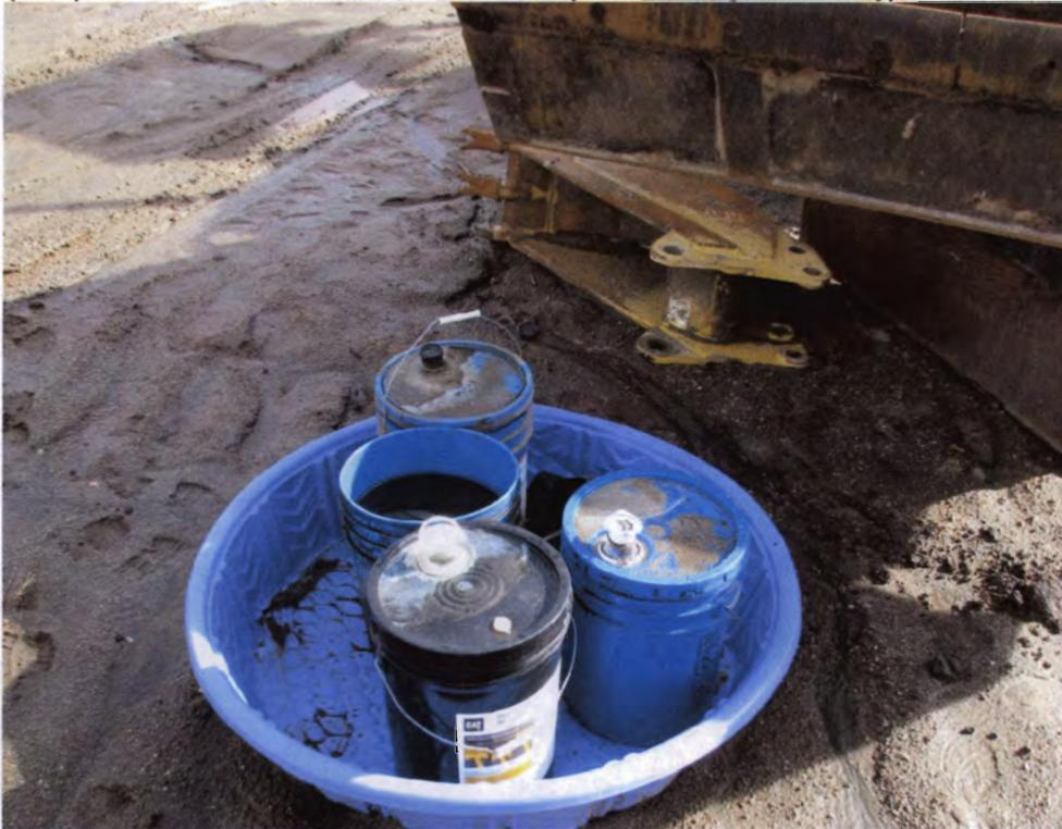
Photo 27: No BMPs to minimize exposure of mechanical construction wastes to stormwater or to potential accidents.
