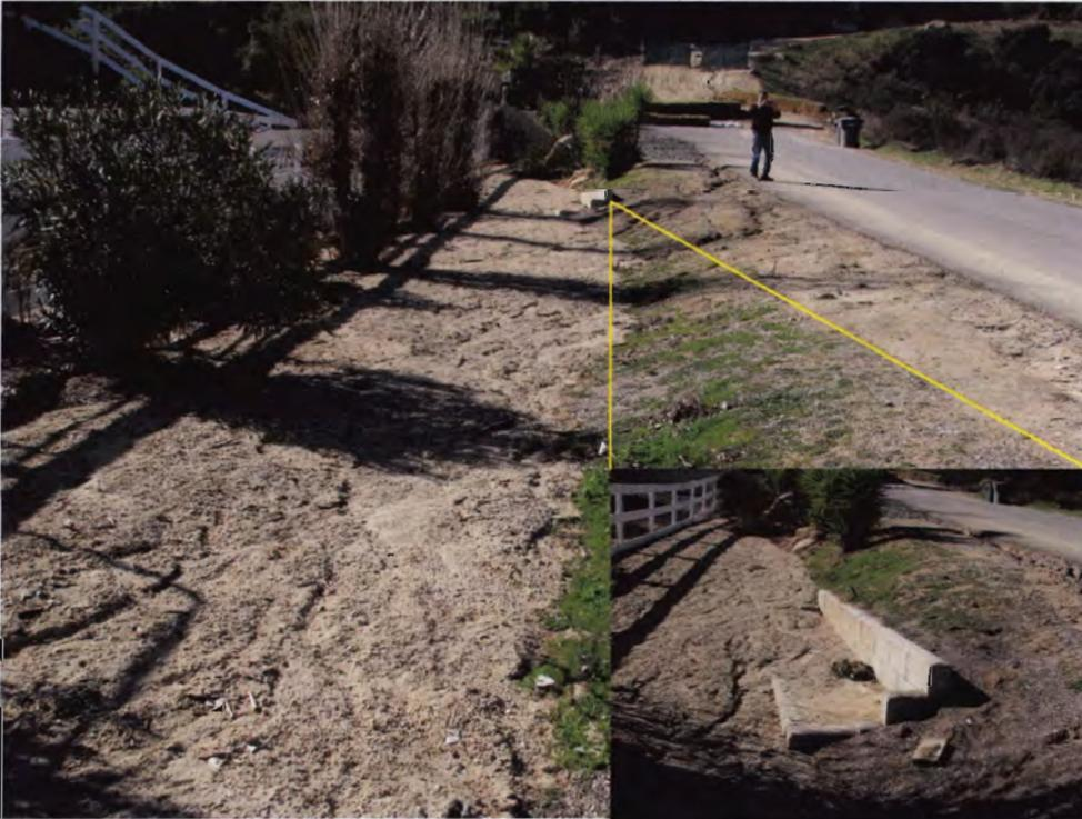
Photo 02: Sediment and silt are deposited along brow ditch along Claremont Street. Insert shows utility vault covered with sediment and silt.
