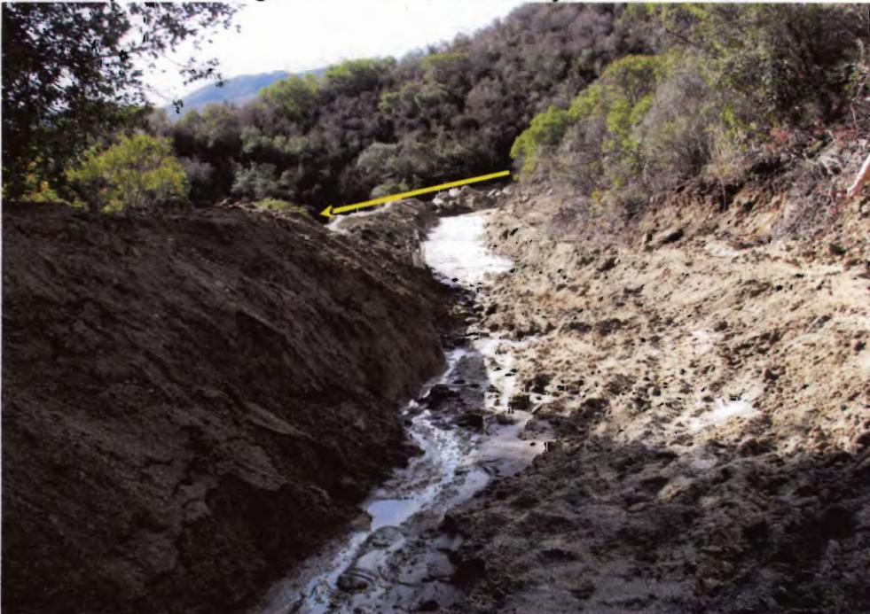
Photo 14: This sediment basin captures runoff from the fire road and upgradient construction activities. The basin is built directly in a natural waterway, shown in background.
