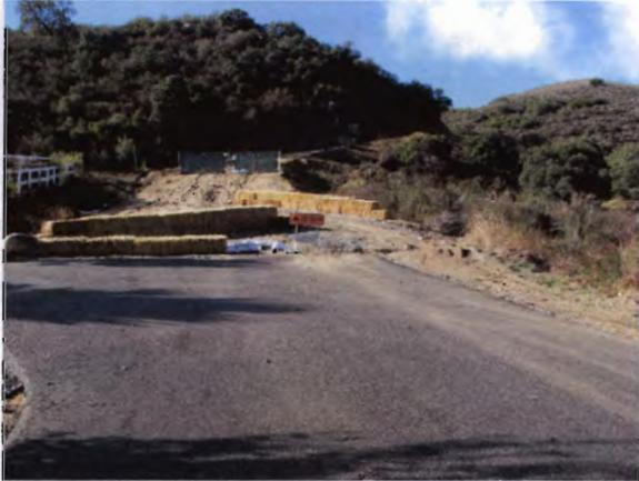
Photo 01: Site entrance at Claremont Street shows inadequate BMP to prevent erosion
