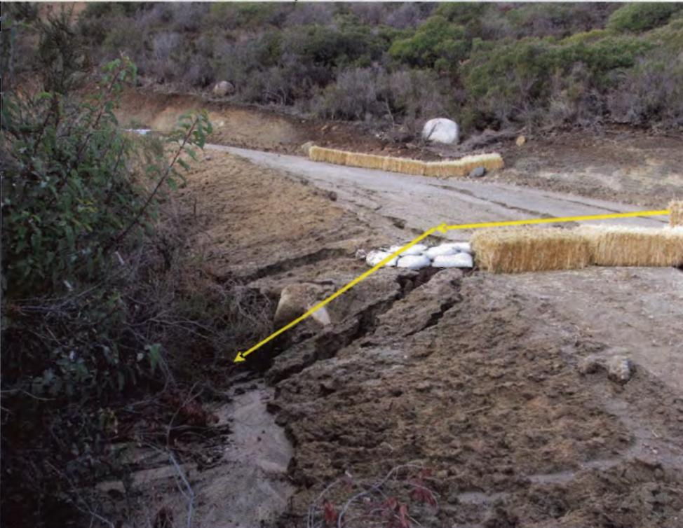
Photo 20: The road was constructed (w/o proper permit) directly across a natural waterway. Erosion effects can be seen across the road.
