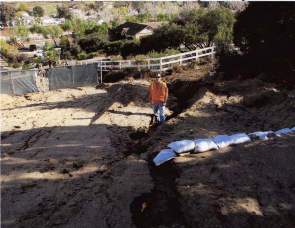
Photo 08: Erosion gullies were caused by high, concentrated storm water flows and failed BMPs.
