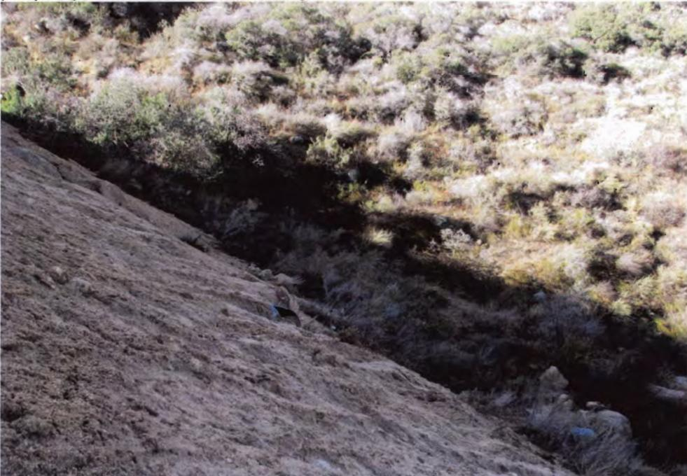
Photo 10: Evidence of recent grading of the fire road shows graded dirt was sidescaped down embankment towards natural waterway.
