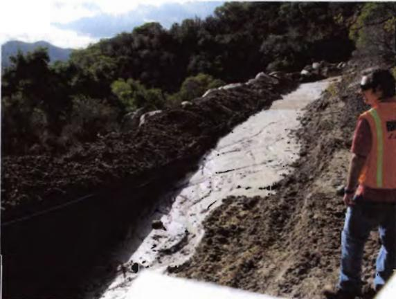
Photo 17: Shows significant sediment and silt in sediment basin
