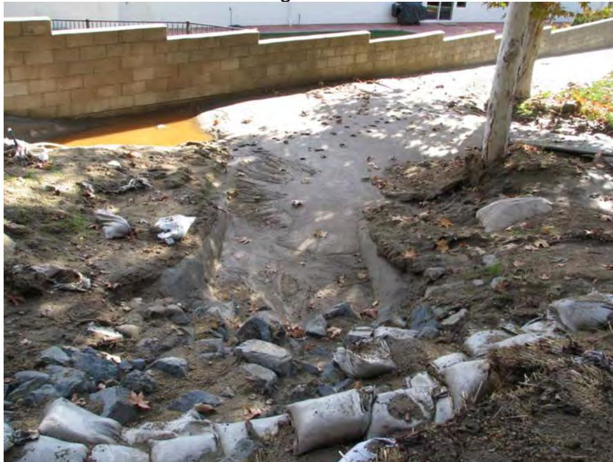
**Figure 8.** Photo of sediment discharge to MS4 tributary to Murrieta Creek.(IMG\_0273.JPG taken by San Diego Water Board on December 23, 2008)
