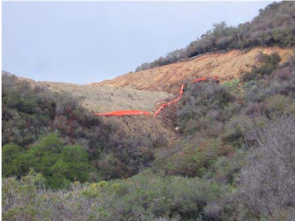
**Figure 6.** Photo of failed silt fence, and inadequately protected large graded slopes with numerous erosion rills. (Photo IMG\_010.JPG taken by County of Riverside on January 29, 2008.)
