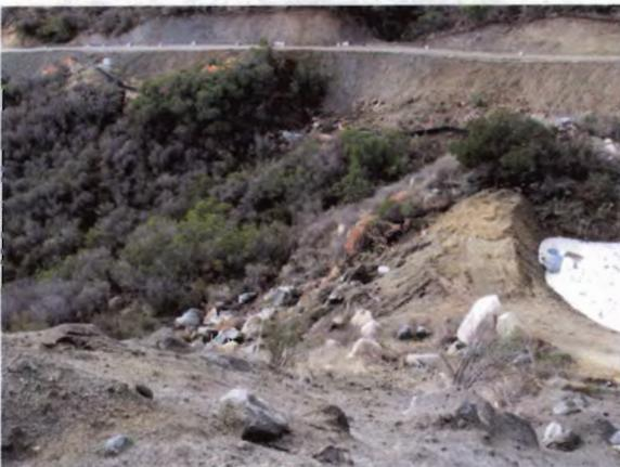
Photo 24: Construction wastes or fill (rocks, trash, and debris) deposited in waterway downgradient from the sediment basin. This sediment basin connects to the sediment basin shown in photos 17 and 18
