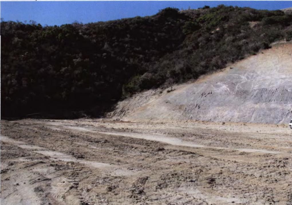
Photo 26: No slope stabilization and building pad is not covered or stabilized.
