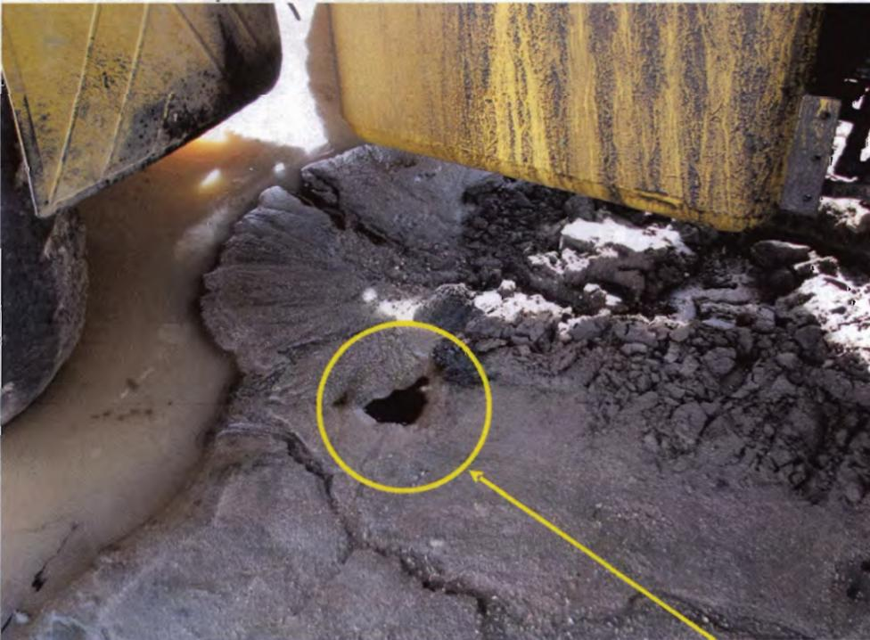
Photo 28: Construction vehicles are improperly stored with no drip pans to capture spill or leaks.
