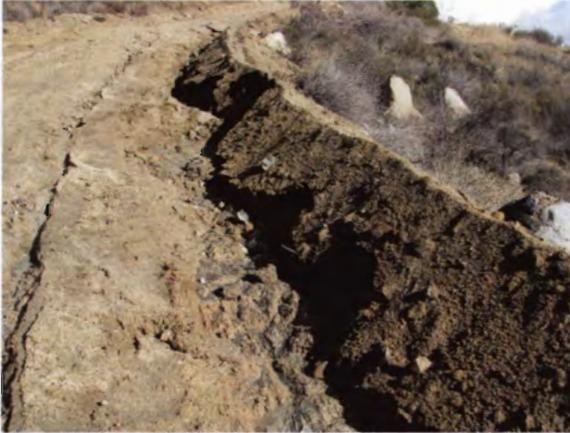
Photo 13: Shows severe erosion along access road leading to middle basin
