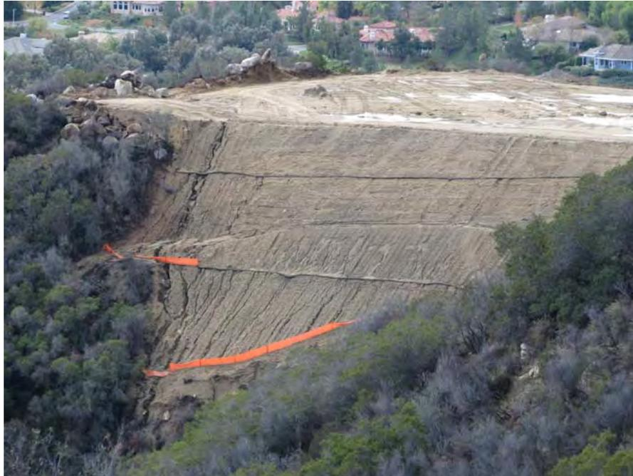
**Figure 10.** Photo of failed silt fences and erosion rills from 38175 Via Vista Grande. (IMG\_077.JPG taken by San Diego Water Board on December 16, 2008.)
