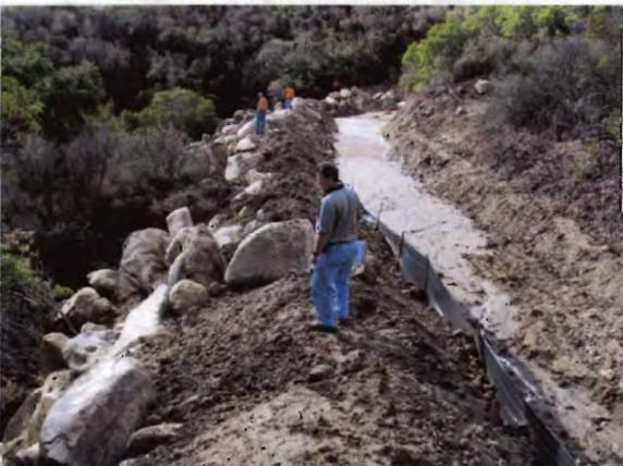
Photo 18: Construction wastes or fill (boulders, rocks, shrubs) sidescaped in waterway
