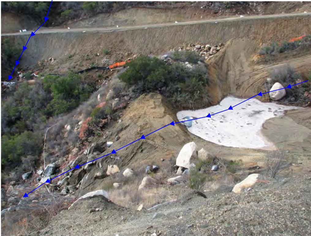
**Figure 1.** Photo of construction wastes/fill (sediment, silt, rocks, and boulders) discharged and detention basin construction in waters of the state. (IMG-081.JPG taken by San Diego Water Board during December 16, 2008 inspection.)
