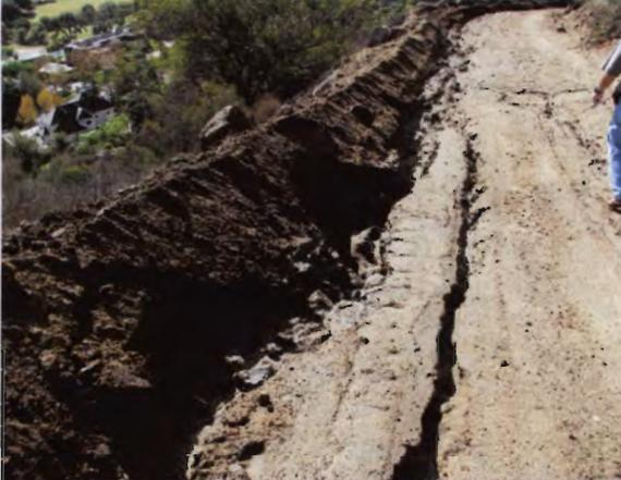
Photo 14: Looking downhill along access road shows erosion gullies
