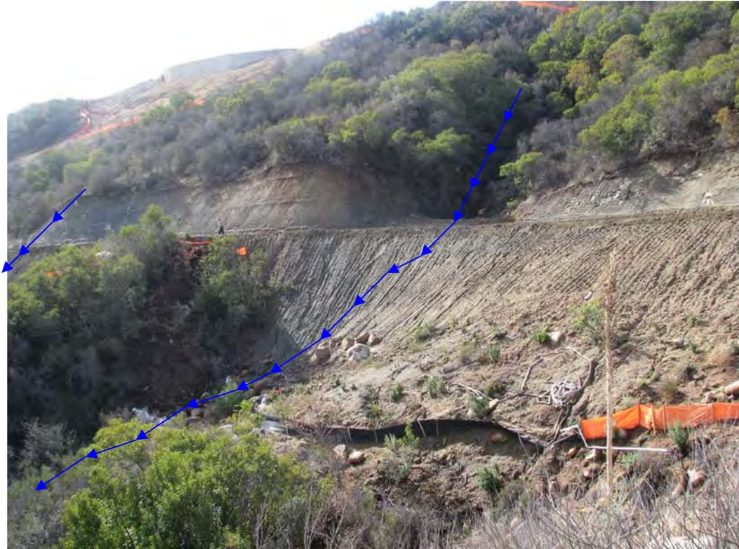
**Figure 3.** Photo of construction wastes/fill (sediment, silt, rocks and boulders) discharged into waters of the state from construction of the access road. (IMG\_0293.JPG taken by San Diego Water Board during December 23, 2008 inspection.)
