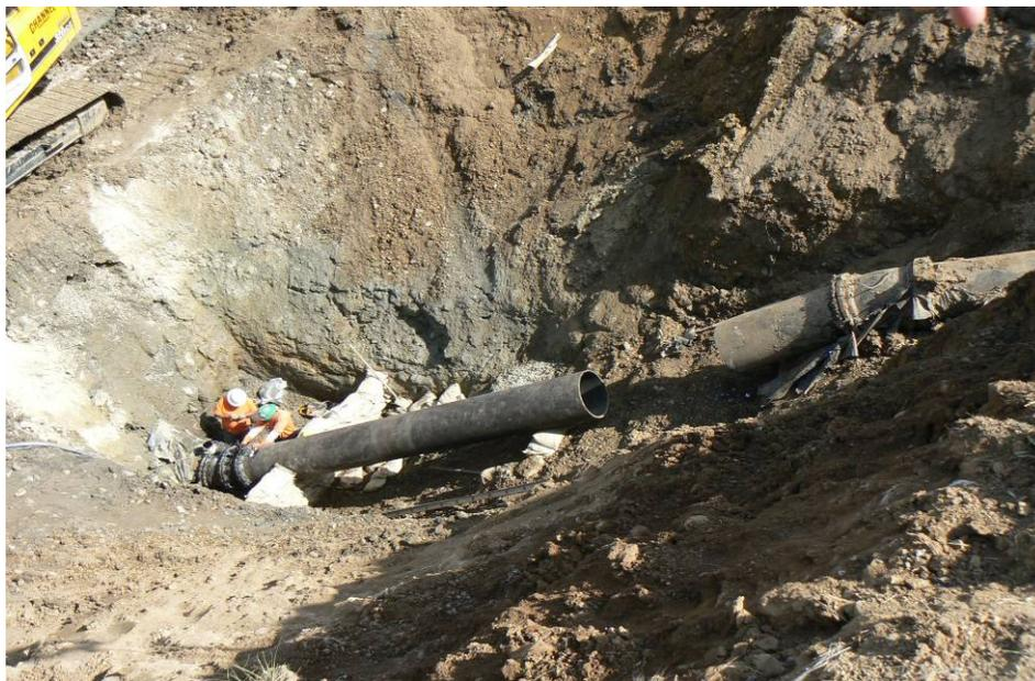
Figure 8. Force main rupture repair work on March 26, 2010
