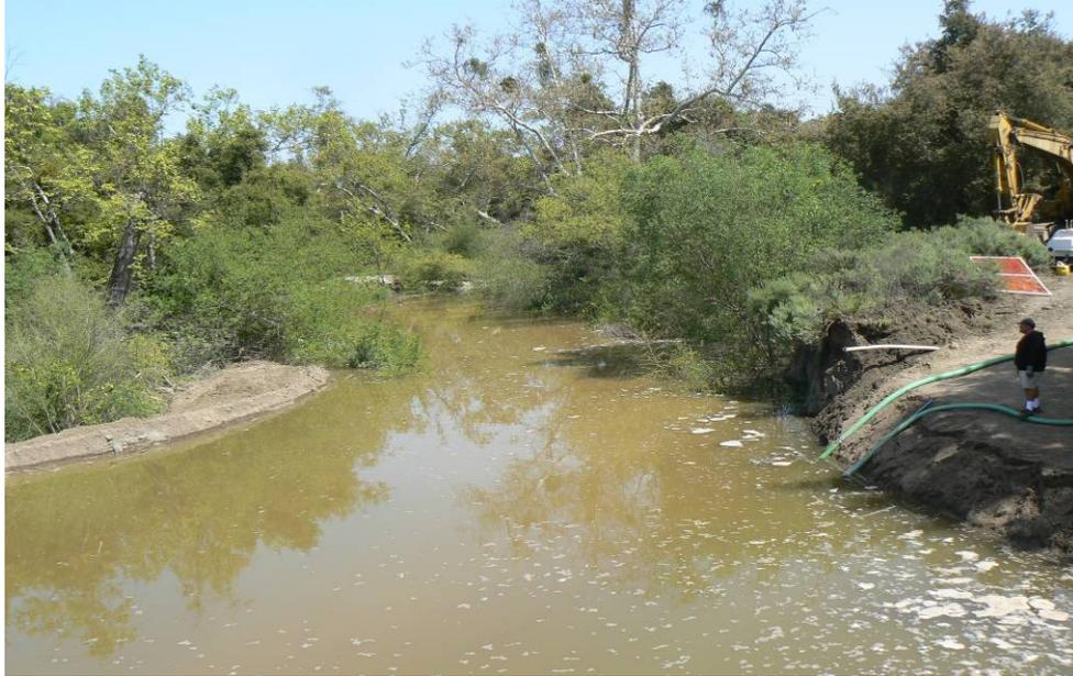
Figure 6. Sewage backed up in Tijeras Creek north of containment berm
