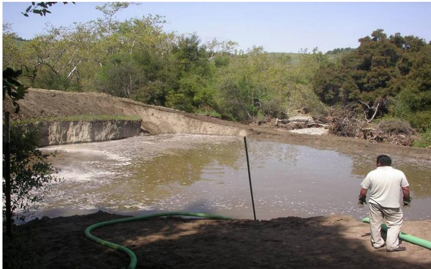
Figure 4. Earthen berm construction on March 25, 2010 to contain raw sewage within Tijeras Creek
