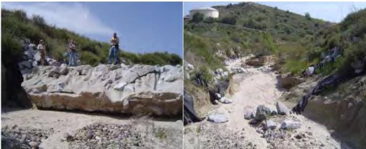
**Figure 3-2. Undermining of grade control and erosion of banks downstream of structures intended to stabilize a particular stream reach. Left photo is looking upstream at drop structure; right photo is looking downstream from the drop structure.**
