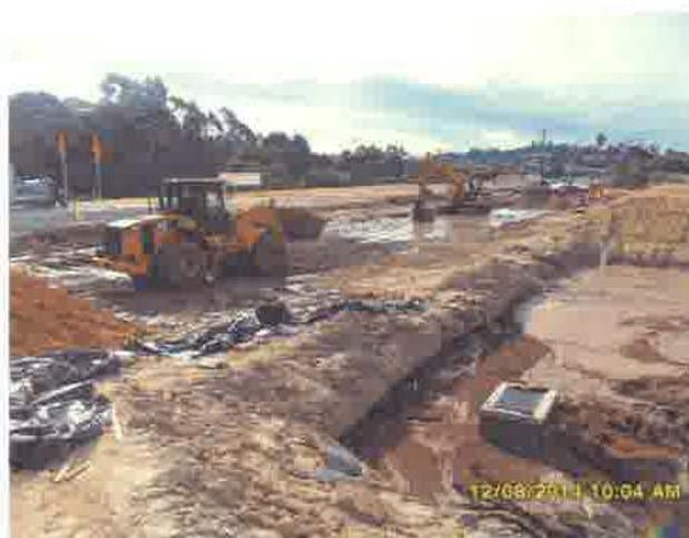
Lack of erosion controls in inactive areas.
