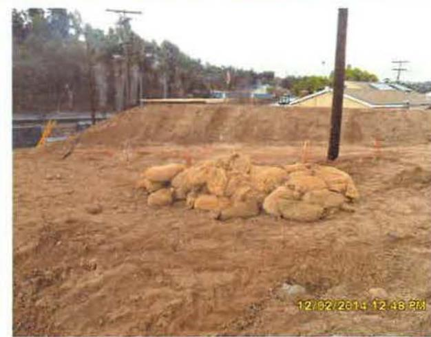
Lack of erosion control BMPs on inactive areas.
