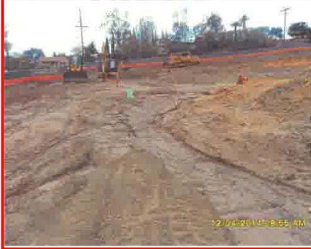
Although stockpile is partially covered it lacks perimeter containment.
