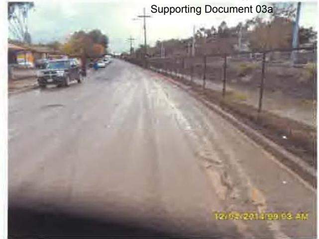
Lack of erosion control in inactive areas.
