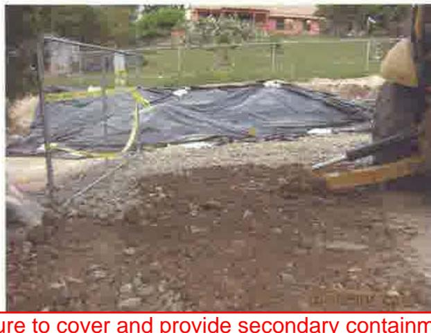
Failure to cover and provide secondary containment.
