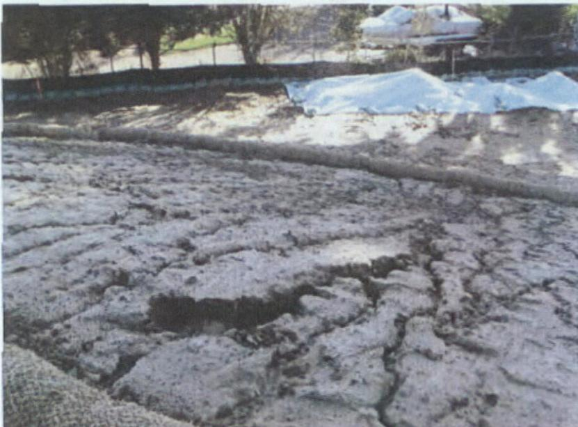
**Photo 5: Significant erosion rills leading toward property boundary along Carretta Way.**
