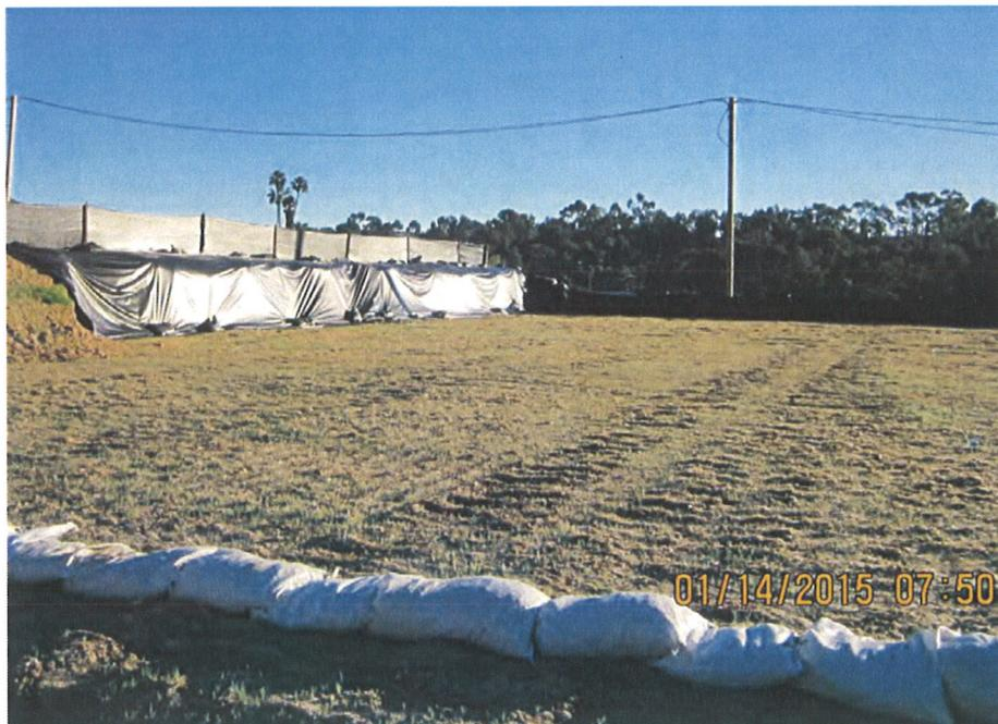
Photo 6 Sidewall protected with plastic sheeting.
