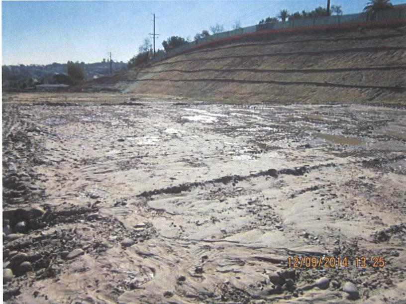
Photo 1. Lot lacking erosion control BMPs
