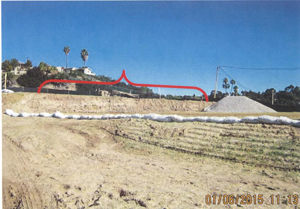
Photo 5. Sidewall without adequate erosion control
