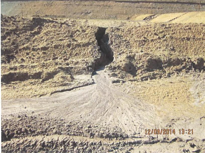
Photo 3. Evidence of erosion at edge of a lot
