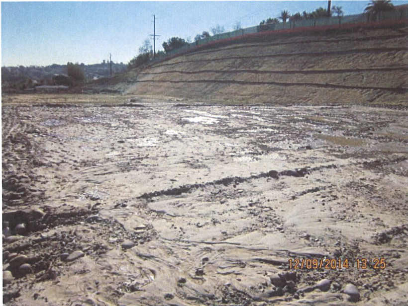
Photo 1. Lot lacking erosion control BMPs
