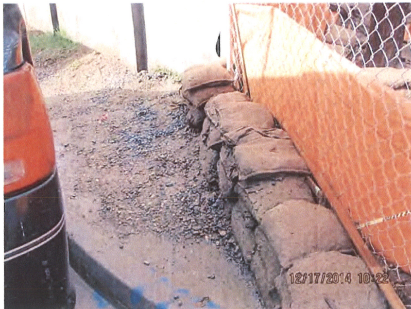
Photo 2. Evidence of sediment discharge at Akins entrance/exit
