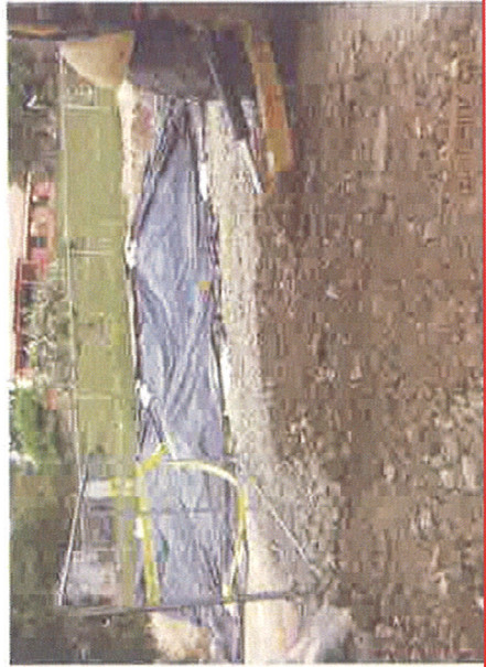
Failure to cover and provide secondary containment.
