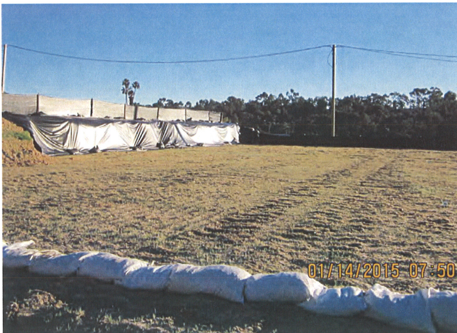
Photo 6 Sidewall protected with plastic sheeting.
