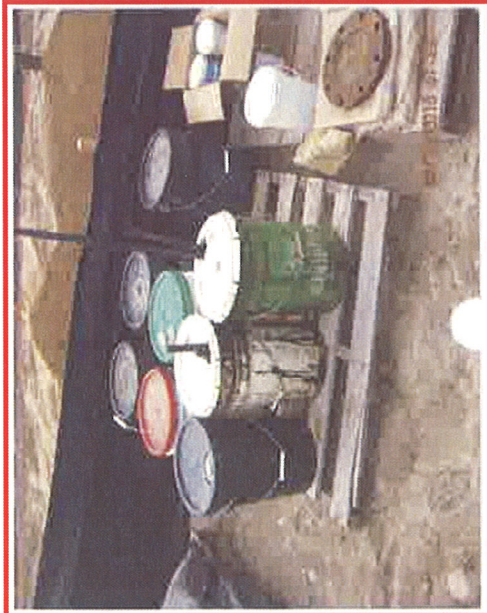
Failure to cover and provide secondary containment.
