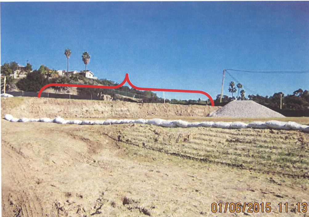
Photo 5. Sidewall without adequate erosion control
