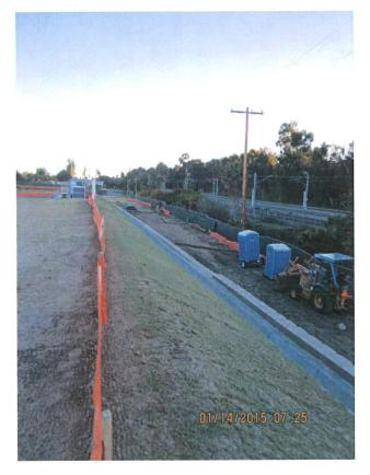
Photo 4. Rills filled in, area re-hydroseeded, silt fence added to perimeter of lot.
