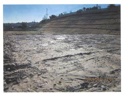
Photo 1. Lot lacking erosion control BMPs
