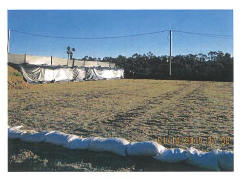
Photo 6Sidewall protected with plastic sheeting.
