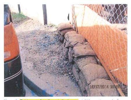
Photo 2. Evidence of sediment discharge at Akins entrance/exit
