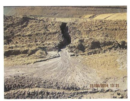
Photo 3. Evidence of erosion at edge of a lot
