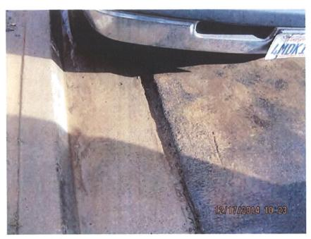
Photo 3. Sediment accumulation along Akins curb gutter, downstream of Akins entrance/exit
