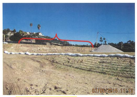
Photo 5. Sidewall without adequate erosion control
