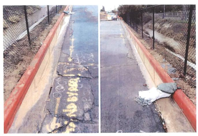
Photos 2 &3. Ponded Water at First Set of Gravel Bags Downstream of Akins Avenue Entrance/Exit (Looking downstream and upstream, respectively)
