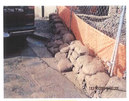
Photo 1. Evidence of sediment discharge at Akins entrance/exit
