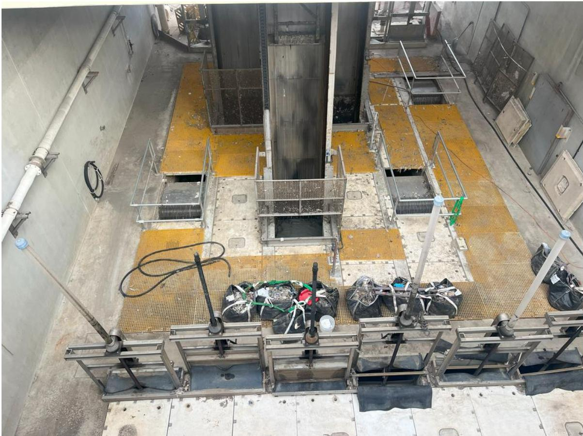
Figure 2: Influent Channels and Bar Screens. (MC 01/10/2024)
