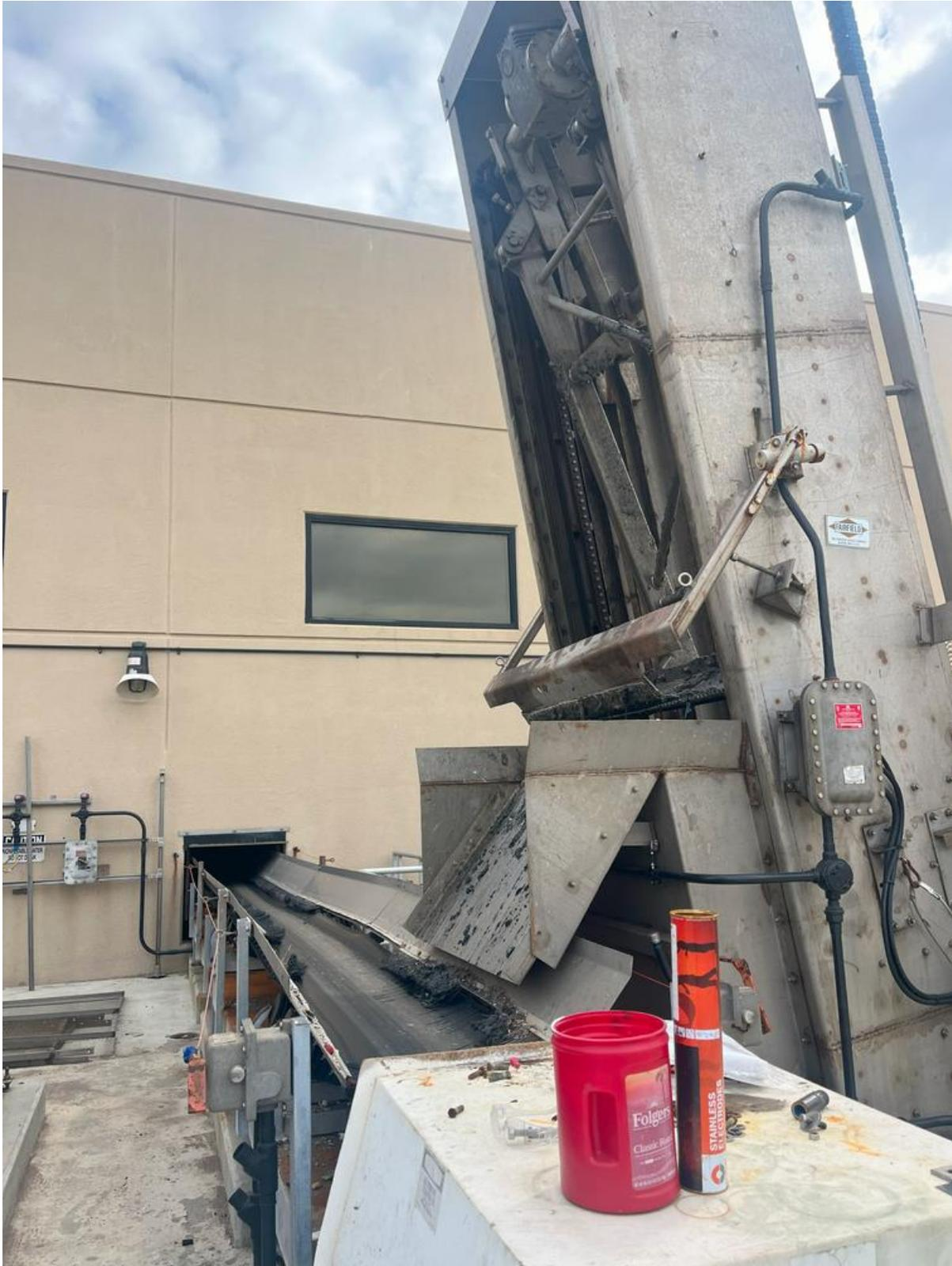
*Figure 3: Automatic Bar Screen: This is the top end that discharges to a conveyor belt for collection of the debris. (MC 01/10/2024)*
