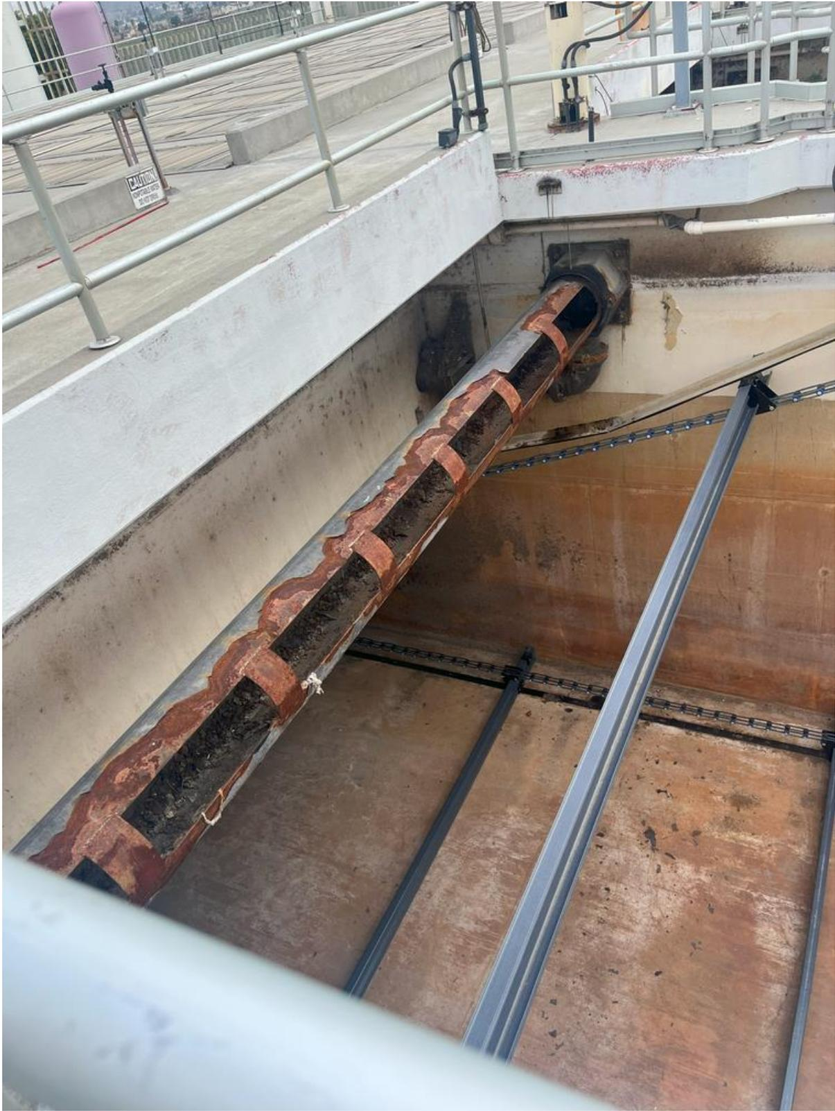
Figure 8: Existing Skimmer Trough at PST No. 5. (MC 01/10/2024)
