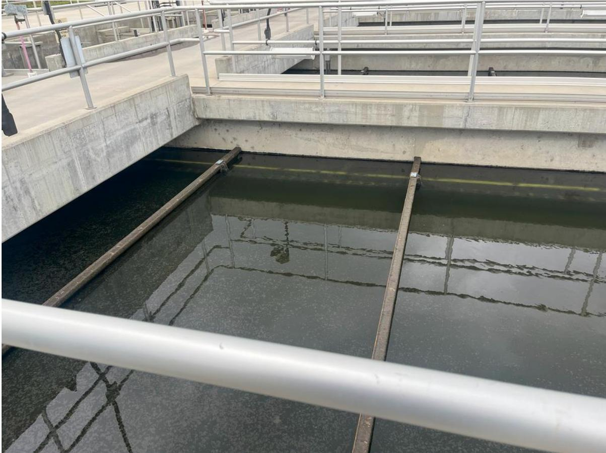
Figure 12: Secondary Settling Tank. (MC 01/10/2024)
