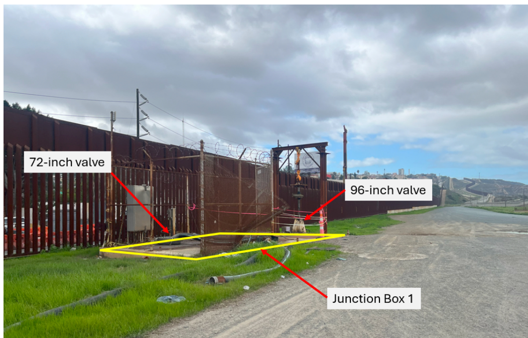
Figure 4: Junction Box 1. (MC 01/10/2024)
