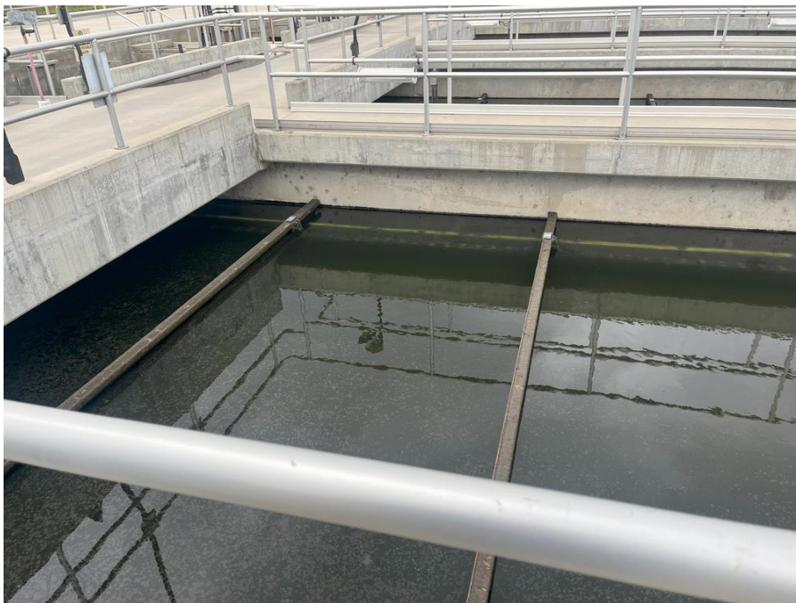
Figure 8: Secondary settling tank. (MC 01/10/2024)
