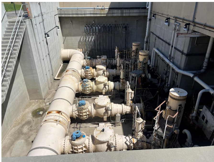
Figure 5: Influent pumps. (MC 04/03/2024)
