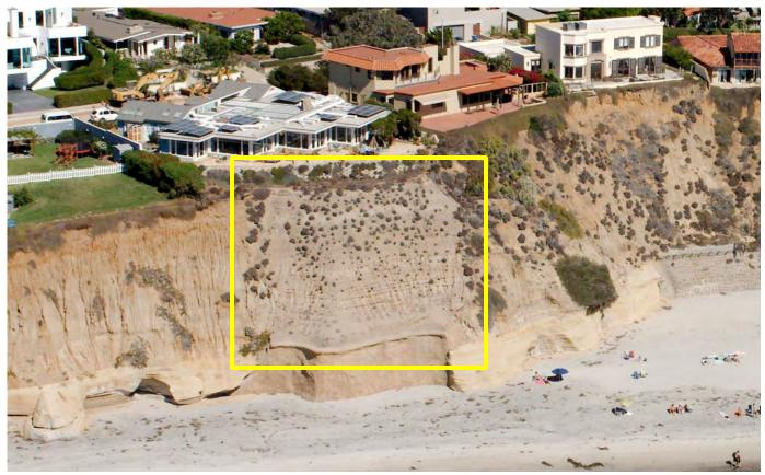
Proposed installation of hydroseed and container plantings on the existing geogrid slope
