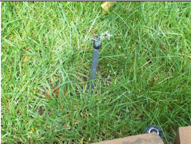
Photo 7: Single sprinkler head for entire valve. Cap off sprinkler or use the valve for another area.
