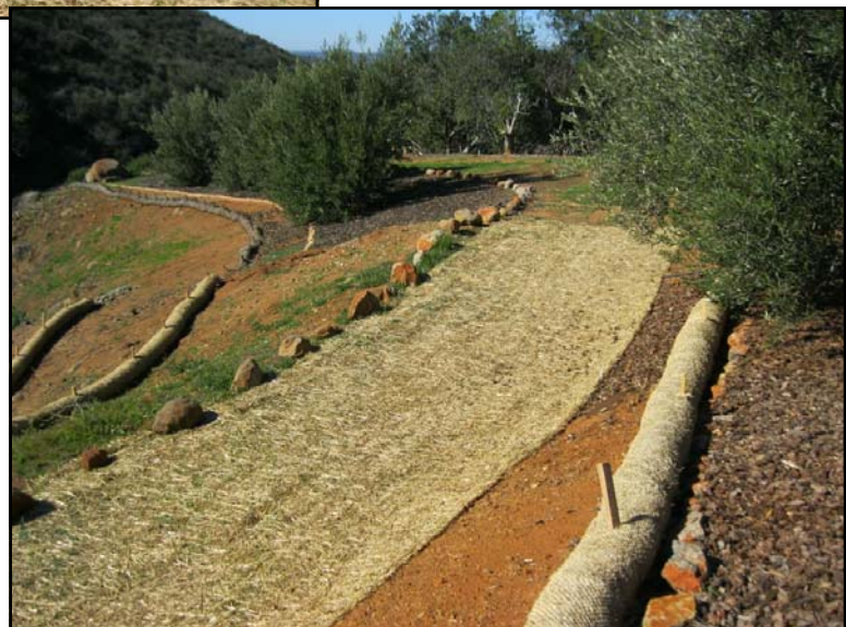
Left Photo: The access road has been protected with a straw mat. The uphill access road slope (on the right) has been protected with a straw wattle. An extension pipe from the outlet of the roof runoff structure has been extended and it now outlets into a drainage creek and natural rock dissipater. The BMPs implemented were heavy use area protection, straw wattle and underground outlet and dissipater. Photo taken during follow-up site visit.
