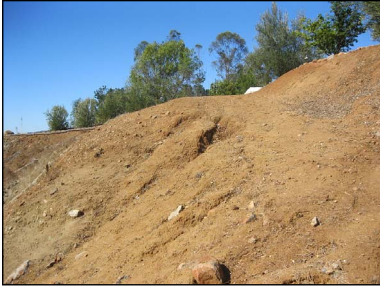
Left Photo: Photo taken looking up hill at a dirt access road (on the right), which is experiencing sheet, rill and rut erosion from stormwater runoff and erosion on the outboard slope (on the left) caused by the outlet location of a roof runoff structure (gutter) pipe. Photo taken during initial site visit.
