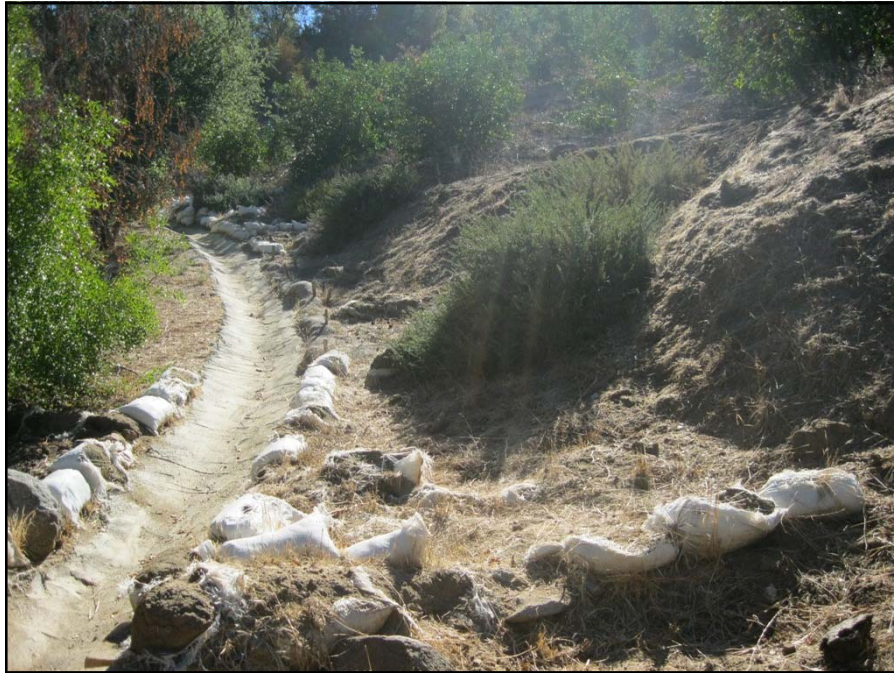
Above Photo: A slope experiencing erosion and sediment loss, with the sediment flowing into the lined waterway which empties into Rainbow Creek. The degraded sand bags were the property owners' attempt to control the sediment lost from the slope and the citrus grove directly uphill. Photo taken during the initial site visit looking uphill.
