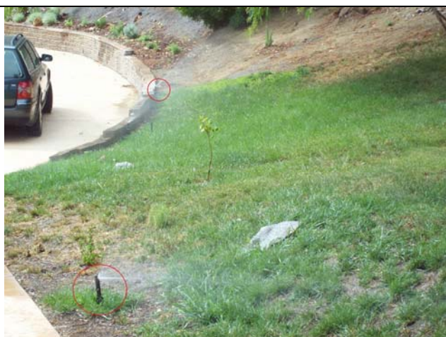
Photo 3: Mixed sprinkler heads on the same valve is never suggested.
