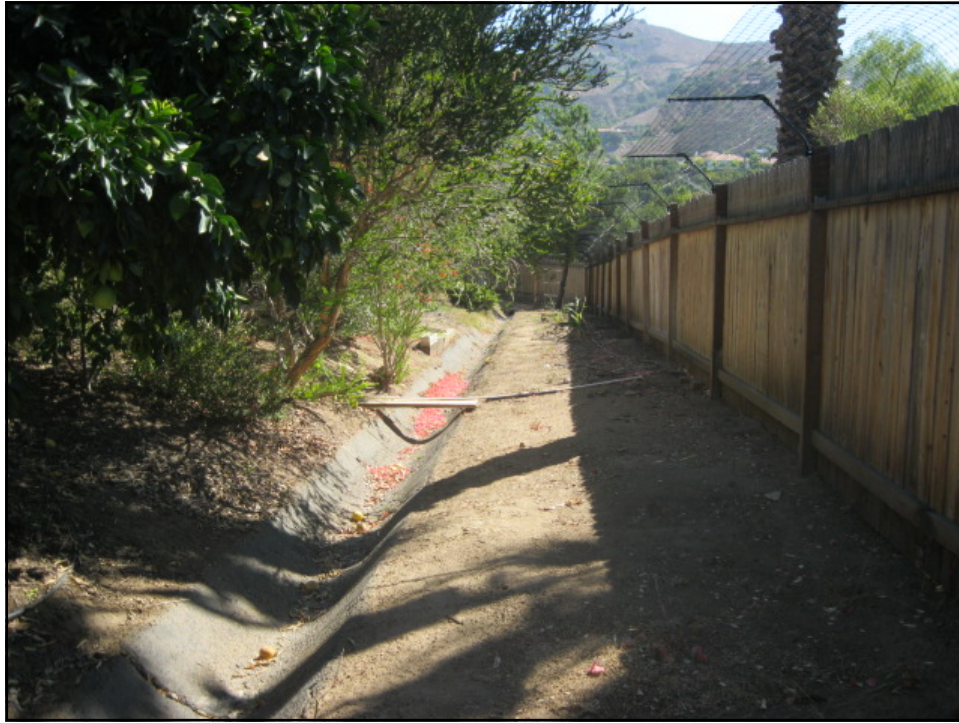
Above Photo: A bare slope experiencing sediment loss, which enters the lined waterway and empties into a tributary of Rainbow Creek that is located directly downstream of the property. Photo taken during the initial site visit.
