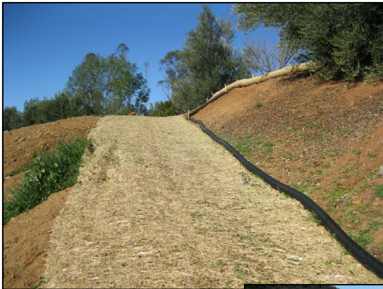
Left Photo: The access road has been protected with a straw mat. The uphill access road slope (on the right) has been protected with a straw wattle. An extension pipe from the outlet of the roof runoff structure has been extended and it now outlets into a drainage creek and natural rock dissipater. The BMPs implemented were heavy use area protection, straw wattle and underground outlet and dissipater. Photo taken during follow-up site visit.
