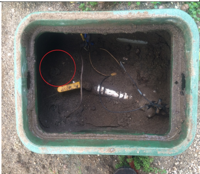
Photo 3: An inline pressure regulator can be installed after the isolation ball valve.
