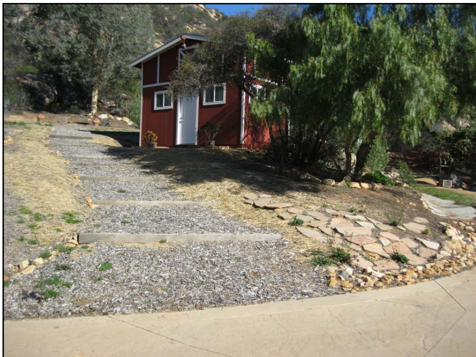
Below Photo: The exposed and vulnerable area has been protected with wood chips and straw to help prevent and control sediment loss. The BMP implemented was heavy use area protection. Photo taken during the follow-up site visit at bottom of stairs looking up towards the top of the stairs.
