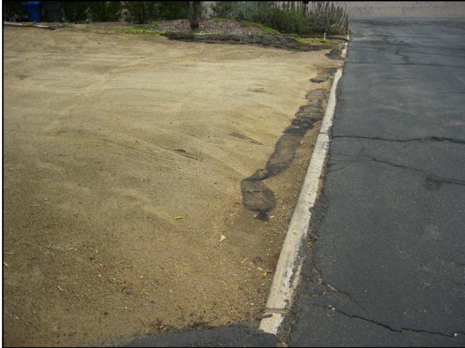
Above Photo: Heavy use area (dirt parking area) experiencing sheet, rill and rut erosion and sediment loss. The owner has attempted to keep the sediment on the parking area and off the driveway with straw wattles (now degraded). Photo taken during the initial site.
