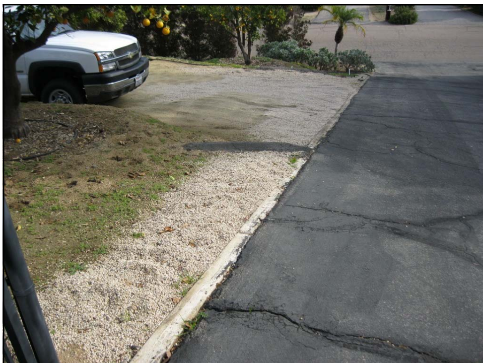
Below Photo: The exposed and vulnerable area has been protected with gravel to help prevent and control sediment loss. The BMPs implemented were heavy use area protection and a lined waterway. Photo taken during the follow-up site visit .
