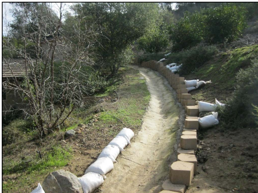
Below Photo: The lined waterway was reinforced and a retaining wall was installed to catch the sediment flowing from the uphill property. Sand bags were also installed to act as silt barriers. The slope was allowed to grow weeds in order to help prevent erosion, as well. The BMPs implemented lined waterway maintenance, retaining wall, silt barriers and critical area planting. Photo taken during the follow-up site visit.
