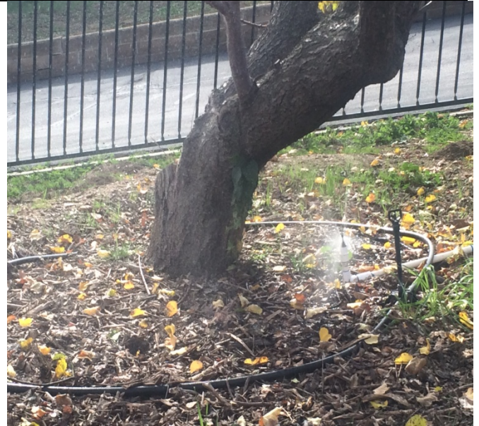
Photo 2: Misting caused by high pressure.
