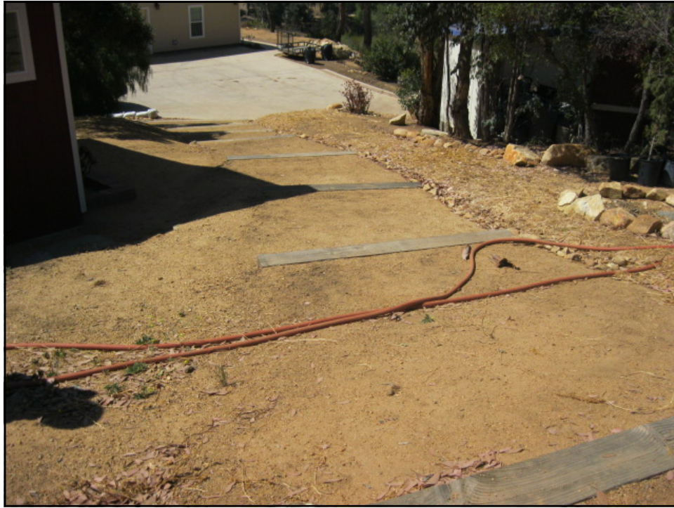
Above Photo: Heavy use area (stairs) experiencing sheet erosion and sediment loss. Photo taken during the initial site visit at top of stairs looking towards bottom of stairs.
