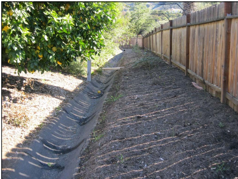
Below Photo: The exposed and vulnerable area has been mulched with wood chips and compost and planted with native, low-water use plants to help prevent and control sediment loss. The BMPs implemented were mulching and critical area planting. Photo taken during the follow-up site visit.
