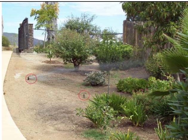
Photo 1: A single rotor sprinkler irrigates this areas (Station #2). The same area also has drip irrigation running to it, but the valve is shut off.
