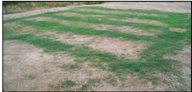
Unusually green vegetation over the leach field is another sign of a septic system that has failed or is about to fail.
