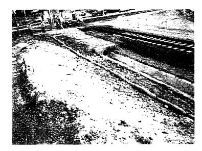
29. No erosion controls on north-facing slope.
