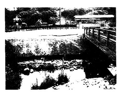
27. Silt fence improperly installed in Loma Alta Creek. No erosion controls on south-facing slope. Same violations noted in NOV No. R9-2007-0208.
