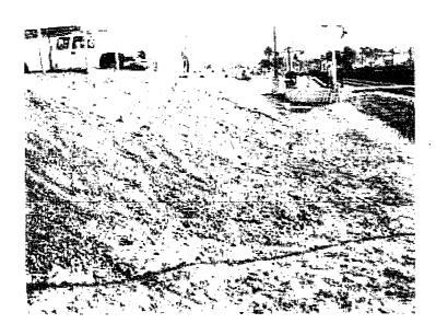
36. No sediment or erosion controls on exposed slopes.
