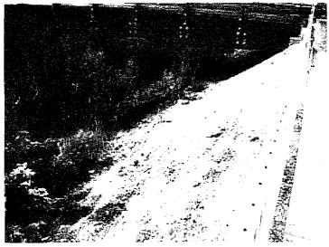
23. No erosion or sediment controls next to bridge on Loma Alta Creek.
