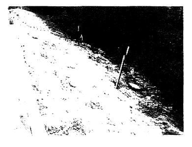
22. No erosion or sediment controls on steep slopes along Loma Alta Creek.
