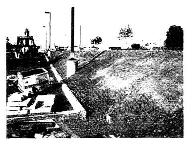
35. No sediment or erosion controls on slopes surrounding the parking lot.
