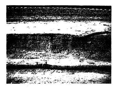
7. Inadequately maintained fiber rolls resulting in erosive rills.
