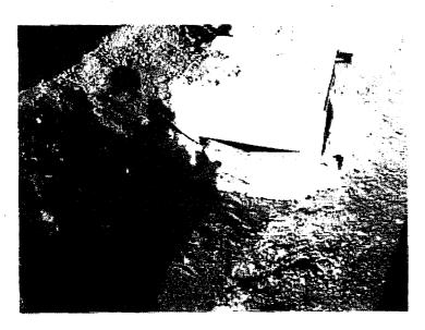
39. Gravel bags not stacked high enough to adequately protect drain inlet. No erosion protection in earthen channel.
