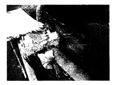
5. Silt fence flattened by construction debris above head wall of storm drain inlet.
