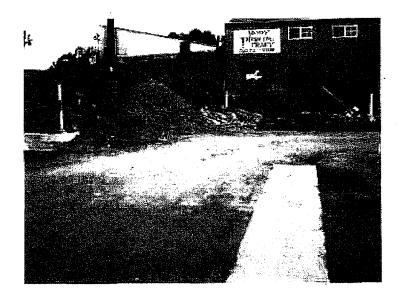
10. Sediment tracking on pavement and soil stockpile without erosion and sediment controls.
