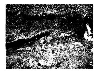
4. Fiber rolls on slopes out of place due to not being adequately staked in and trenched in.
