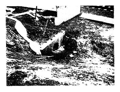
12. Inadequate inlet protection in an area with unstabilized slopes.
