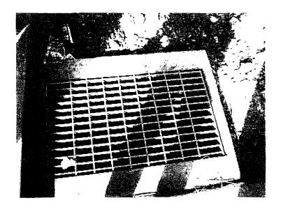
31. No inlet protection in area still under construction.
