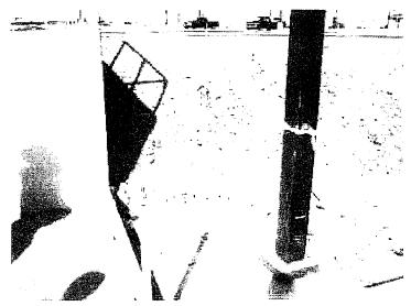
32. No sediment or erosion controls in area above storm drain inlet. No inlet protection.
