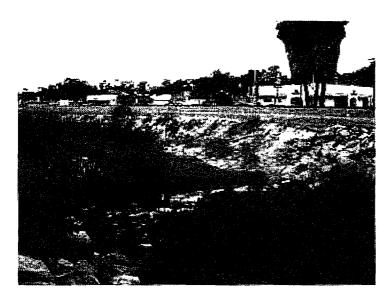
17. No erosion or sediment controls on slopes.
