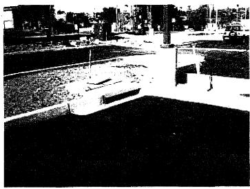
41. Storm drain lacks inlet protection. Parking lot still susceptible to sediment flows.
