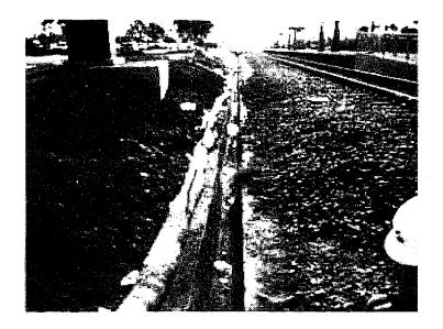
1. Drainage ditch with a significant amount of trash and sediment. No erosion controls on slope.
