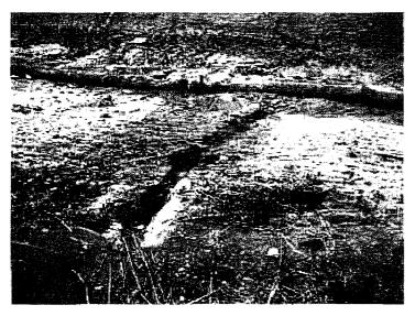
8. Gully formed below a storm water outfall – no erosion controls.
