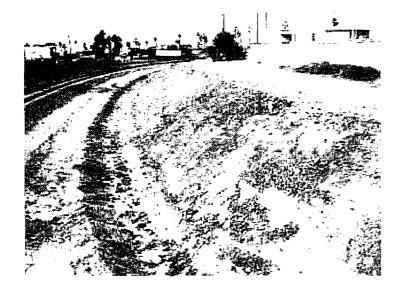
13. Exposed slopes with no erosion controls or sediment controls.
