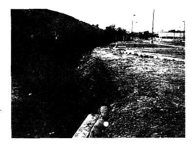
20. Lack of erosion and sediment controls for exposed soil.
