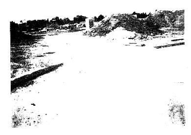
33. No sediment controls to prevent sediment tracking.
