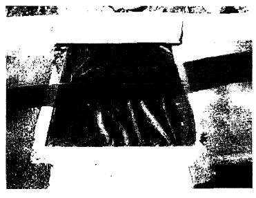
40. Filter fabric needs additional controls to prevent clogging by sediment.
