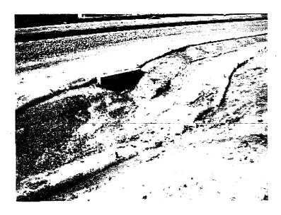
6. No erosion controls on slopes. Inadequate inlet protection. Fiber rolls not trenched in. Dirt channel needs protection.
