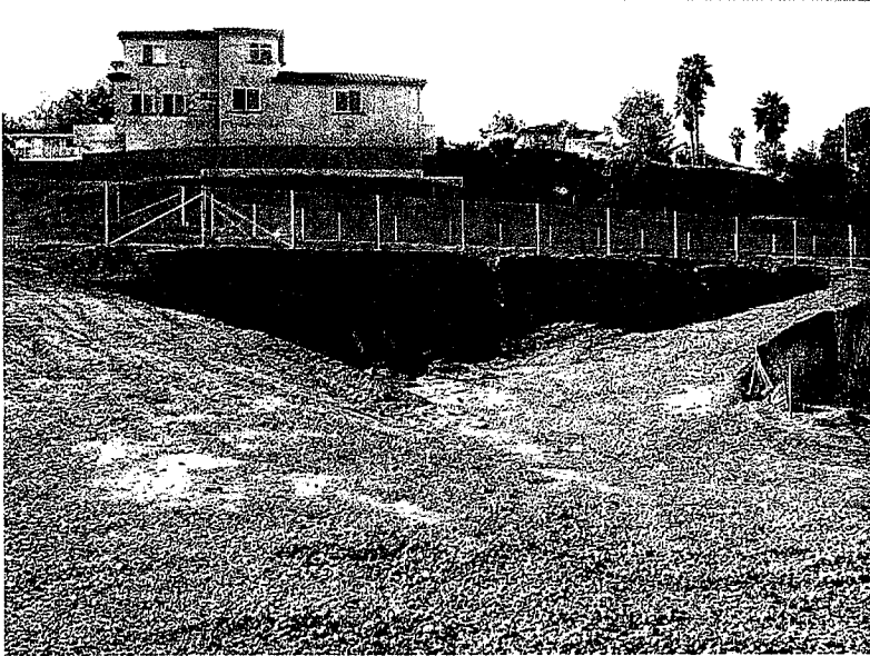
7. Another culvert that provides storm water run onto the construction storage yard is not redirected away from disturbed soils.
