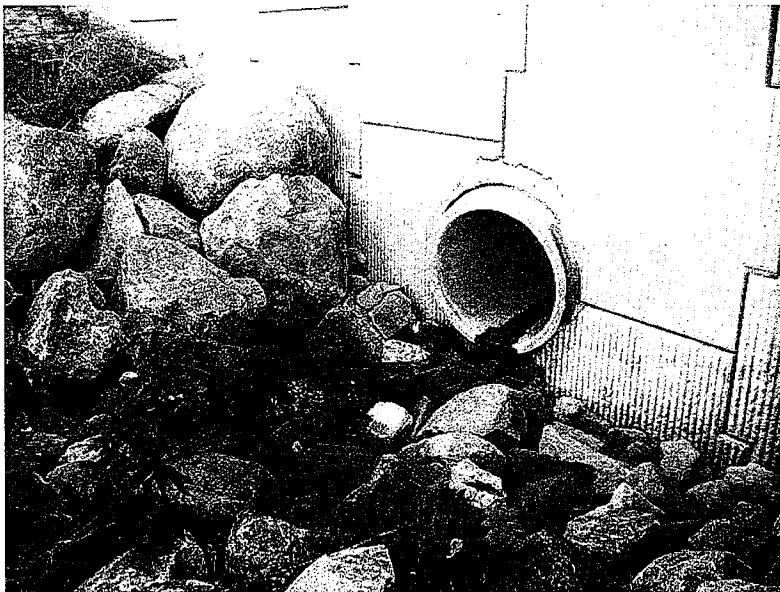
5. This culvert is the source of the run on coming through the storage yard.
