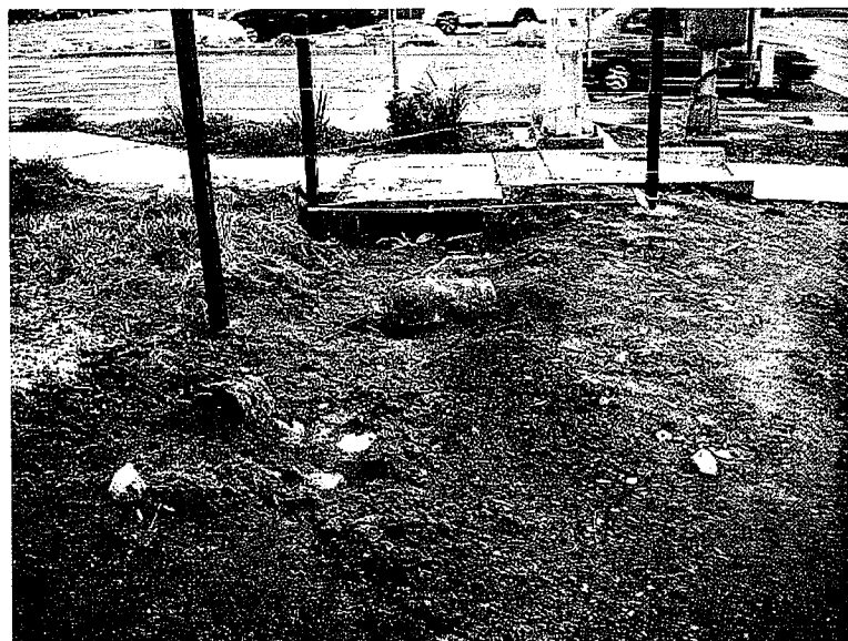
Photo 18 was taken at the Vista Transit Center.
