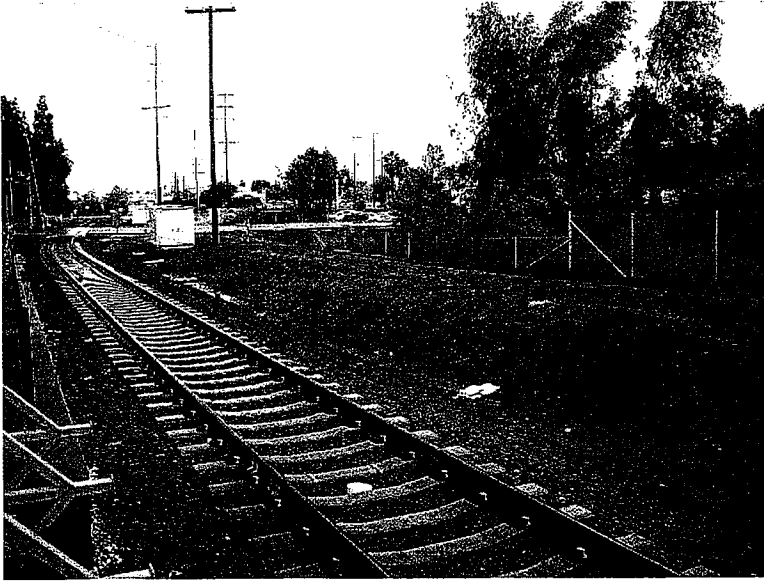
4. Slope lacks both erosion and sediment controls.
