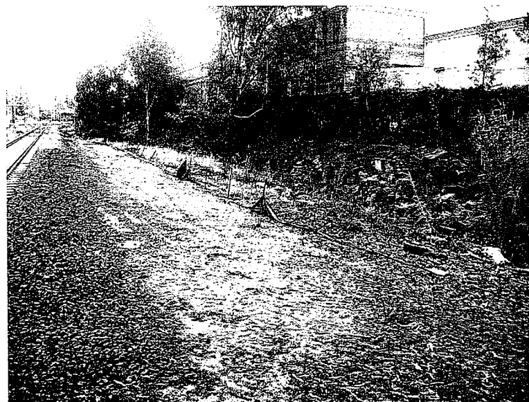
6. Silt fence in disrepair.
