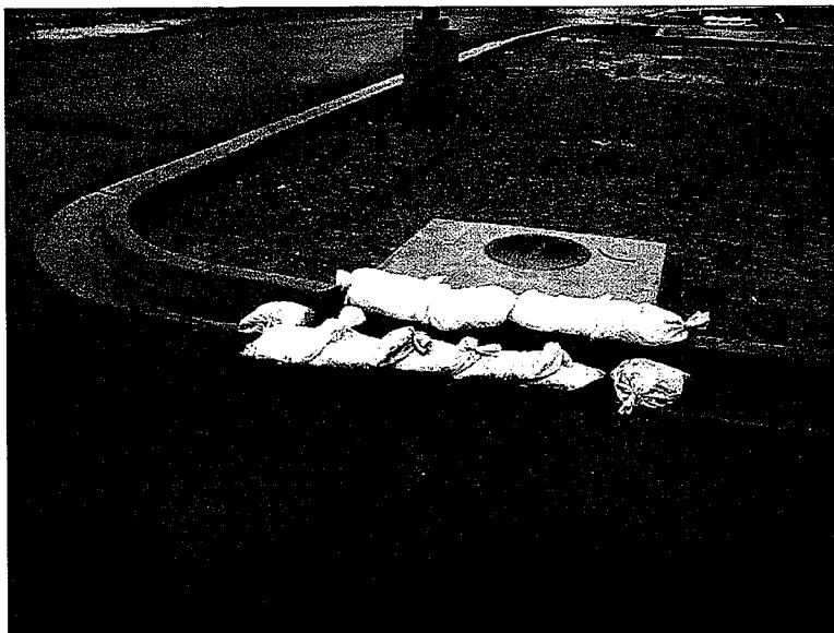
5. Gravel bags surrounding inlet in parking lot.
