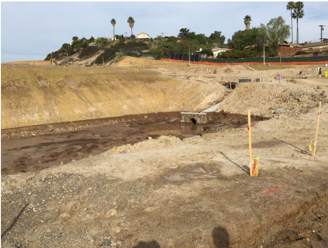
Figure 8. Failure to apply linear sediment controls. Photograph taken by Wayne Chiu, San Diego Water Board, on December 15, 2014, depicting the lack of linear sediment controls on a slope. IMG_5035.jpg
