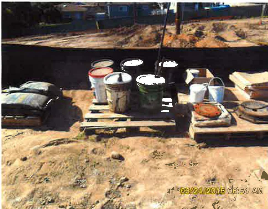
Figure 12. Failure to properly store chemicals. Photograph taken by the City of Lemon Grove on March 24, 2015, depicting chemicals and vehicle lubricants stored on pallets without protection from the elements and without secondary containment.
