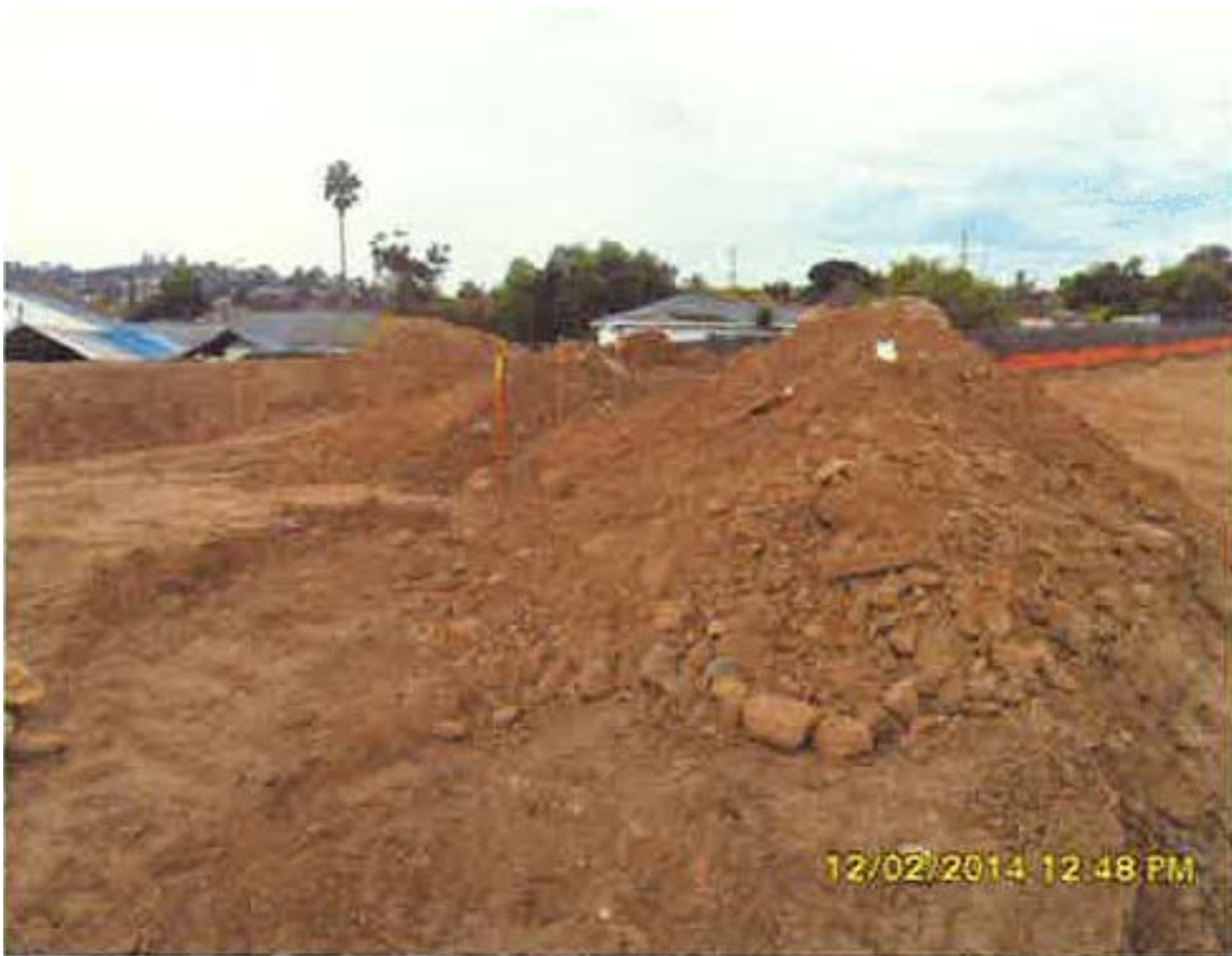
Figure 3. Failure to implement material stockpile BMPs. Photograph taken by the City of Lemon Grove on December 2, 2014.
